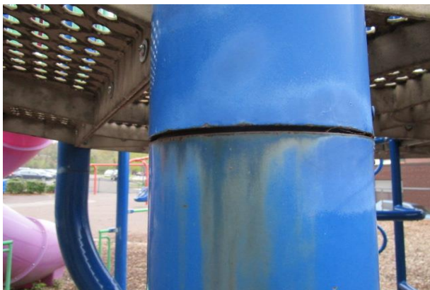
Structural Stability - Structure rusting & showing gaps at support post joints - MAINTENANCE
