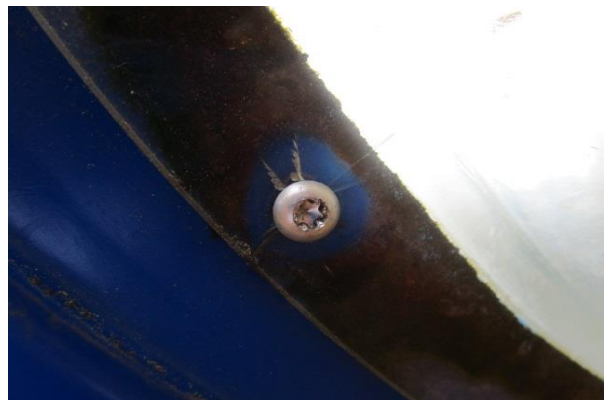
Look Down Panel - Loose at post bracket, bubble cracked at bolts - MAINTENANCE
