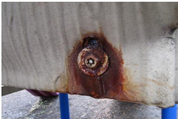
Stairs - One stair exposed holes in steel - CLASS B HAZARD
