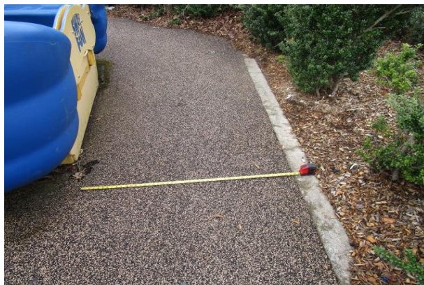
Sway Fun Glider - Use zone inadequate at 48" at rear - CLASS C HAZARD
