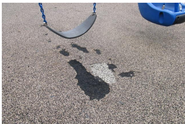
8ft. Swing Set - Surfacing has large holes - MAINTENANCE
