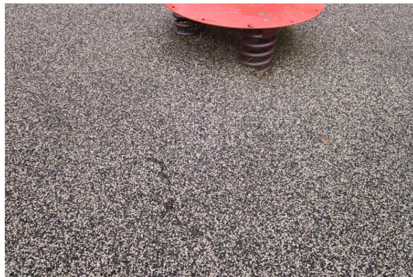
Surfacing - Small cracks in rubber - MAINTENANCE
