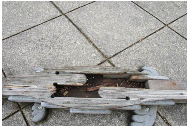
Alligator (SoundPlay) - Music component is missing - MAINTENANCE
