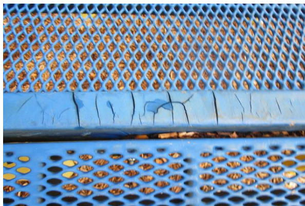
Decks (4) - One square 48" deck cracked at joints & very worn at Suspension Bridge, bolts pulling through steel - CLASS A HAZARD
