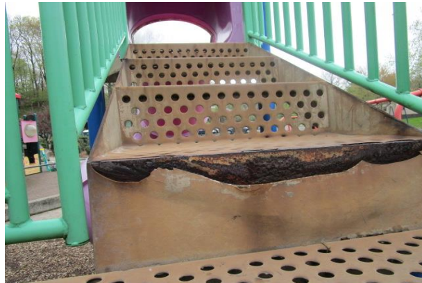
Stairs - One stair exposed holes in steel - CLASS B HAZARD
