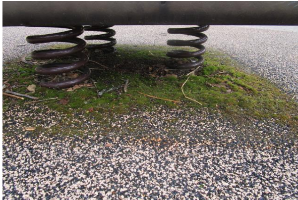
Bounce Saucer Pad - Top component missing - CLASS B HAZARD
