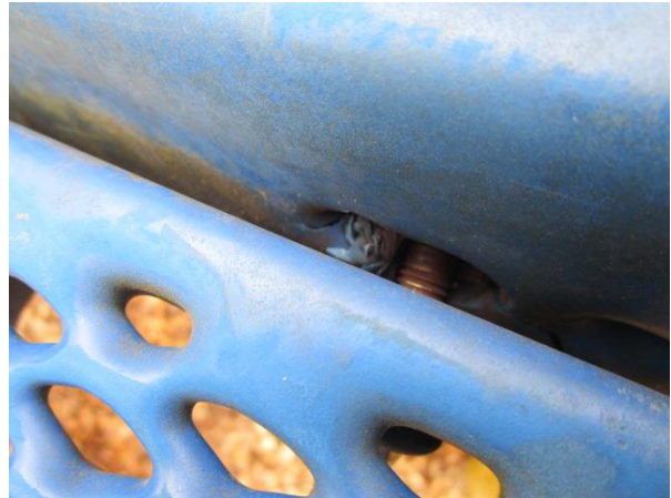
Look Down Panel - Loose at post bracket, bubble cracked at bolts - MAINTENANCE
