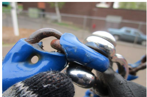
Freestanding Equipment 8ft. Swing Set (2Bays)(Landscape) - Chains worn at two belt seats - CLASS A HAZARD
