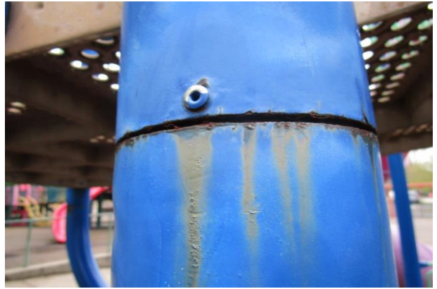
Structural Stability - Structure rusting & showing gaps at support post joints - MAINTENANCE
