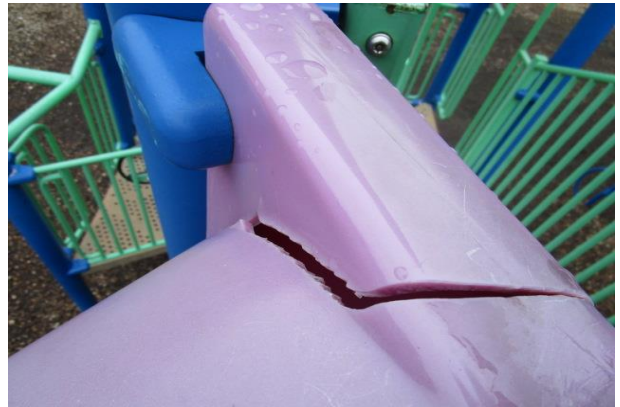
Wiggle Tube Slide - Cracked at top hood section - CLASS B HAZARD
