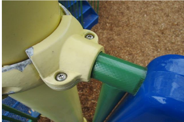
Transfer Platform - Step loose & plastisol worn - MAINTENANCE
