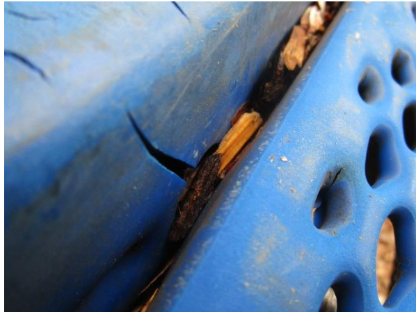
Look Down Panel - Loose at post bracket, bubble cracked at bolts - MAINTENANCE
