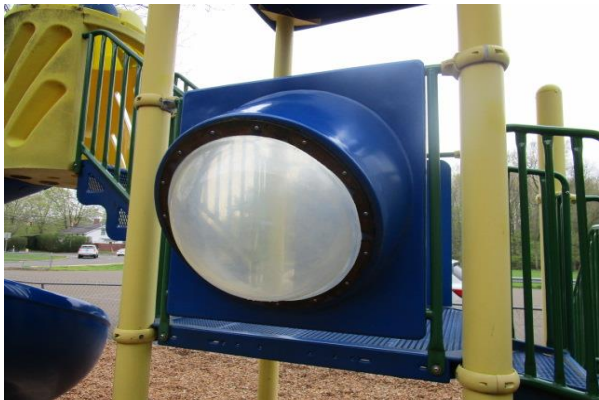
Look Down Panel - Loose at post bracket, bubble cracked at bolts - MAINTENANCE
