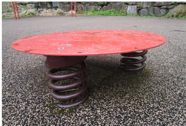
Bounce Saucer Pad - Top component missing - CLASS B HAZARD
