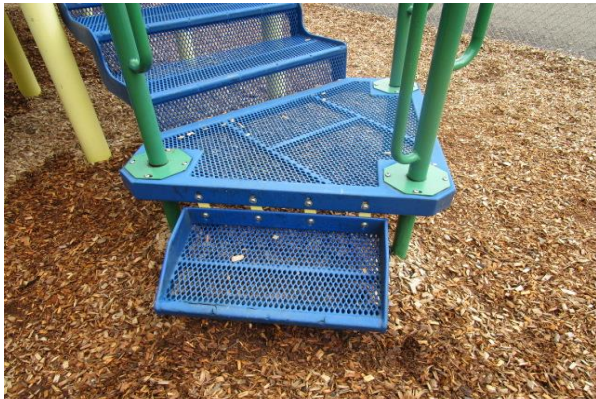
Transfer Platform - Step loose & plastisol worn - MAINTENANCE
