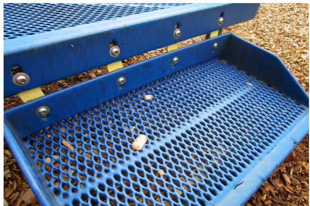
Transfer Platform - Step loose & plastisol worn - MAINTENANCE
