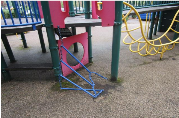
Wiggle Chain Ladder - Ladder & one handhold detached, chain worn - CLASS B HAZARD
