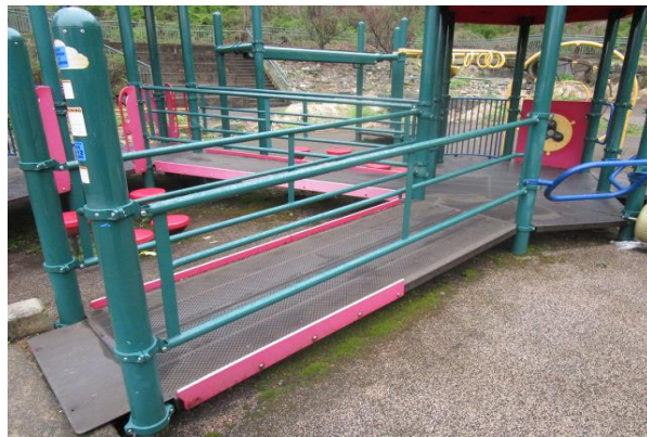
Entrance Ramp (2) - One section of 5" high rail missing - CLASS C HAZARD
