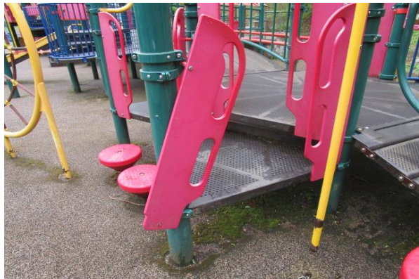
Disc Challenge - One handhold panel not attached - MAINTENANCE
