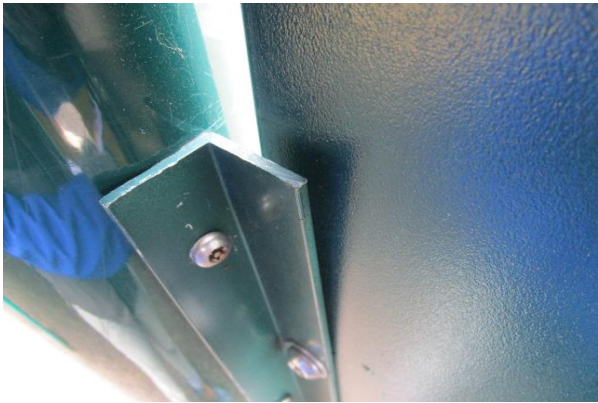
Rockwall (2) - Two protruding bolts - CLASS B HAZARD
