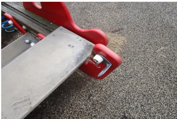
Multi-Spring See-Saw - One foot rest missing - MAINTENANCE
