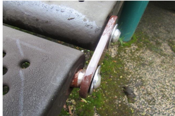
Suspension Bridge - One bolt out of one board - CLASS B HAZARD
