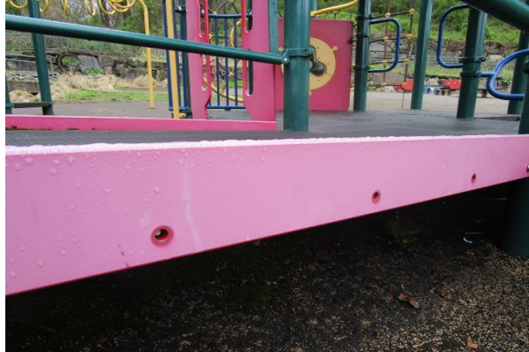
Disc Challenge - One handhold panel not attached - MAINTENANCE
