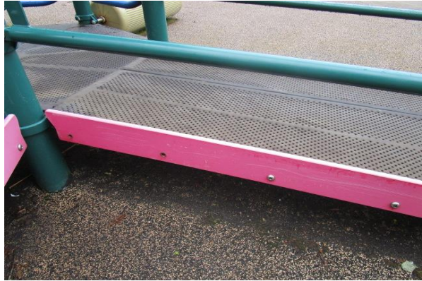
Entrance Ramp (2) - One section of 5" high rail missing - CLASS C HAZARD
