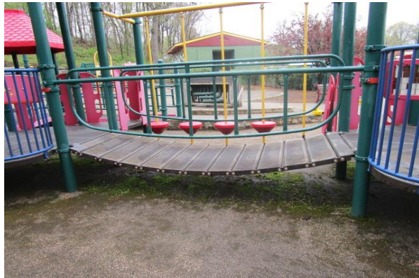
Suspension Bridge - One bolt out of one board - CLASS B HAZARD
