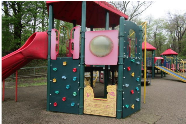
Vertical Rock Wall (2) - Non manufacturer parts, six broken bolt caps - MAINTENANCE
