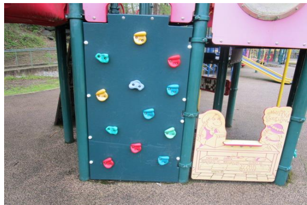
Vertical Rock Wall (2) - Non manufacturer parts, six broken bolt caps - MAINTENANCE
