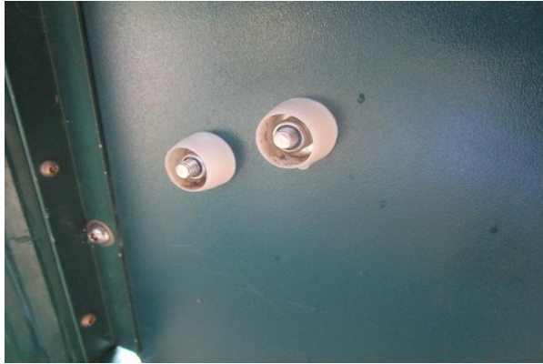
Rockwall (2) - Two protruding bolts - CLASS B HAZARD
