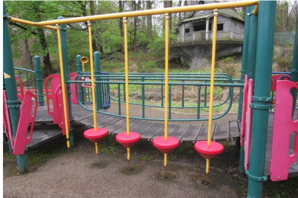
Disc Challenge - One handhold panel not attached - MAINTENANCE
