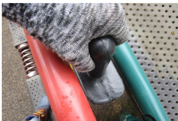
Spring Across Bridge - Head Entrapment between rail & Arch Bridge - CLASS A HAZARD
