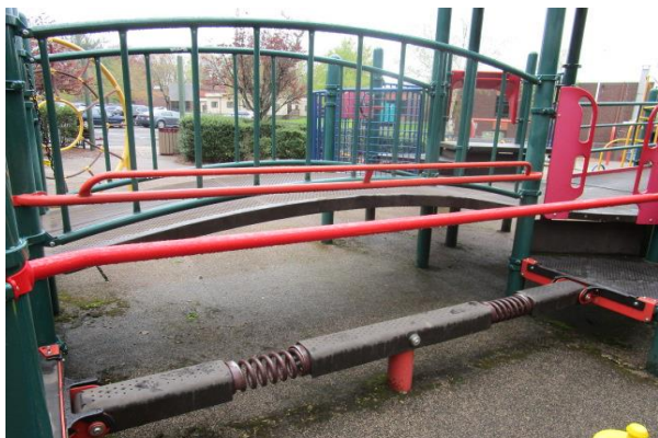
Spring Across Bridge - Head Entrapment between rail & Arch Bridge - CLASS A HAZARD
