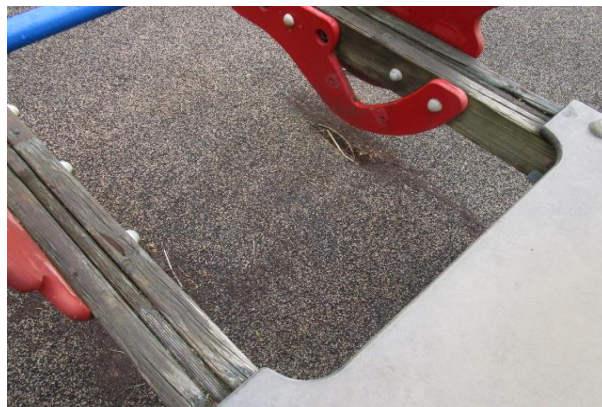
Multi-Spring See-Saw - One foot rest missing - MAINTENANCE
