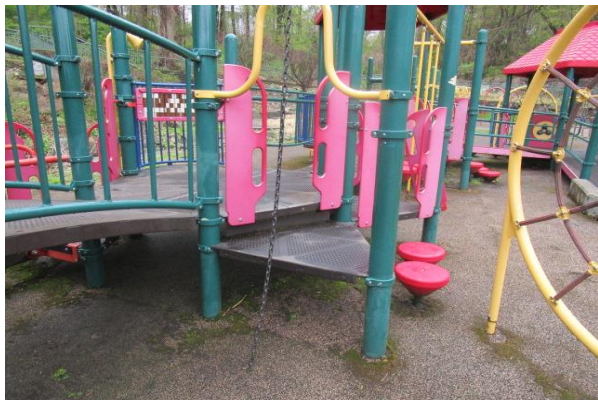
Ascending Chain - Cracked & worn - CLASS B HAZARD Barriers removed - CLASS B HAZARD
