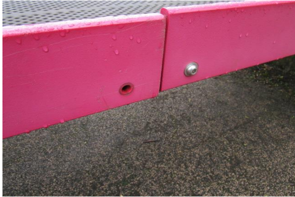
Entrance Ramp (2) - One section of 5" high rail missing - CLASS C HAZARD
