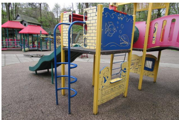
Curved Rung Ladder - Handhold panel cracked at bolts - MAINTENANCE
