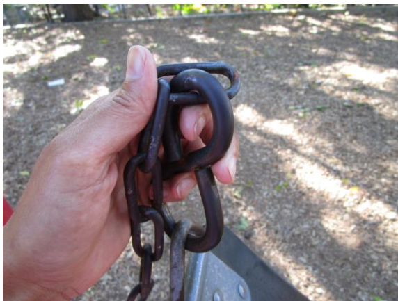
8ft. Swing Set - Eight clevises (below) & all chain starting to wear - MAINTENANCE
