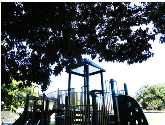
Use Zone - Overhanging branches touching composite - MAINTENANCE
