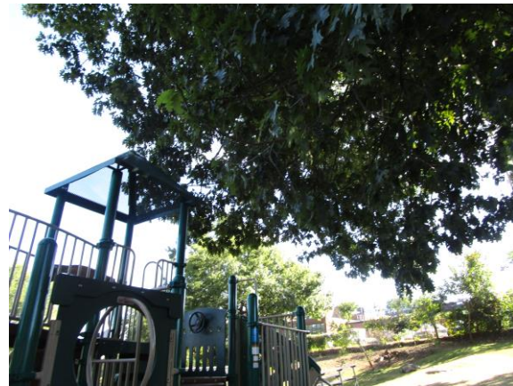
Use Zone - Overhanging branches touching composite - MAINTENANCE
