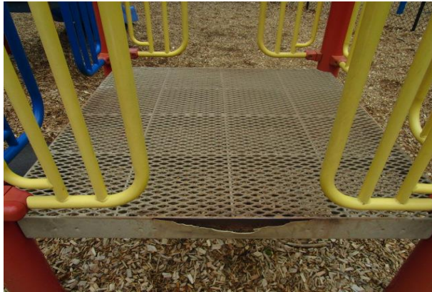
Decks (13) - Plastisol wearing at one deck - MAINTENANCE
