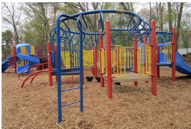
270° Overhead Loop Ladder - Missing one loop, four handholds loose at deck - CLASS B HAZARD
