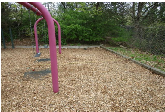
7ft. Swing Set (1Bay/2Belts)(GT) - Inadequate use zone at 13ft. In back - CLASS C HAZARD
