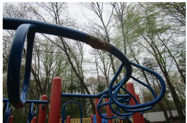
270° Overhead Loop Ladder - Missing one loop, four handholds loose at deck - CLASS B HAZARD
