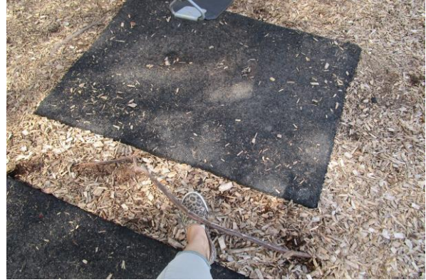
8ft. Swing Set (3Bay/6Belt/1Adapt.) - Felt exposed, tripping hazard - CLASS B HAZARD
