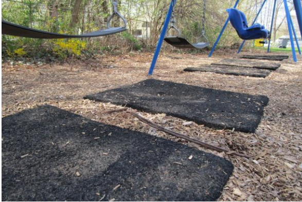
8ft. Swing Set (3Bay/6Belt/1Adapt.) - Felt exposed, tripping hazard - CLASS B HAZARD
