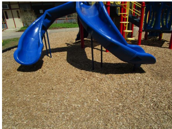
Surfacing - No wear mats at slide exits - CLASS C HAZARD
