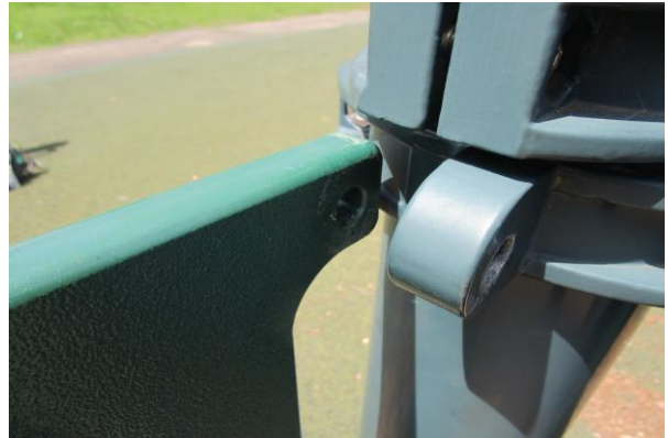
Tic-Tac-Toe Panel - Panel detached at one bolt - MAINTENANCE
