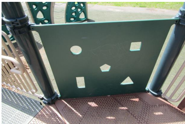
Geo Shapes Panel - Two bolts missing - MAINTENANCE
