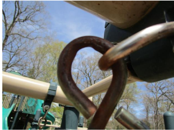
Double Trapeze Rings - Ten "S" - Hooks wearing - CLASS B HAZARD
