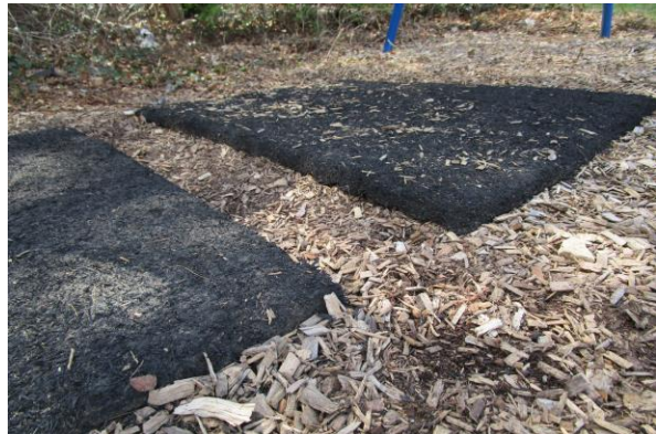
8ft. Swing Set (GameTime) - Wear mats not level, tripping hazard - CLASS B HAZARD
