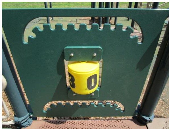
Racing Game Panel - Two levers missing - MAINTENANCE
