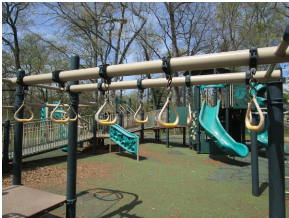
Double Trapeze Rings - Ten "S" - Hooks wearing - CLASS B HAZARD
