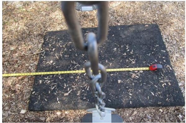
Use Zone - Inadequate at back due to brush 6ft. away - MAINTENANCE
