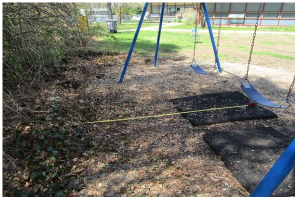
Use Zone - Inadequate at back due to brush 6ft. away - MAINTENANCE
