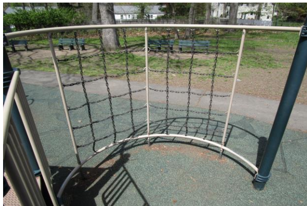
Radius Chain Net - Small cracks in plastisol - MAINTENANCE
