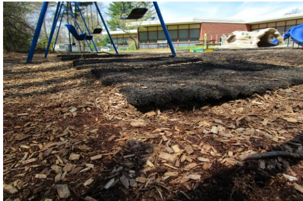
8ft. Swing Set (GameTime) - Wear mats not level, tripping hazard - CLASS B HAZARD
