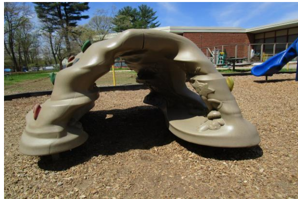
Crawl Thru Rock Climber (Play & Park) - One hand/foot hold cracked - MAINTENANCE
