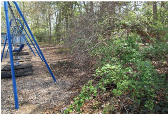
8ft. Swing Set - Brush encroaching in use zone - MAINTENANCE
