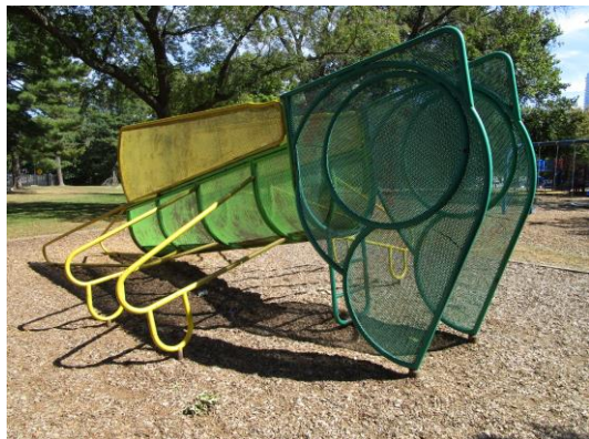
Grasshopper Climber (Unknown) - Pipe ladder split - CLASS B HAZARD
