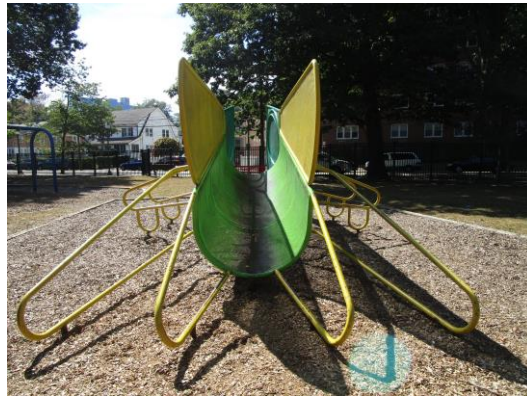
Grasshopper Climber (Unknown) - Pipe ladder split - CLASS B HAZARD
