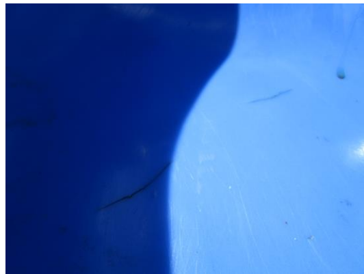
360° Spiral Slide - Two cracks in bed way - CLASS B HAZARD
