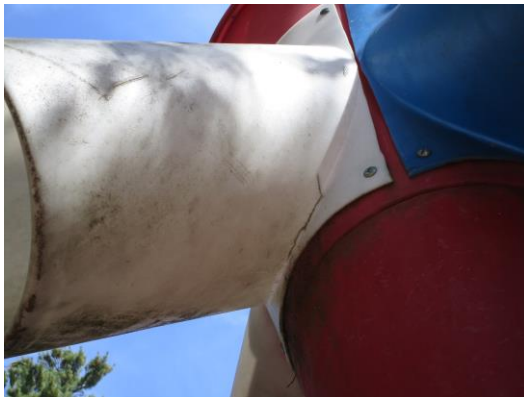
Grasshopper Climber (Unknown) - Pipe ladder split - CLASS B HAZARD
