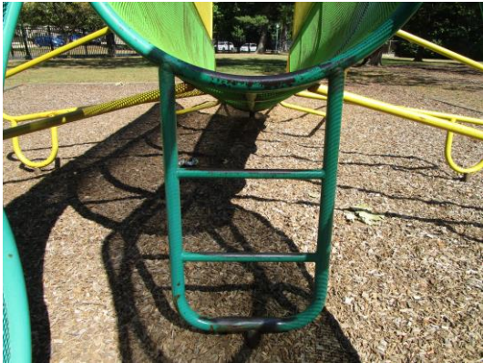
Grasshopper Climber (Unknown) - Anchors exposed - CLASS B HAZARD
