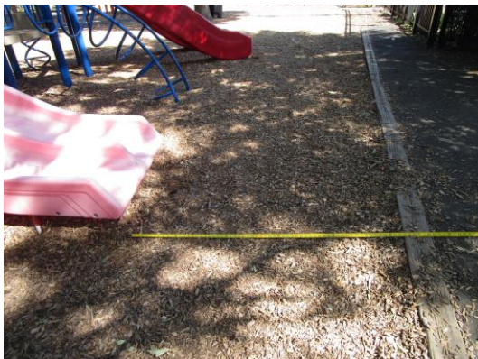
Use Zones - Inadequate, only 63" at Rumble Slide - CLASS C HAZARD
