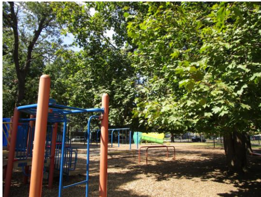
Use Zone - Overhanging branches too close to Overhead Ladder - MAINTENANCE
