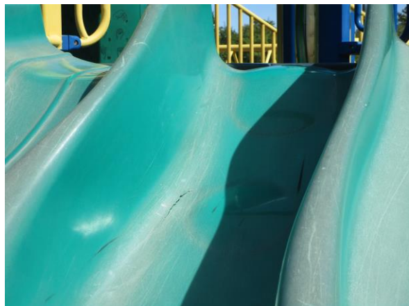
Big Foot Slide - Large crack in center of bed way - MAINTENANCE
