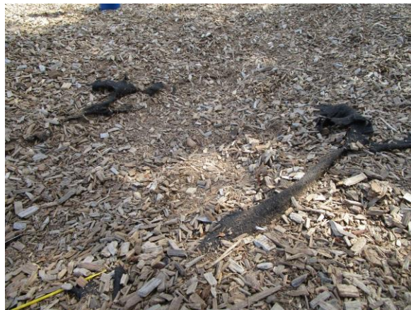
Surfacing - Exposed fabric, tripping hazard - CLASS B HAZARD
