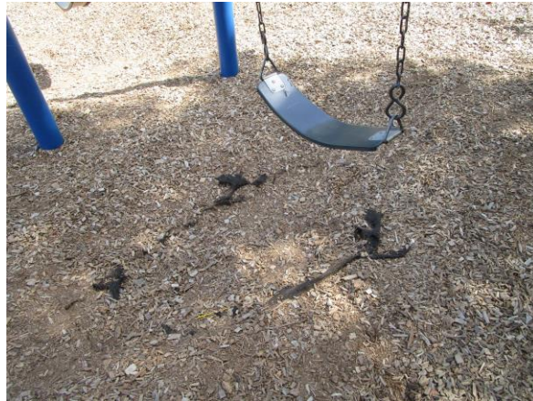
Surfacing - Exposed fabric, tripping hazard - CLASS B HAZARD
