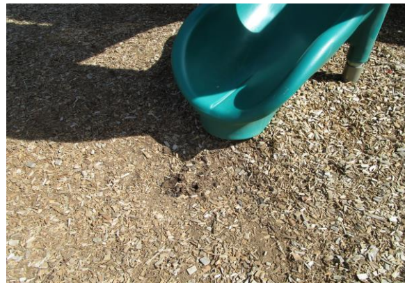
Surfacing - No wear mat at Spiral Slide exit - CLASS C HAZARD
