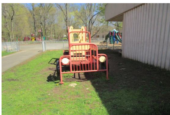
Use Zone - Inadequate, no clear use zone - CLASS A HAZARD
