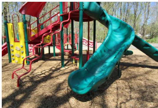
Triple Avalanche Slide - One slide loose at bottom footing - MAINTENANCE
