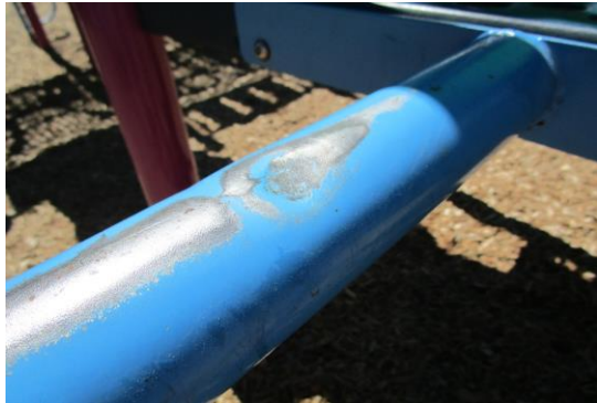
Tunnel Up Crawl Tube - Large cracks at top of one section - CLASS B HAZARD
