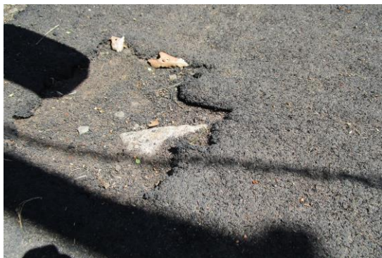
Surfacing - Fabric exposed, tripping hazard - CLASS B HAZARD
