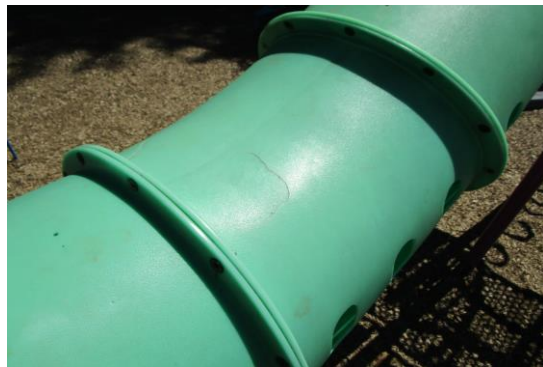
Tunnel Up Crawl Tube - Large cracks at top of one section - CLASS B HAZARD
