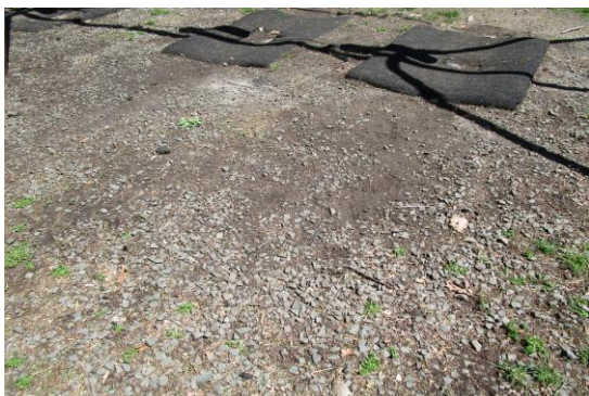
Surfacing - None, gravel & rocks below swings- CLASS A HAZARD
