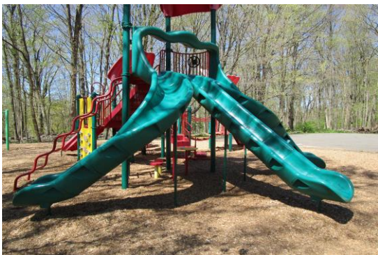
Triple Avalanche Slide - One slide loose at bottom footing - MAINTENANCE
