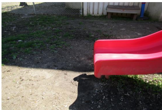
Surfacing - No wear mat at slide exit - CLASS C HAZARD
