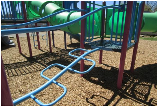
Tree Climber Link - Dent in pipe - MAINTENANCE
