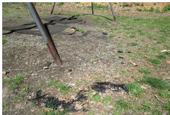
Surfacing - Fabric exposed, tripping hazard - CLASS B HAZARD
