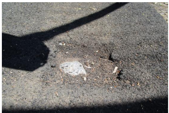
Surfacing - None, gravel & rocks below swings- CLASS A HAZARD
