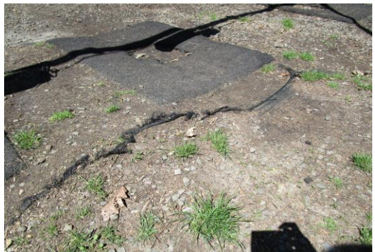
Surfacing - Fabric exposed, tripping hazard - CLASS B HAZARD
