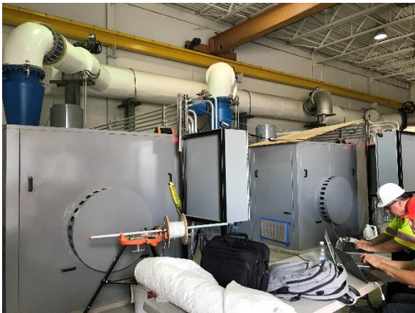
New blowers and sound attenuators
