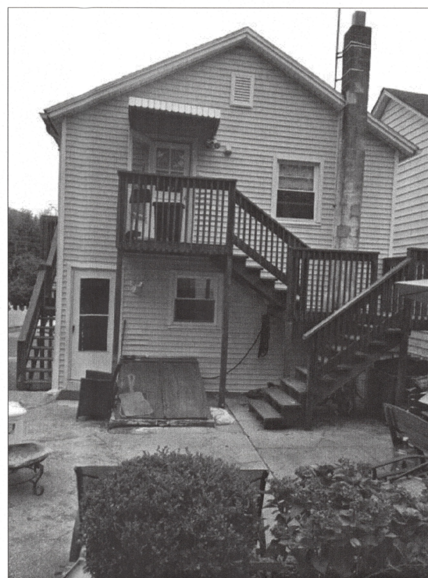
Rear View (WEST ELEVATION)
