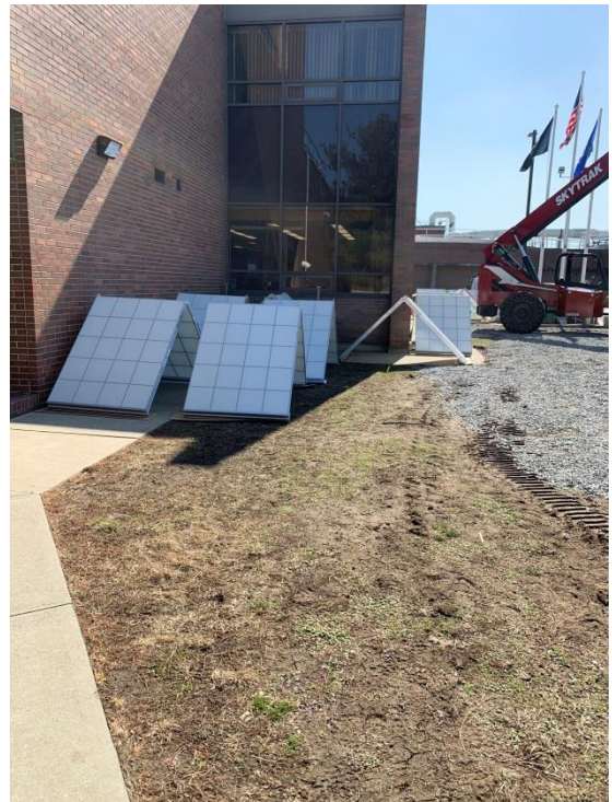
Canopy sections for over the new UV system
