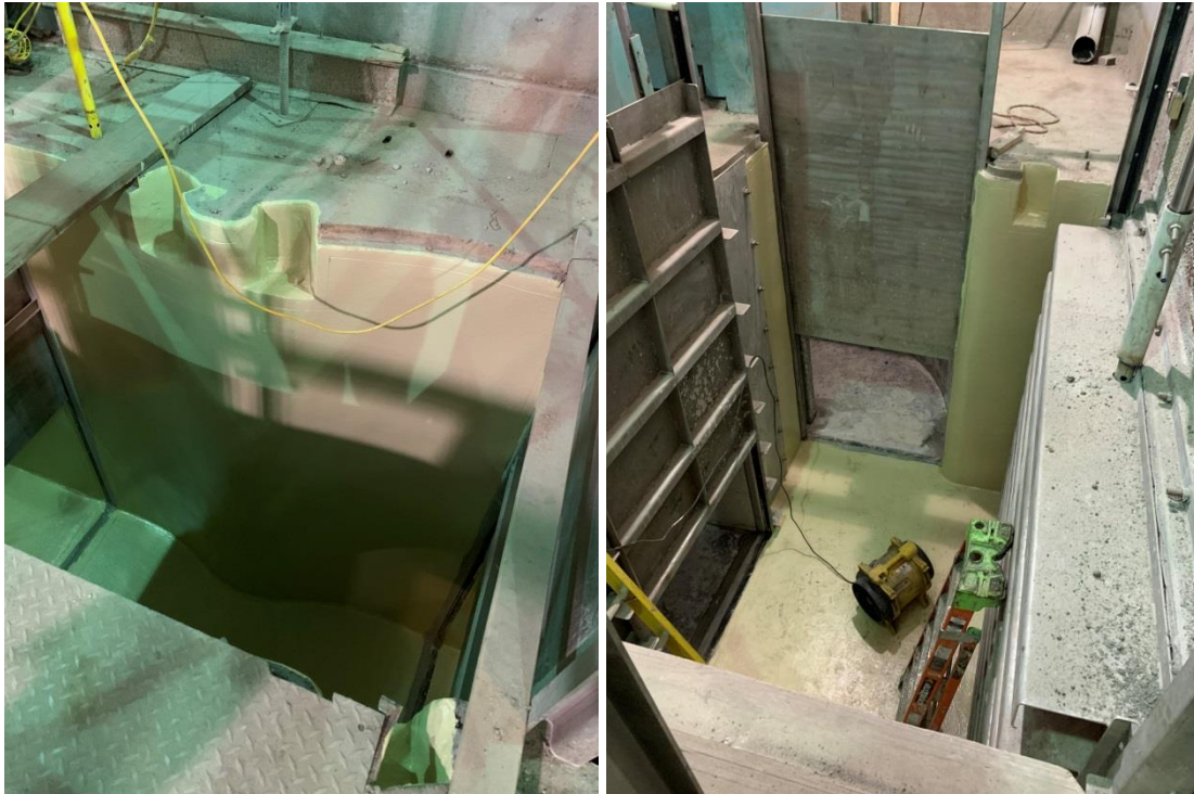
Coating of channels
