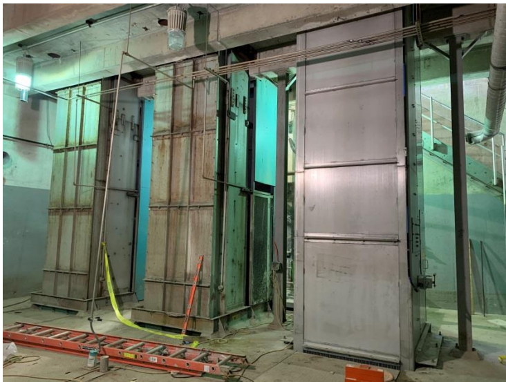
New Bar Screen in Channel 3
