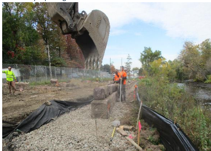
Figure 16 - Repurposing Excavated Brownstone at the Mill River Greenway
