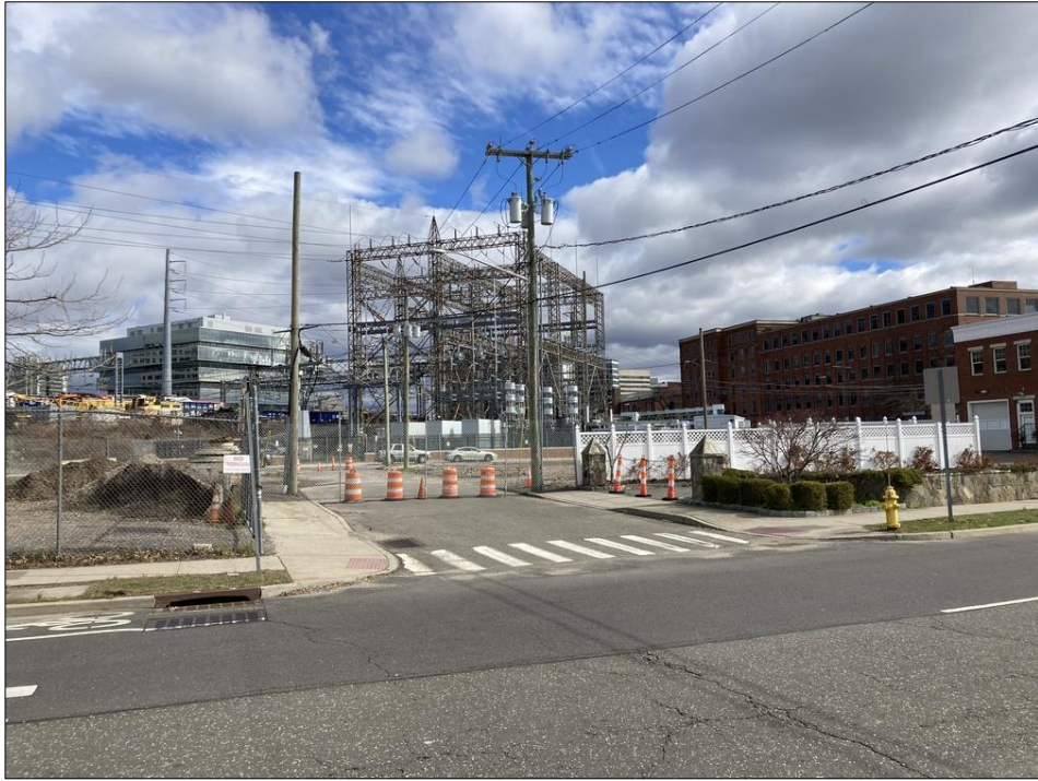
Site view from Dock Street
