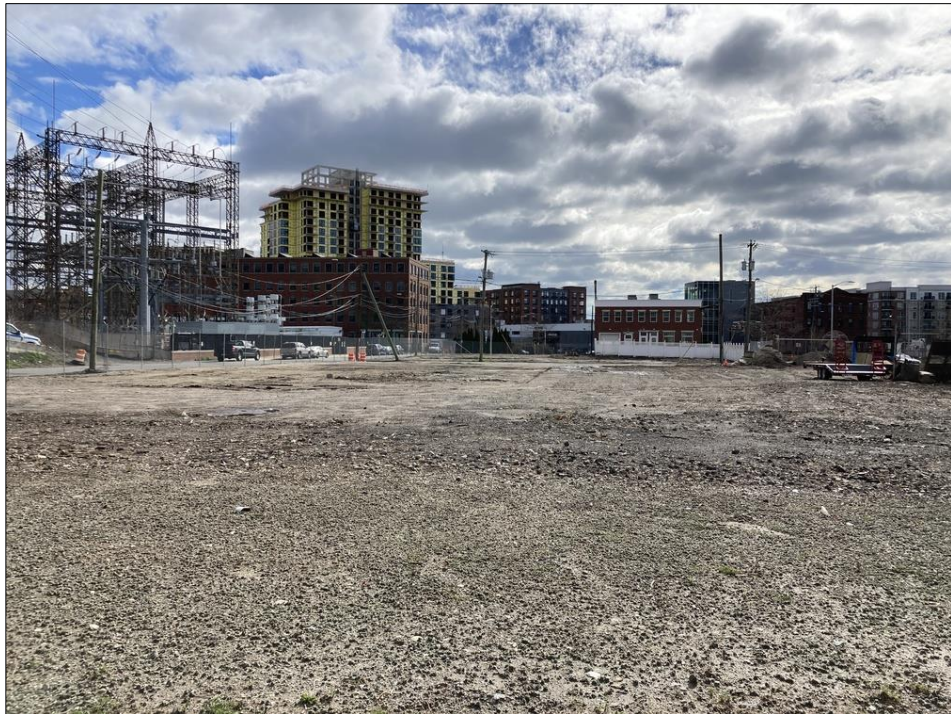
Abutting land - west block
