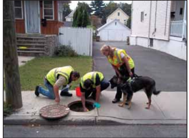
Photo 2. ECS and City employees inspect a stormwater manhole on Orange Street.
