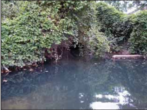
Photo 1. Outfall DIS 50. A bucket of water from this pool tested positive for sewage.
