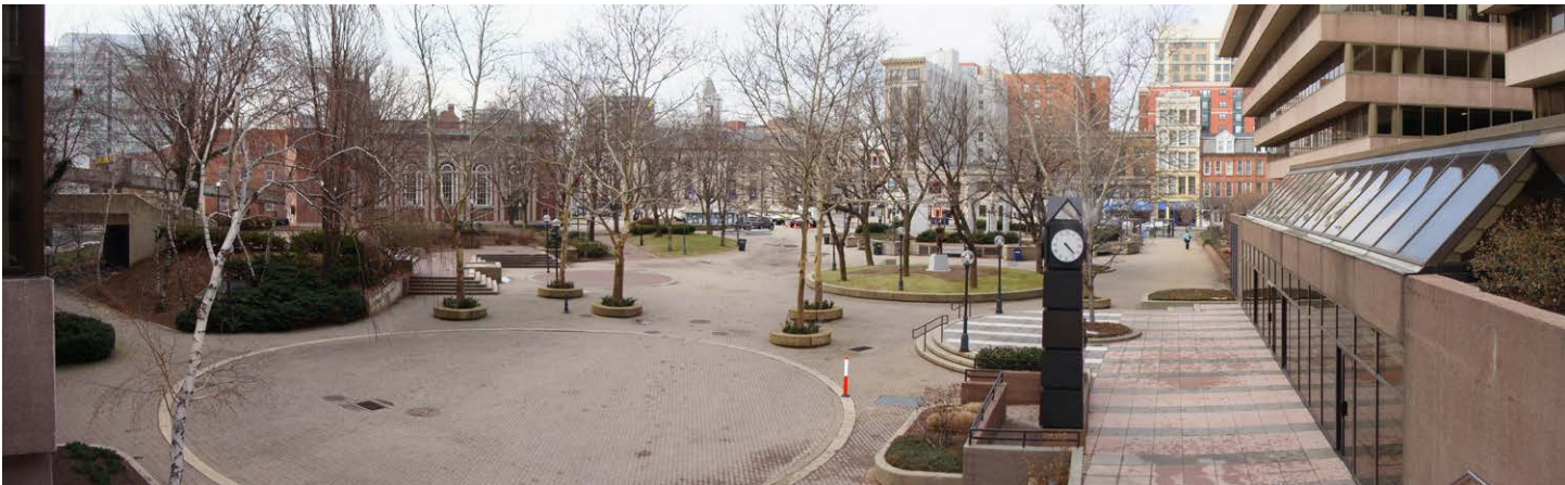
Existing Condition Photos
