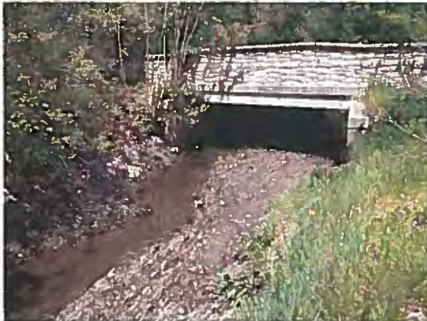
View of sampling location – looking downstream from bridge.
