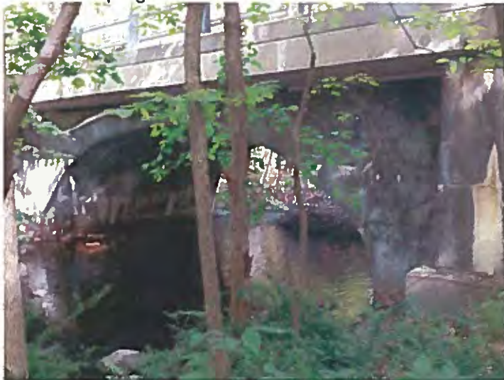
View of sampling location.
