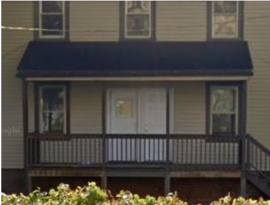
Existing front doors
