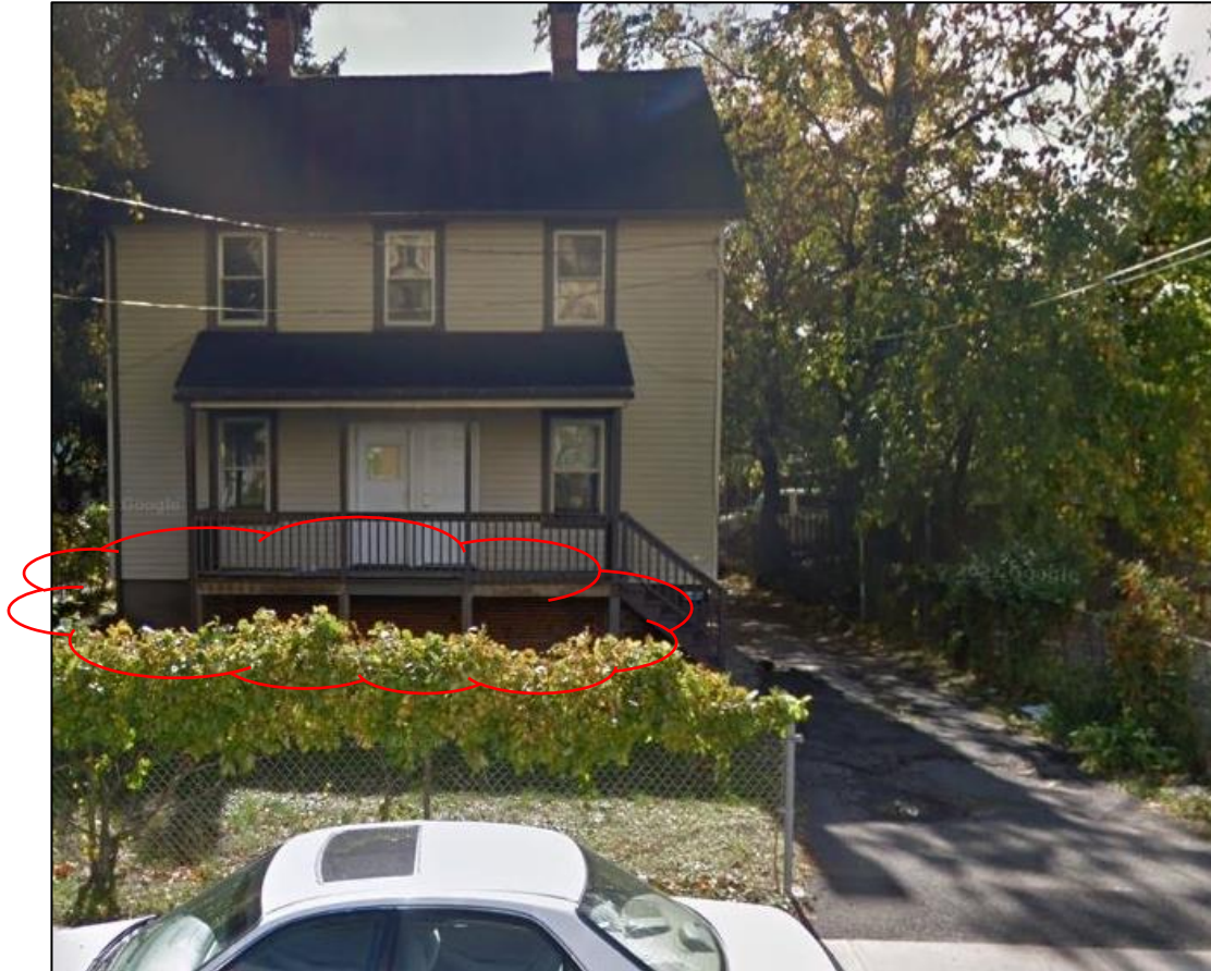
Existing porch (present day)
