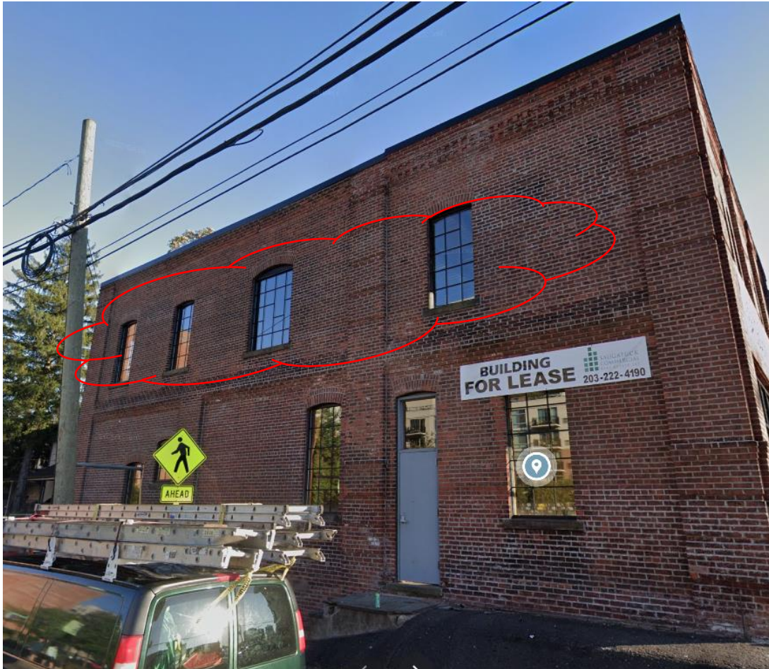
Existing Building (Henry Street frontage)
