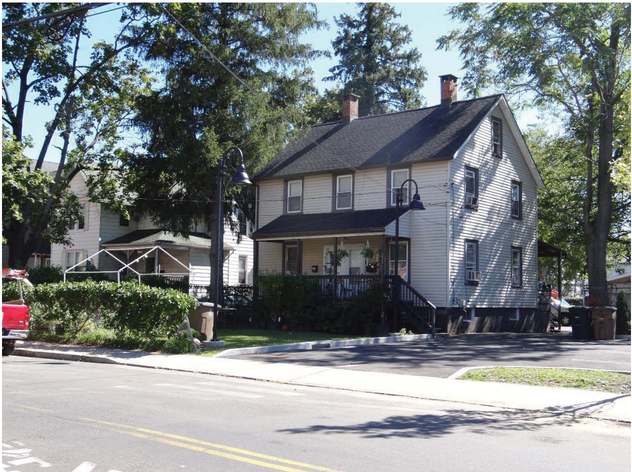
Cottage at 171 Henry Street
