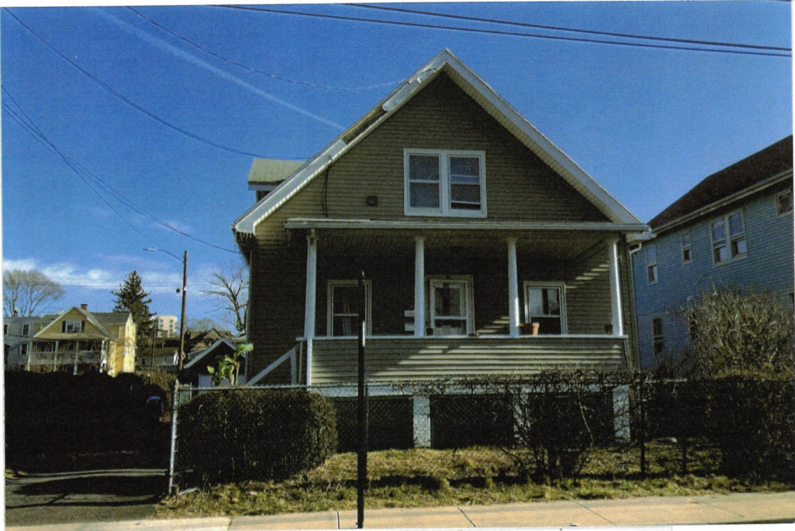
Photograph 1 Facade (South Elevation)
