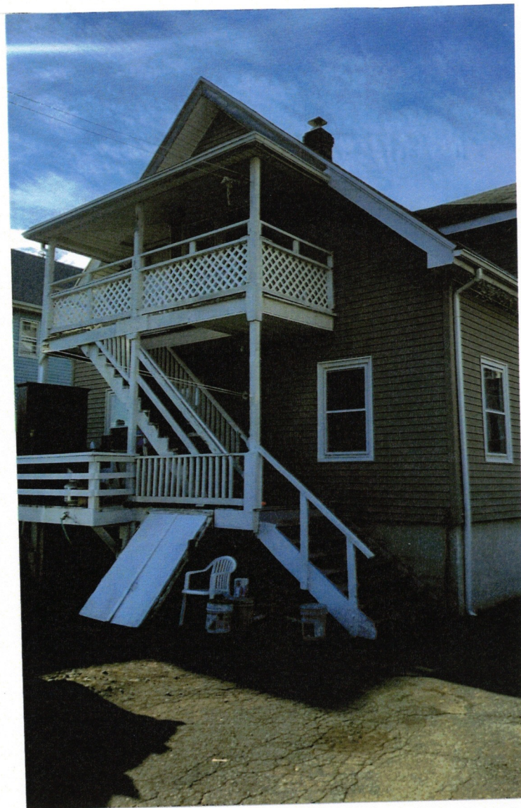
Photograph 8, Rear (North) Elevation
