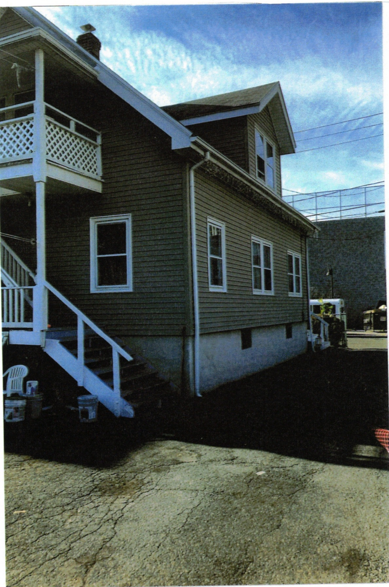
Photograph 7, West Elevation & Rear (North) Elevation (to the left)
