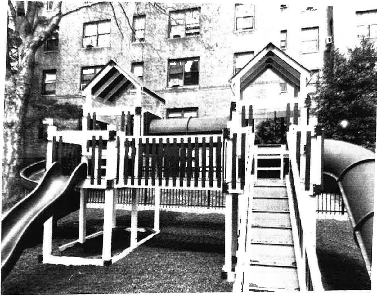
Inspected: 2-12 homemade, composite play set with shredded rubber as surfacing
