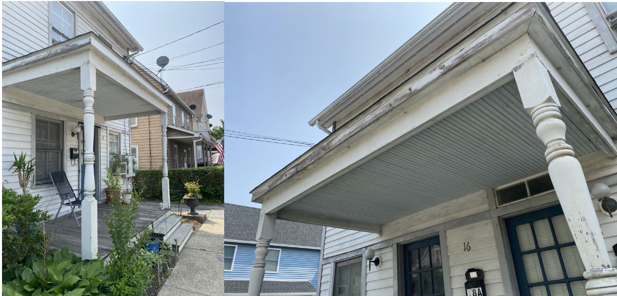
Fig. 4 (left) and Fig. 5 (right) in situ veranda posts and beadboard on the porches of 18 Taylor Street. Period-appropriate colors and finishes will be used in the restoration of the building's original porches.
