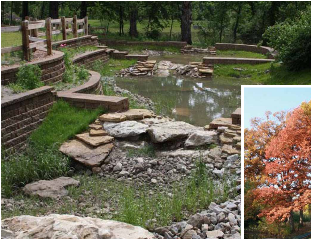
Stormwater from the school driveway and parking lot passes through the three cells of the bioretention system (above) en route to the receiving pond (right).
