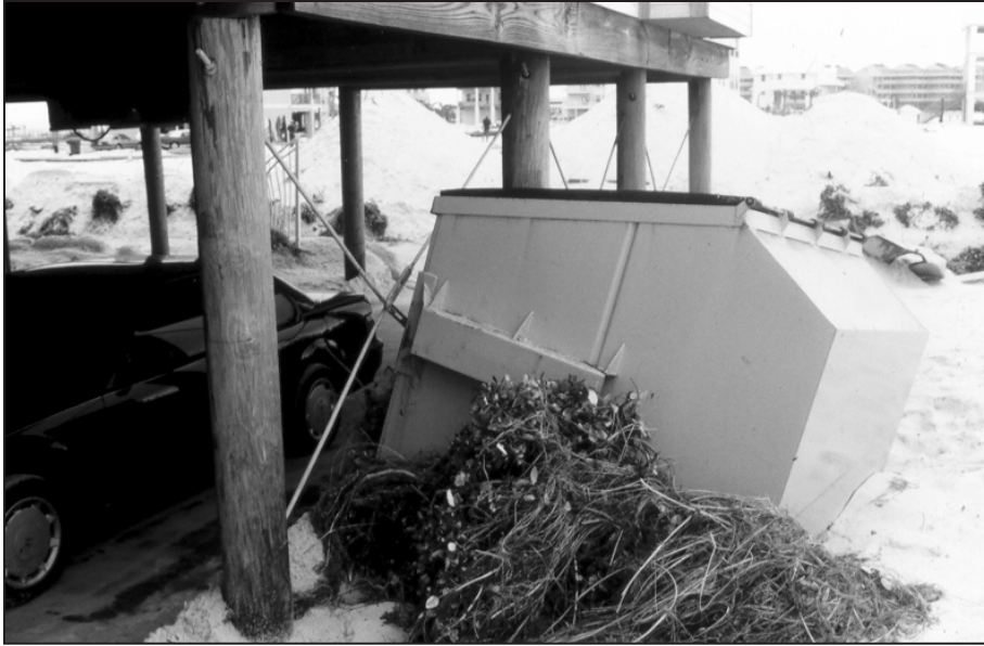
Figure 7. Trapping of floating debris by metal rod cross-bracing
