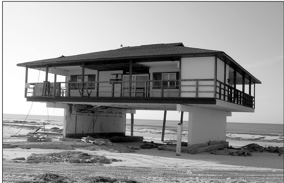
Figure 9. House elevated on shore-perpendicular shear walls. This design approach is risky for low-rise buildings since lateral out-of-plane loads (wind and flood acting on the faces of the shear walls) can be large and special design considerations and detailing are required.
