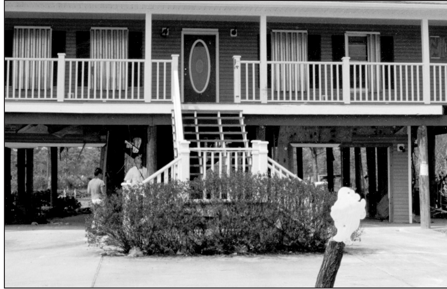
Figure 2. Example of open stairs that minimize transfer of flood and wave forces (note that building codes enforced by most communities require use of risers that prevent passage of a 4-inch sphere).
