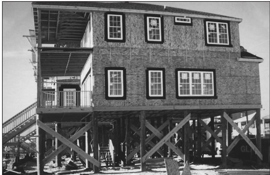
Figure 6. Elevated coastal home with timber cross-bracing, principally in the shore-perpendicular direction
