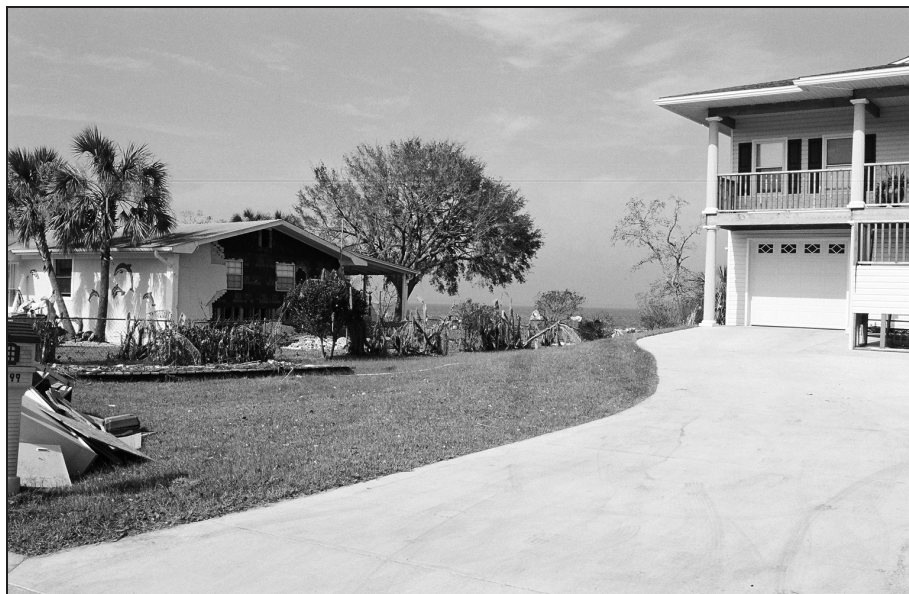
Figure 17. Post-hurricane photo showing elevated building surrounded by gently sloping fill, with adjacent damaged pre-FIRM building (the presence and configuration of the fill were judged by the damage inspection team not to have led to flood or wave damage to the elevated building or the nearby pre-FIRM building).
