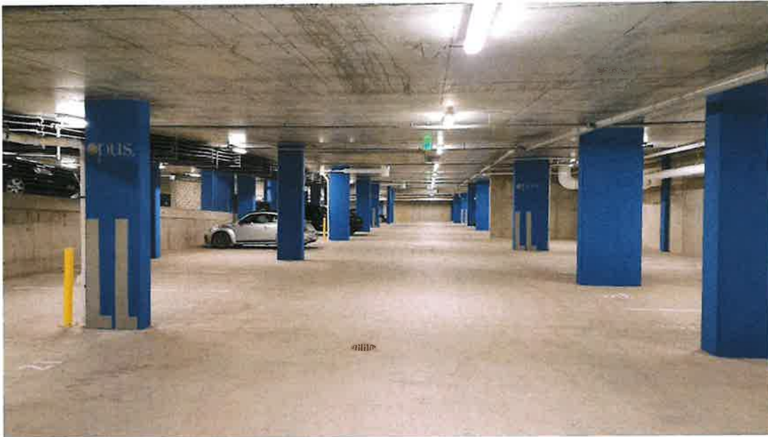
Figure 5- Basement Level of Garage in Good Condition
