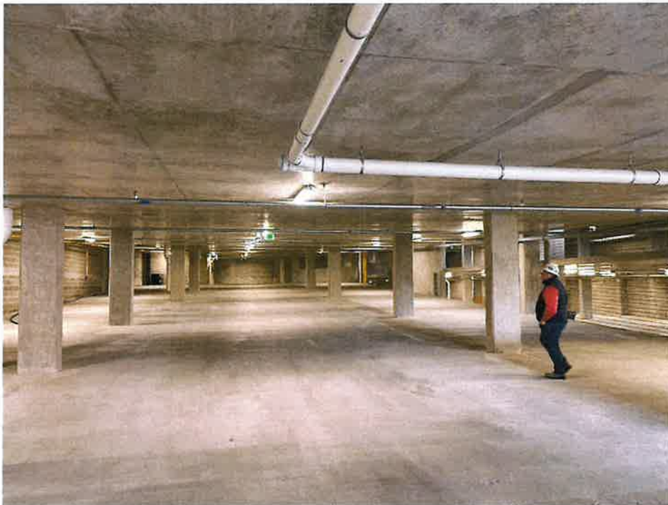
Figure 12- 2 nd Floor of Parking Garage
