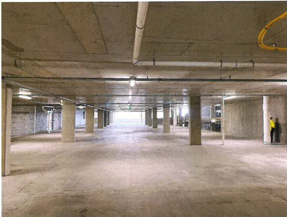
Figure 14- 3 rd Floor of Parking Garage
