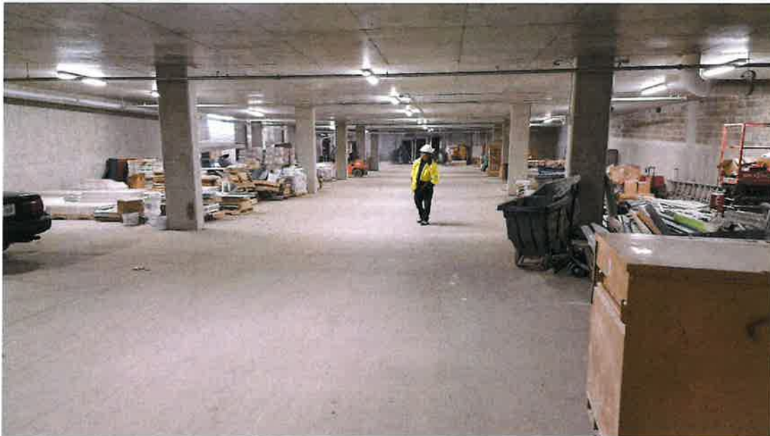
Figure 6- 1st Level of Parking Garage
