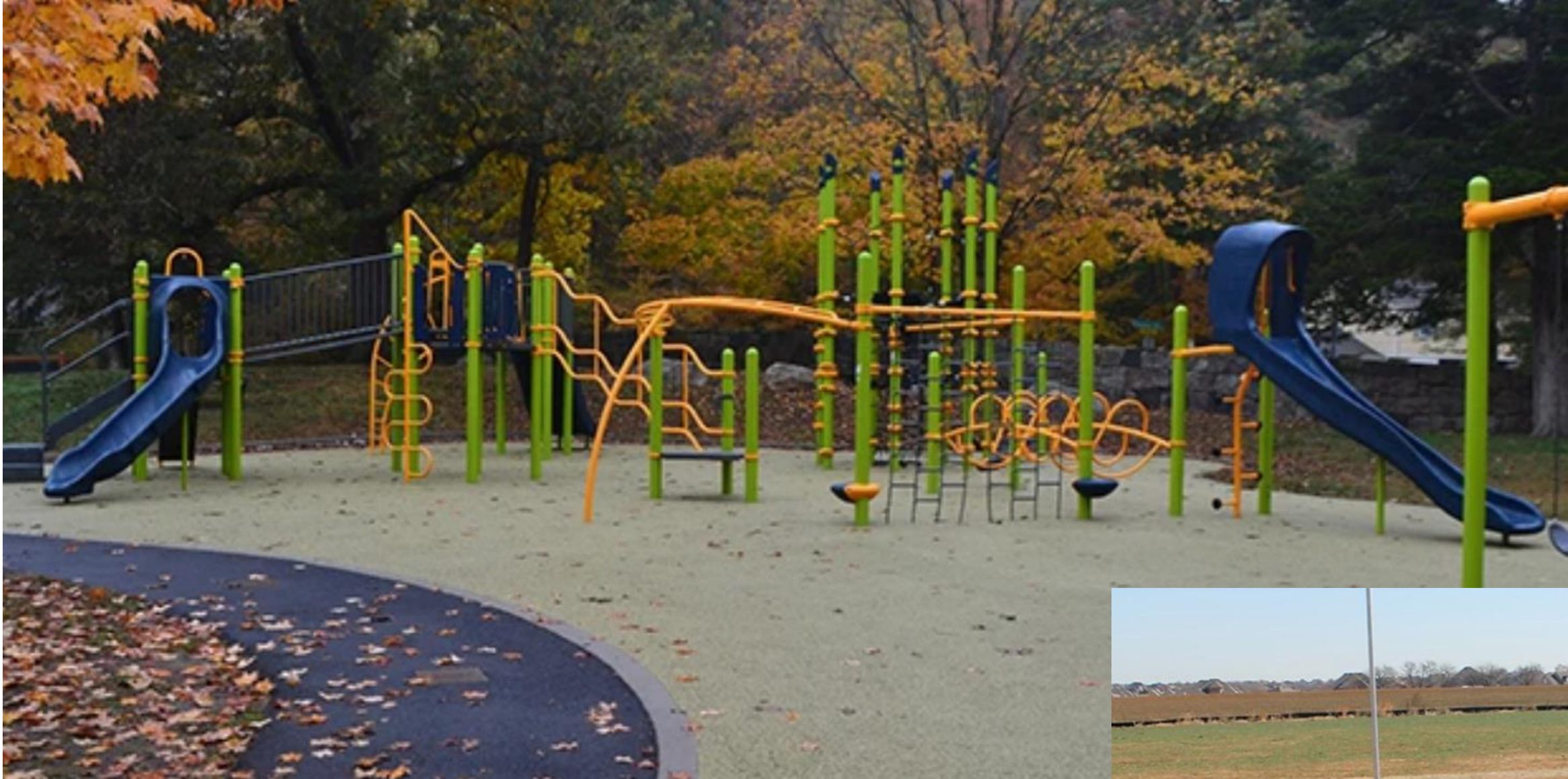
Poured in Place Rubber (PIP)
