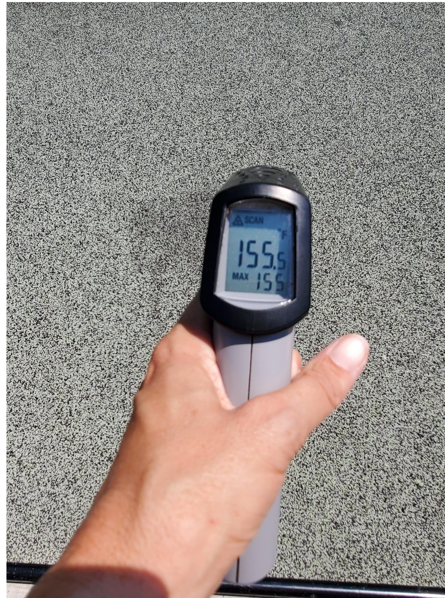
Poured in Place Rubber (PIP)
