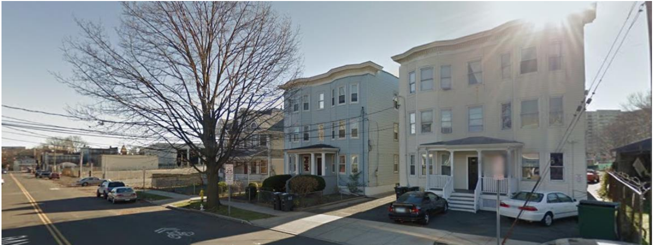
Multi-family residences looking east on Woodland Avenue
