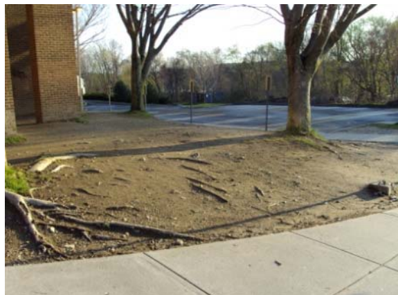
Photo #30: Barren landscaping at front of building
