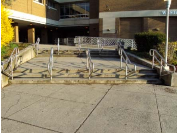
Photo #19: Concrete steps at front of building
