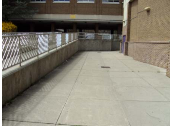
Photo #32: Concrete retaining wall and sidewalk at front of building
