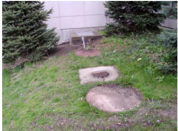
Photo #82: Underground 6,000-gallon fuel oil storage tank adjacent New AgriScience
