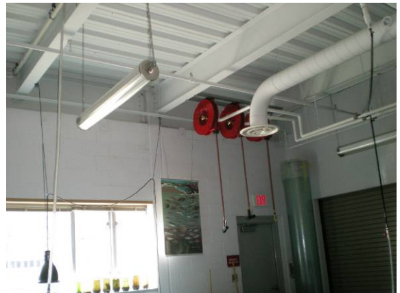
Photo #250: Structure of new AgriScience Building
