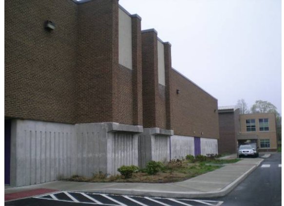
Photo #170: Elevation of old gym facing football field
