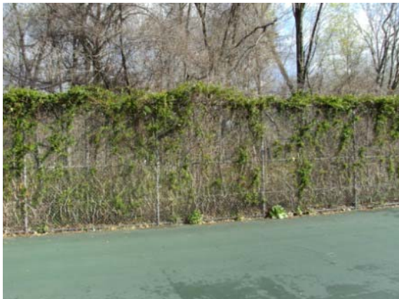
Photo #41: Chain link tennis court fencing
