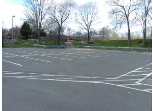
Photo #8: Parking lot at rear of building (north elevation)
