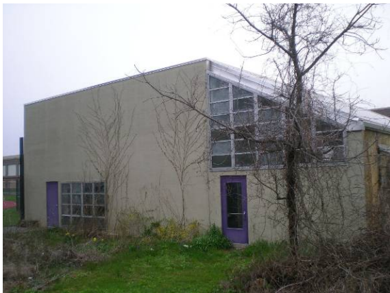
Photo #263: Old AgriScience Building – west elevation
