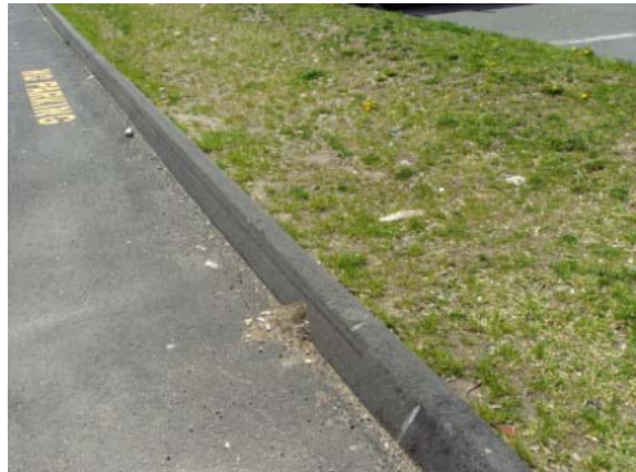
Photo #22: Asphalt curbing
