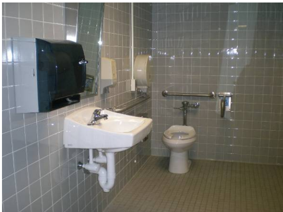
Photo #203: ADA restroom - ground floor level near auditorium and music classrooms
