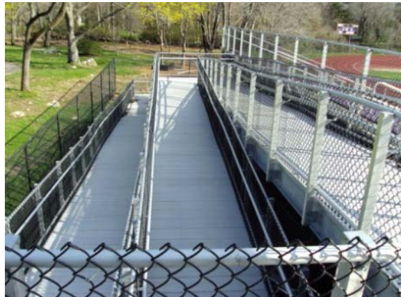
Photo #46: ADA ramp at football field bleachers leading to press box
