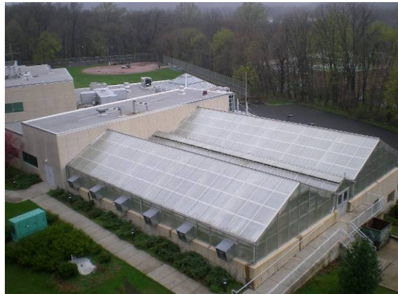
Photo #246: Roof overview – new AgriScience Building
