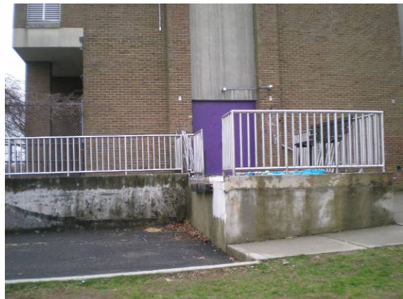
Photo #222: Loading dock at Auditorium
