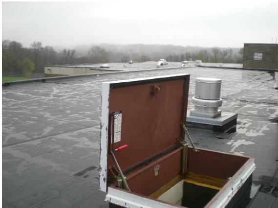
Photo #191: Roof hatch
