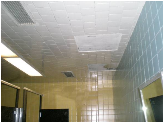
Photo #213: Finishes in students' restroom in Finch (A) Wing
