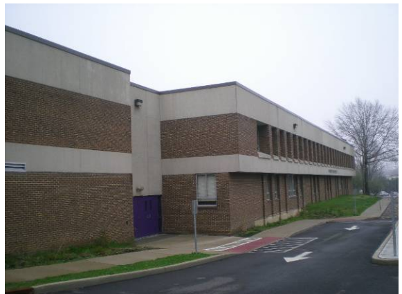
Photo #168: Street/south facing elevation
