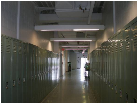
Photo #249: Corridor of new AgriScience Building
