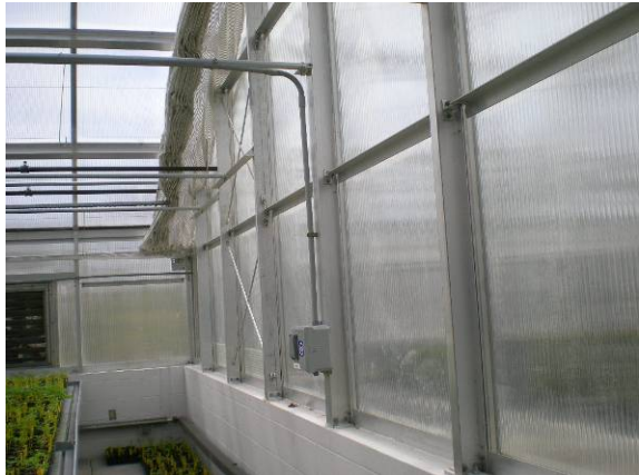
Photo #256: Structure of acrylic panel walls
