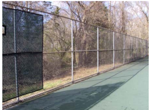
Photo #42: Chain link tennis court fencing
