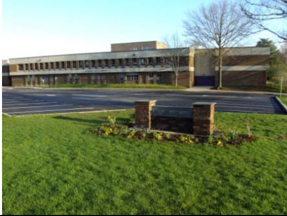
Photo #1: Property identification signage at front elevation of building
