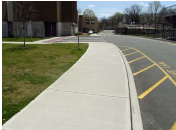
Photo #16: Concrete sidewalk and curbing at west elevation of building
