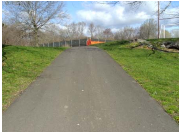
Photo #18: Asphalt sidewalk leading to practice soccer field and tennis courts
