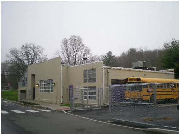
Photo #261: Old AgriScience Building – east and north elevations
