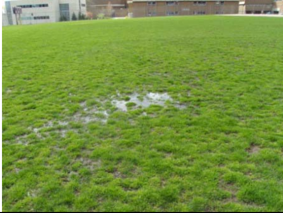
Photo #61: Baseball field ponding
