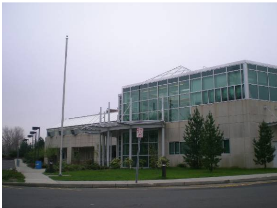
Photo #239: New AgriScience Building – east elevation
