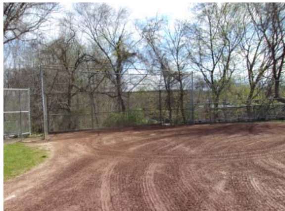
Photo #58: Softball field chain link fence backstop
