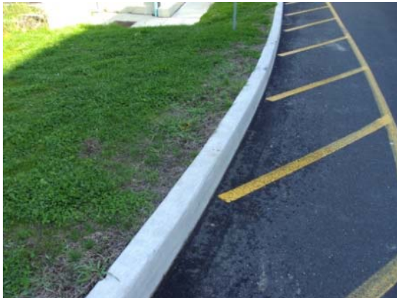
Photo #21: Concrete curbing
