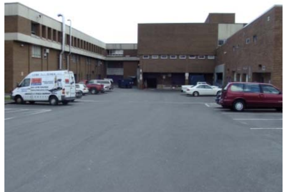
Photo #10: Service drive at rear of building
