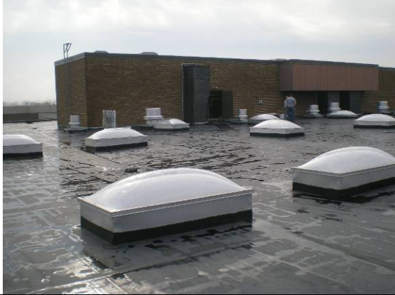
Photo #193: Partial overview of skylights and roofing
