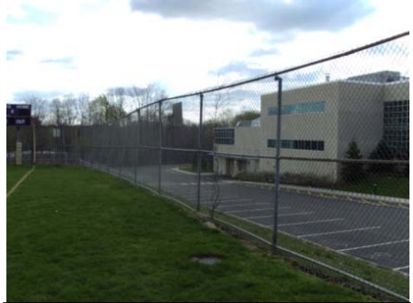
Photo #38: Chain link fencing condition at baseball field
