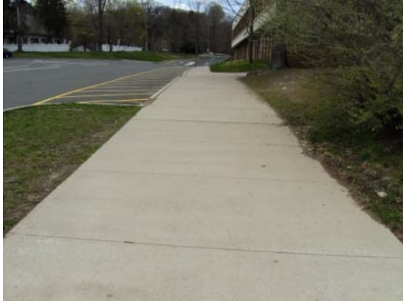
Photo #13: Concrete sidewalk at front of building
