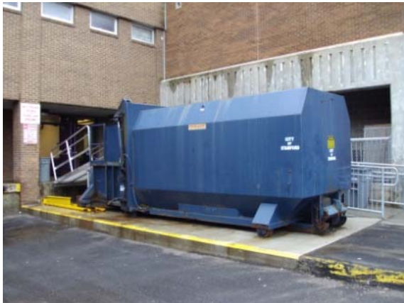
Photo #71: Compactor at rear loading dock
