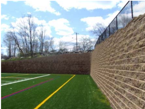
Photo #33: Masonry retaining wall adjacent to new soccer field
