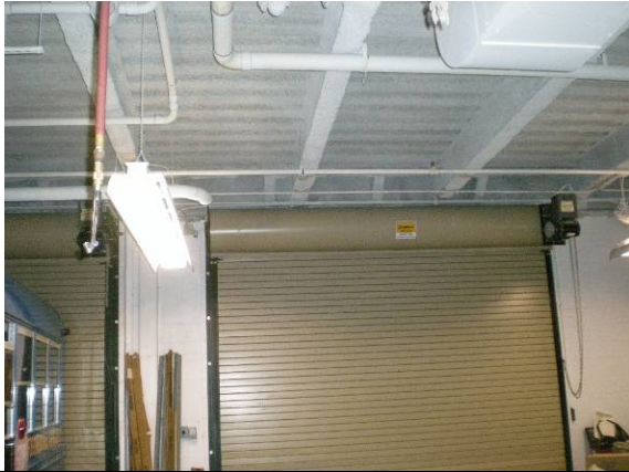
Photo #259: Roll up door and structure in new AgriScience Building
