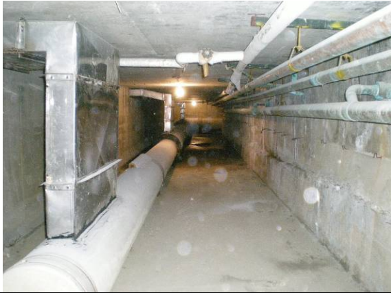
Photo #235: Structure at pool below grade
