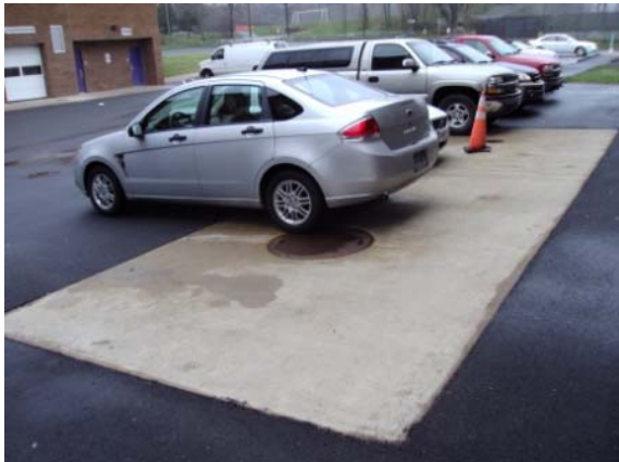
Photo #81: Underground 10,000-gallon fuel oil storage tank rear of main building
