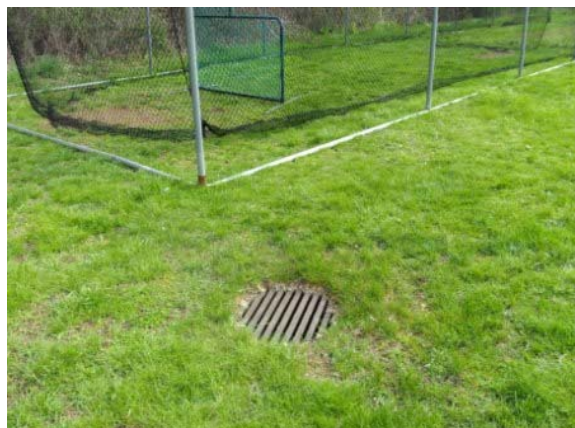
Photo #28: Drainage inlet at landscaping
