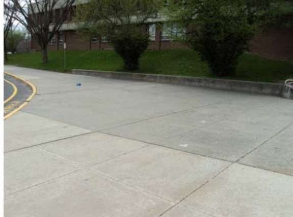
Photo #14: Concrete sidewalk at front of building
