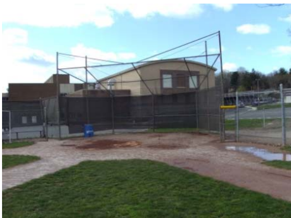
Photo #53: Baseball field chain link fence backstop
