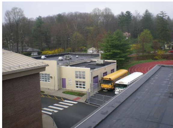
Photo #264: Roof overview of old AgriScience Building
