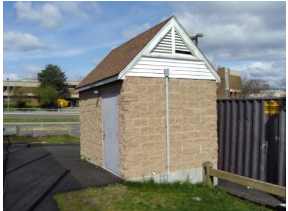
Photo #166: Old pump house building adjacent to new soccer field
