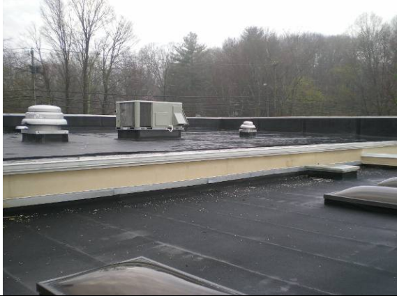
Photo #265: Roof overview of old AgriScience Building
