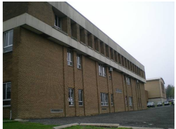
Photo #186: Partial north elevation of Finch (A) Wing
