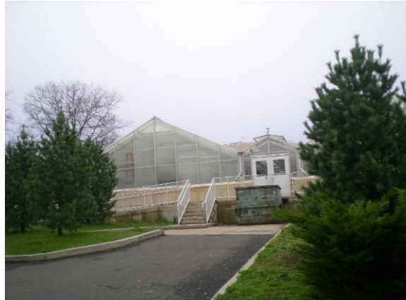
Photo #242: New AgriScience Building – southeast elevation
