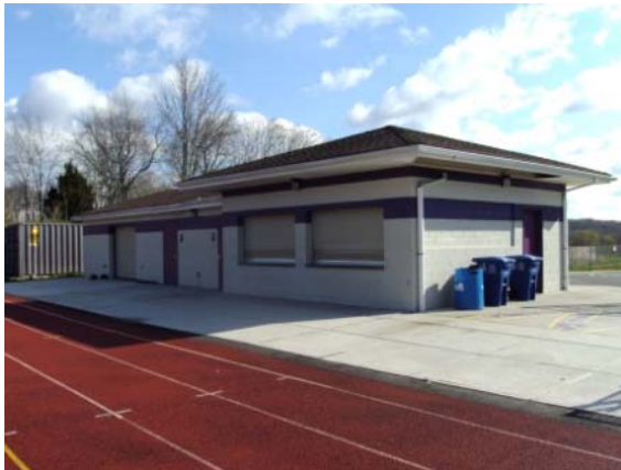
Photo #161: Concession stand building adjacent to football field
