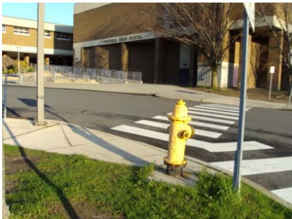
Photo #137: Fire hydrant at front of building
