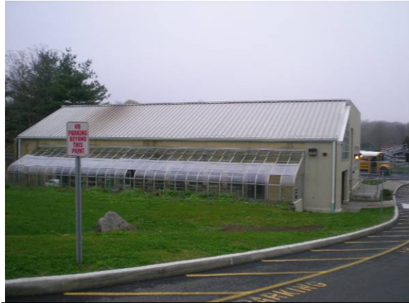
Photo #260: Old AgriScience Building – south elevation
