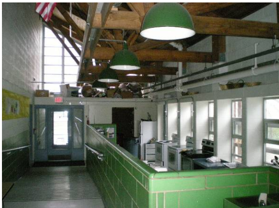
Photo #269: SPED classroom with kitchenette workstations and ADA access
