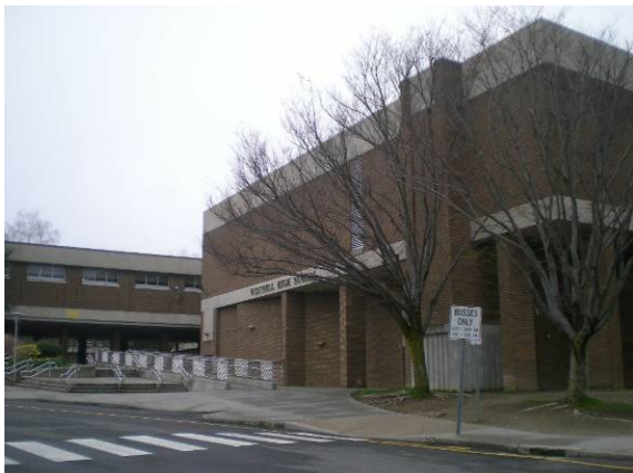
Photo #167: Main entrance and partial elevations
