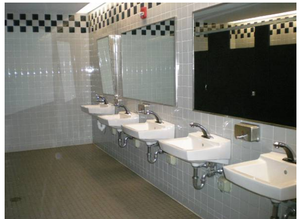
Photo #252: Restroom of new AgriScience Building
