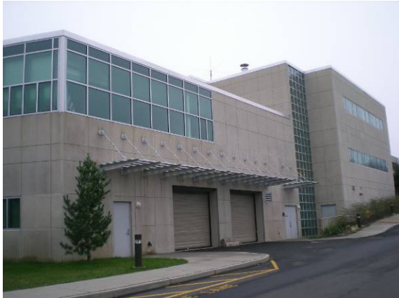
Photo #241: New AgriScience Building – north elevation
