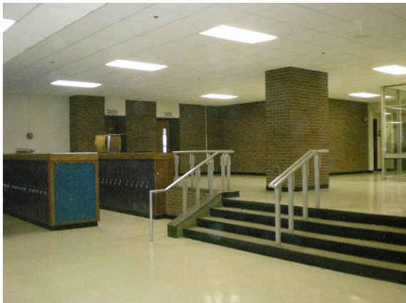
Photo #231: No ADA access to Main Office in Raynor (B) Wing
