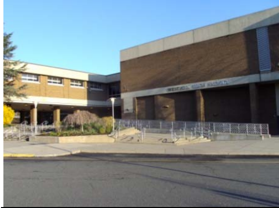
Photo #2: Front elevation of building and building identification signage
