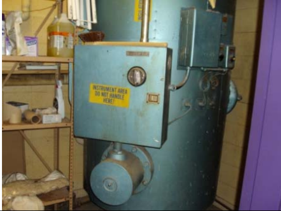
Photo #103: Domestic electric water heater at custodial closet
