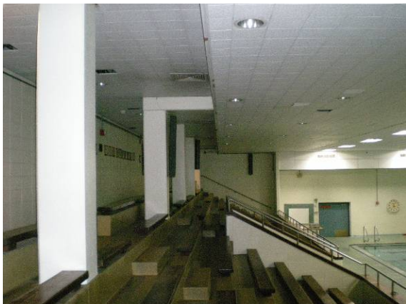
Photo #215: Bleacher seating in pool area
