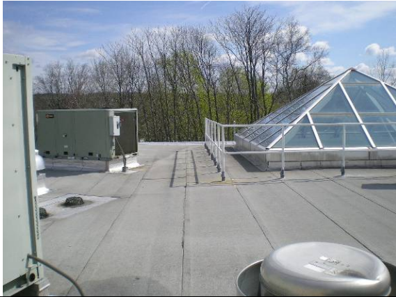
Photo #247: Roof overview – new AgriScience Building
