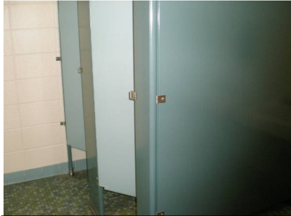
Photo #212: Teachers' restroom in Finch (A) Wing
