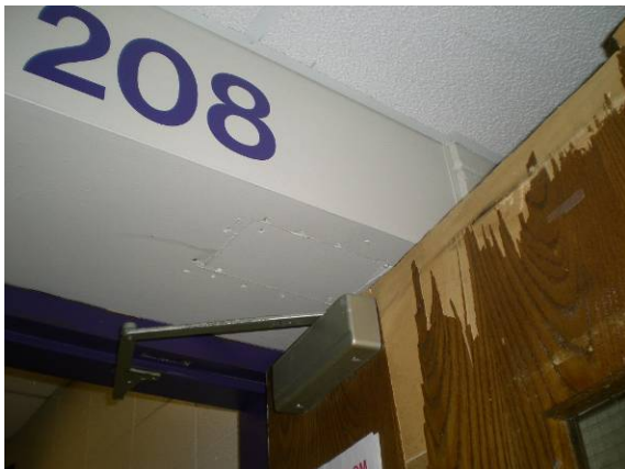
Photo #227: Condition of classroom door
