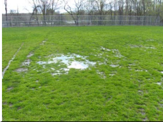
Photo #62: Softball field ponding and sink holes
