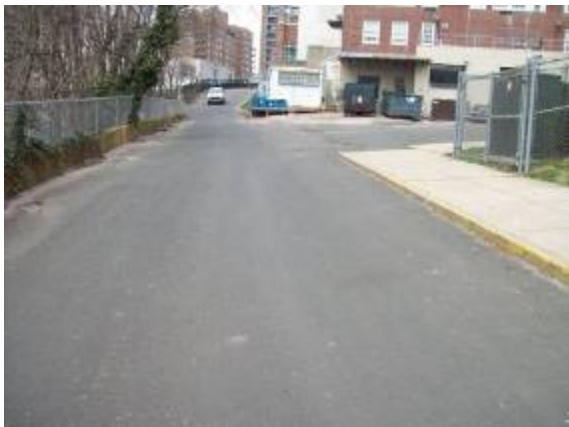
Photo #5: Drive aisle at south side
