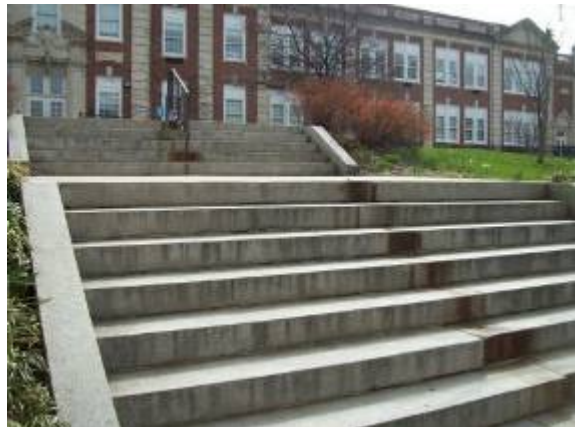
Photo #18: Concrete steps near Strawberry Hill Avenue
