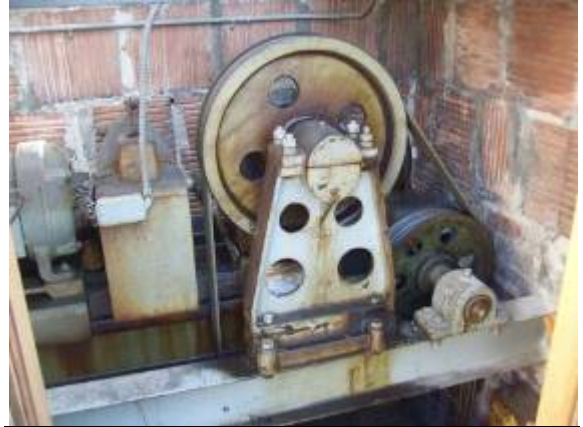
Photo #116: Elevator 4 traction equipment
