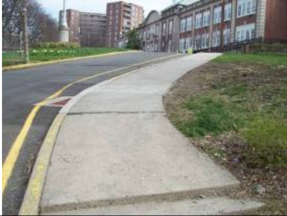
Photo #13: Sidewalks along front elevation
