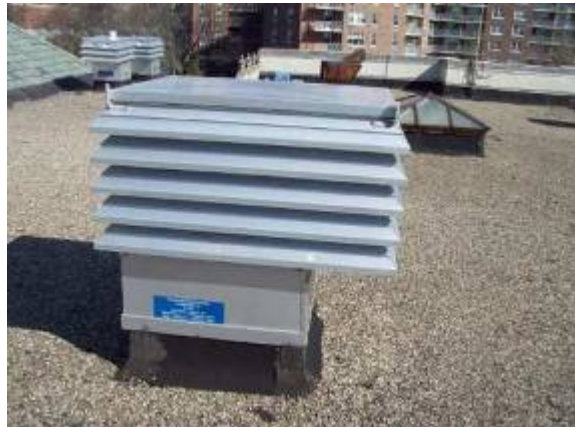
Photo #76: Typical exhaust louver
