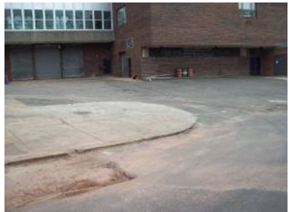
Photo #6: Maintenance parking area
