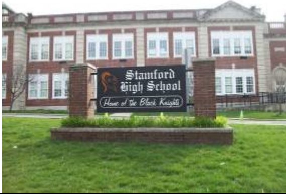
Photo #37: Property signage
