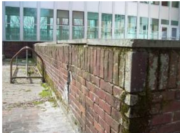
Photo #24: Retaining wall near building connector
