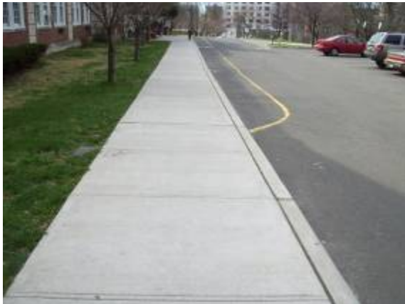
Photo #15: New sidewalk along front elevation
