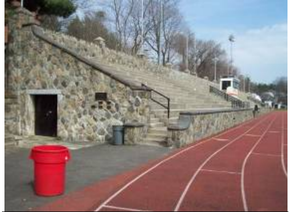
Photo #26: Seating structure at Boyle Stadium
