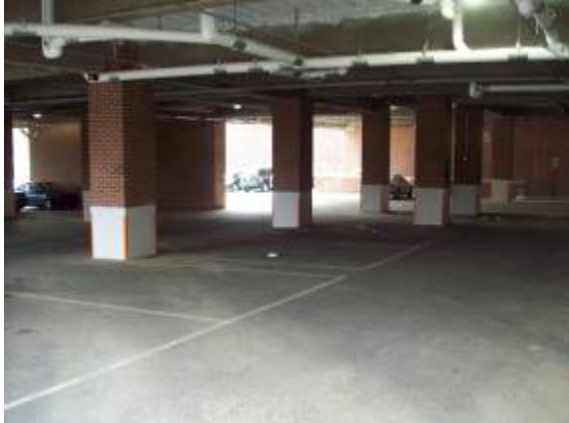
Photo #7: Parking area beneath 9 th grade wing
