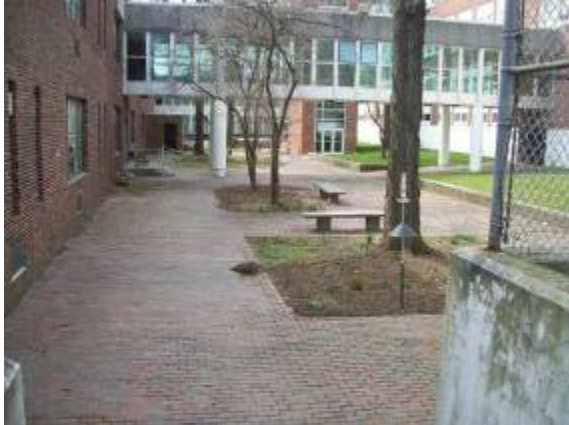
Photo #19: Brick pavers east of original building
