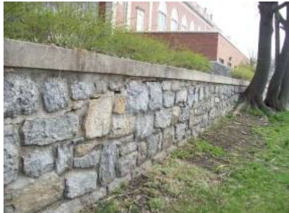
Photo #22: Retaining wall near south entrance
