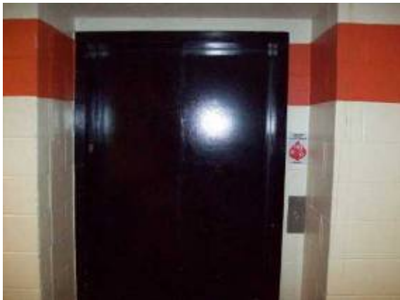
Photo #107: Elevator 2 cab doors
