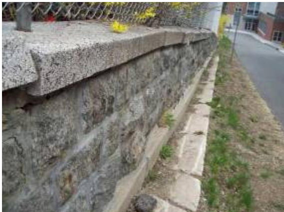
Photo #23: Retaining wall along north property line
