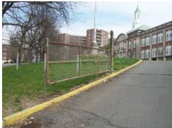
Photo #36: Damaged gate at south entrance
