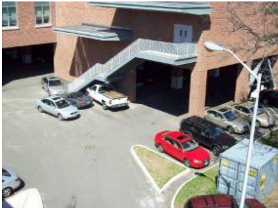
Photo #39: Site lighting
