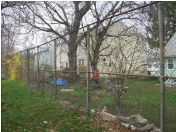
Photo #33: Old fencing near upper playing field
