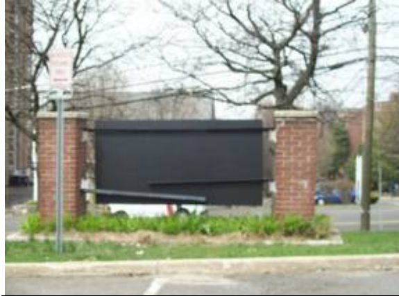
Photo #38: Minor damage to signage
