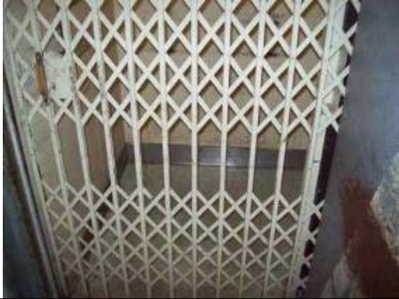
Photo #115: Elevator 4 cab interior
