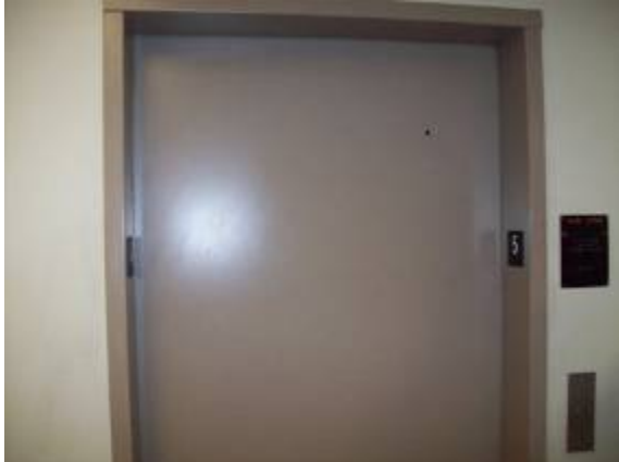
Photo #103: Elevator 1 cab doors
