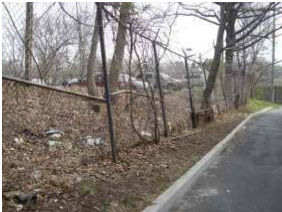
Photo #35: Damaged fencing along north property line
