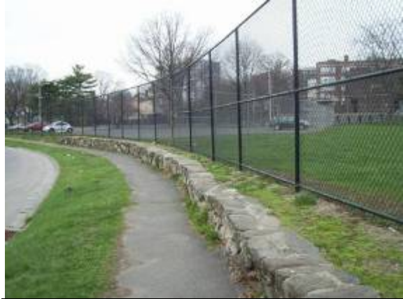
Photo #32: New fencing along Hillendale Avenue
