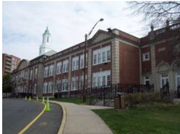
Photo #40: Site lighting
