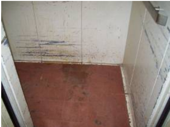
Photo #111: Elevator 3 cab interior
