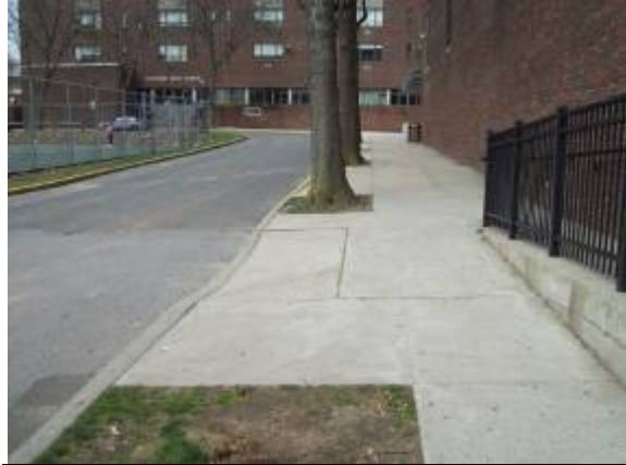
Photo #14: Sidewalks and drive aisle along gymnasium
