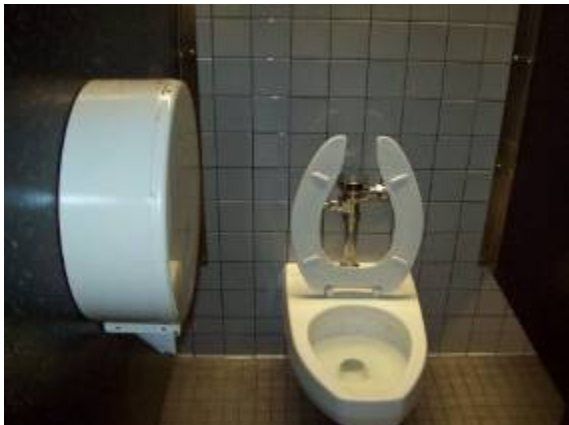
Photo #83: Restroom fixtures – water closet
