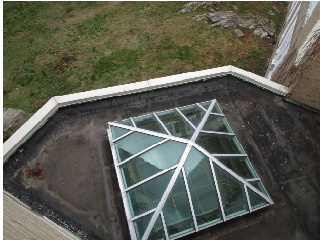
Courtyard corner roof with skylight
