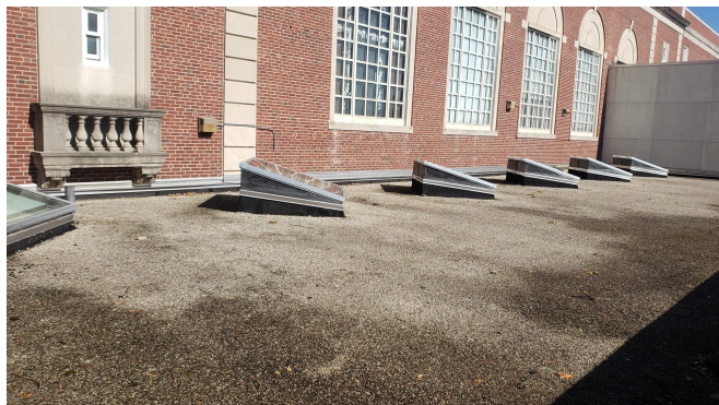
View of roof
