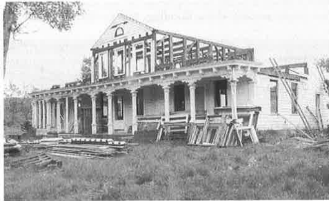
Dismantling of Bruchmann residence, May 2000
