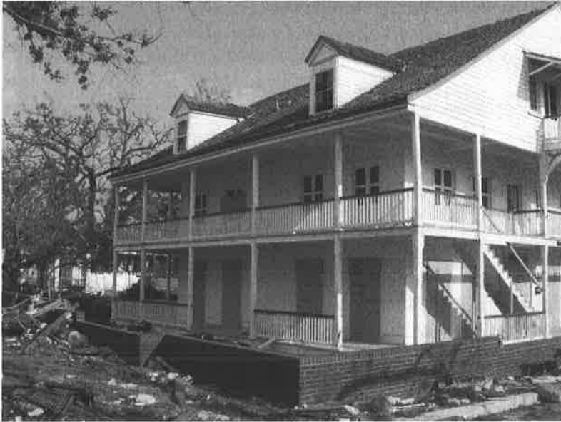
Built by John Holm in 1847, the Magnolia Hotel, badly damaged from Hurricane Camille in 1969, was moved 100 yards north and restored by the City of Biloxi in 1972. As a result, the hotel experienced only minimal flooding during Hurricane Katrina.
