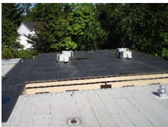
View of EPDM roof
