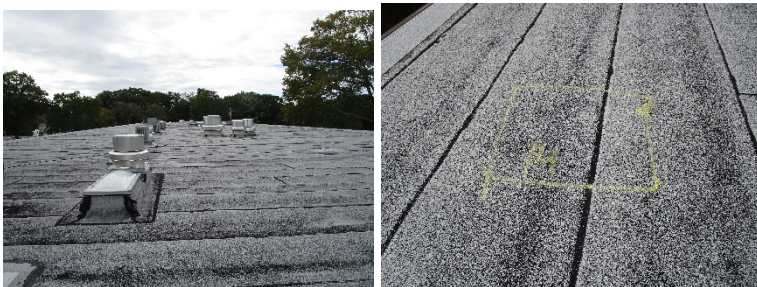
View of upper JM roof
