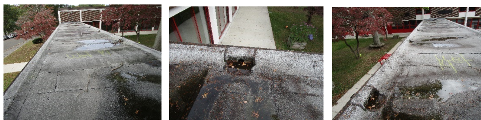
Views of the connector roof.
