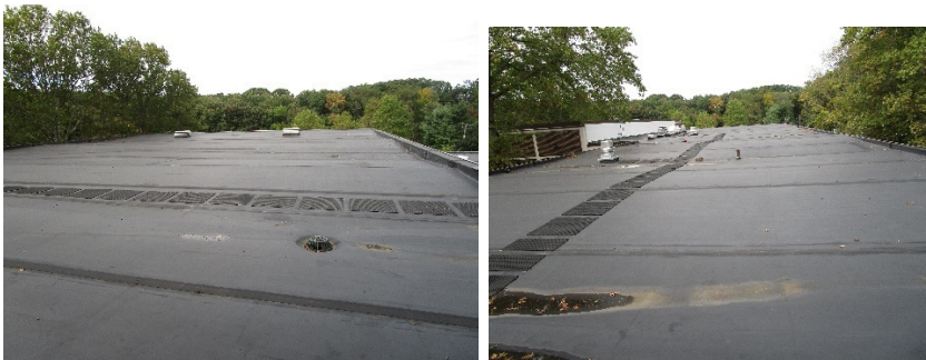
Views of the JM EPDM roof
