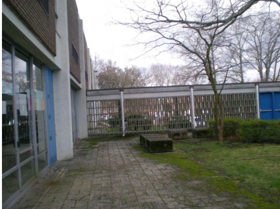
Photo #37: Courtyard pavers condition and partial elevations
