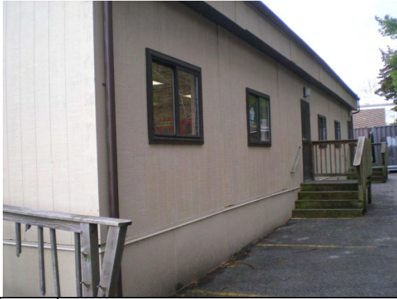
Photo #7: North elevation of modular addition
