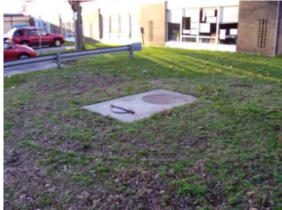
Photo #158: Underground 10,000-gallon fuel oil storage tank at rear of building
