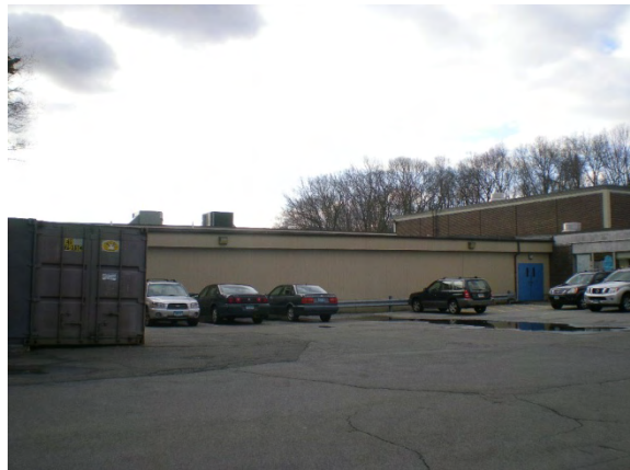
Photo #6: West elevation of modular addition
