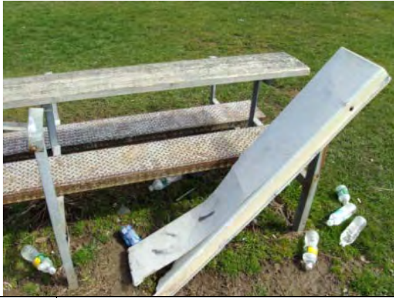
Photo #151: Damaged bleacher seat at soccer field
