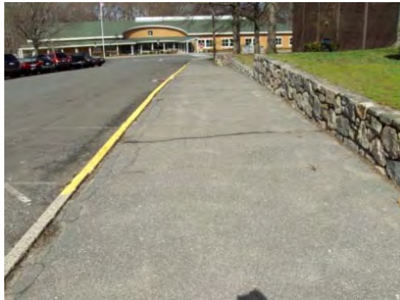
Photo #103: Asphalt sidewalk and curbing at side elevation
