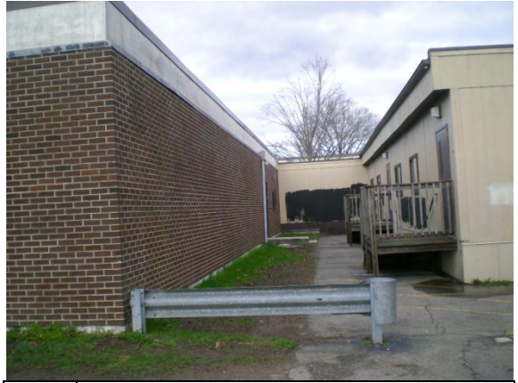
Photo #8: East elevation of modular showing connection to main building
