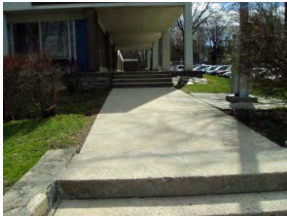
Photo #111: Concrete sidewalk at front elevation
