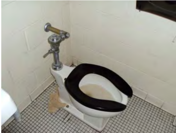
Photo #181: Floor-mounted toilet at restroom
