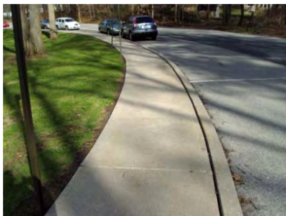
Photo #113: Concrete sidewalk and curbing along rear drive lane
