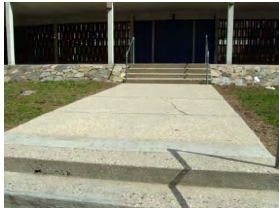
Photo #112: Concrete sidewalk at side elevation
