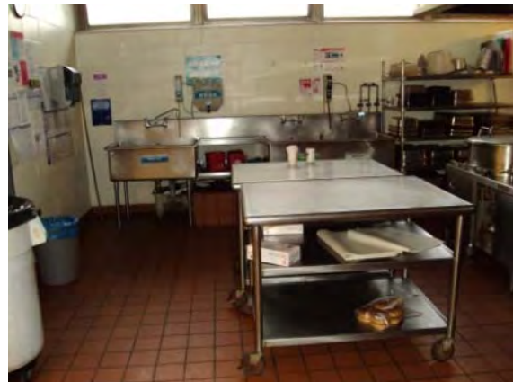
Photo #220: Kitchen work tables and 3-compartment sink and faucets
