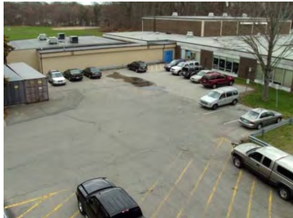
Photo #94: Parking lot at rear of building (north elevation)
