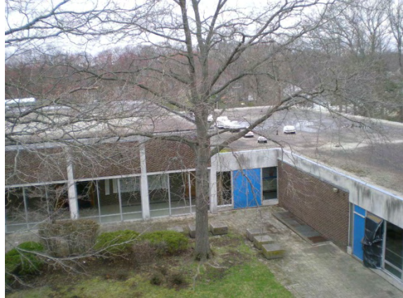
Photo #44: Courtyard elevations and roofs along classroom corridor and broken glass panel at right
