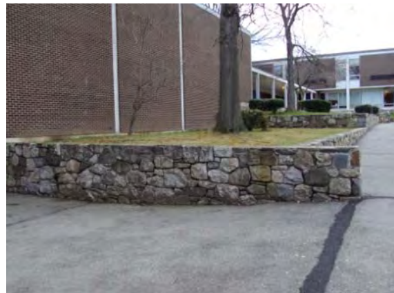
Photo #124: Stone masonry retaining walls along side elevation of building
