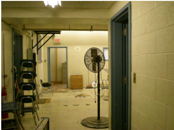
Photo #83: Lower level classroom with damaged flooring undergoing renovation
