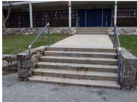
Photo #120: Concrete steps with metal handrails
