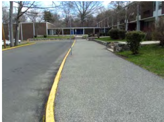
Photo #102: Asphalt sidewalk and curbing at front elevation
