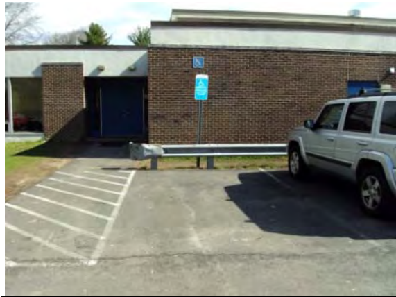
Photo #98: Accessible parking at right side of building (south elevation)
