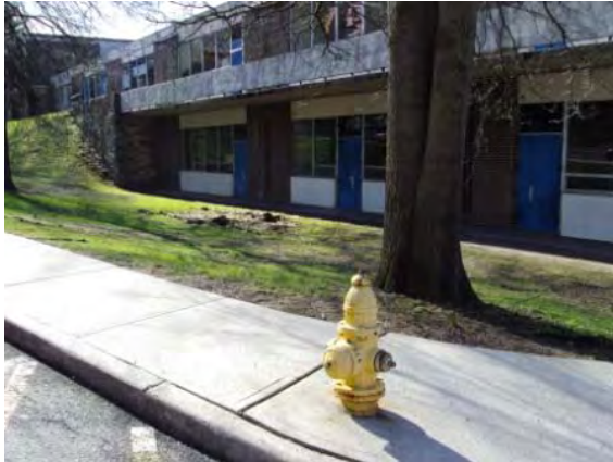
Photo #139: Fire hydrant at left side of building
