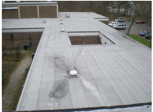
Photo #42: Roof overview along south section
