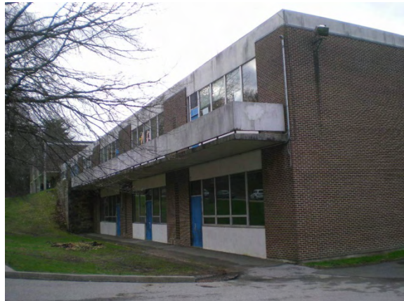
Photo #4: North elevation along service drive
