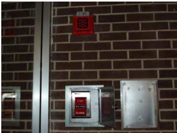
Photo #143: Fire pull station and strobe alarm
