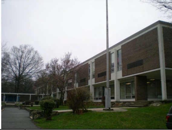
Photo #1: Front entrance elevation (west facing elevation)
