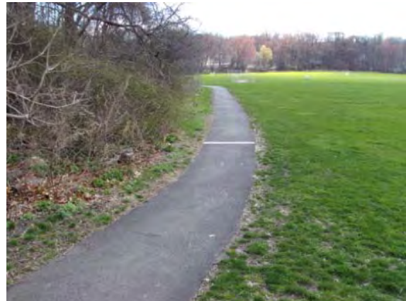
Photo #106: Asphalt walking path leading to playfields at the northeast elevation
