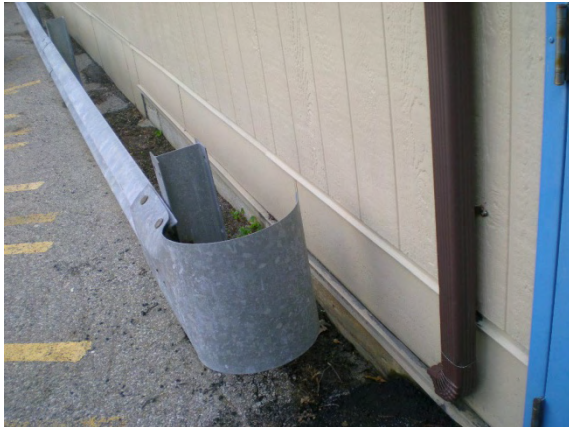
Photo #39: Modular addition slab connection at service yard area
