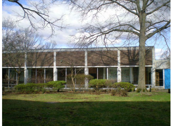
Photo #38: Courtyard elevation towards auditorium
