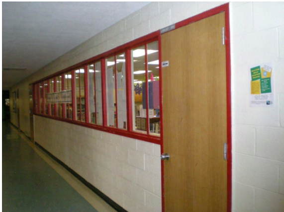
Photo #89: Entrance to Media Center with knob handle hardware
