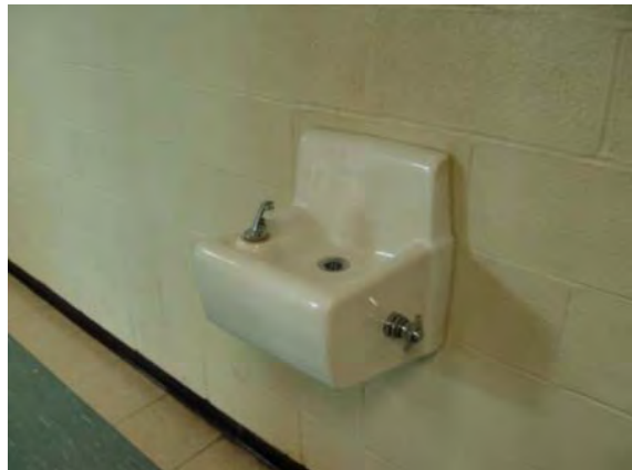
Photo #184: Common area drinking fountain at corridor
