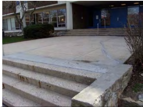
Photo #110: Concrete sidewalk leading to main entrance
