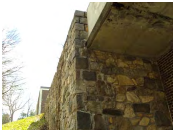
Photo #125: Stone masonry retaining wall at rear of building
