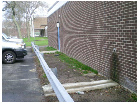
Photo #12: Partial south elevation showing storm water discharge onto parking lot
