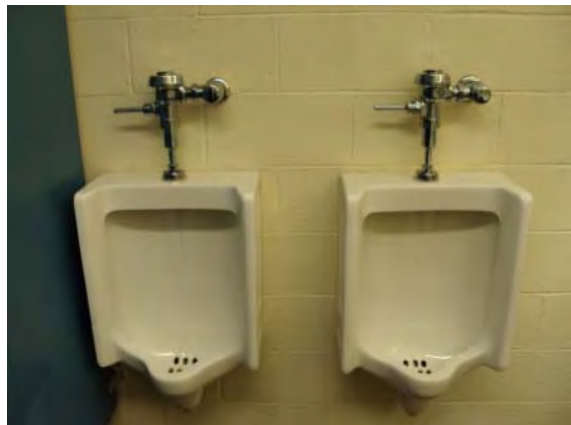
Photo #180: Boys common area restroom urinals
