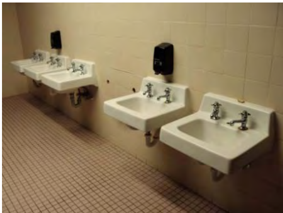
Photo #179: Common area restroom lavatory sinks
