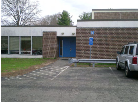
Photo #13: ADA entrance and parking at south entrance
