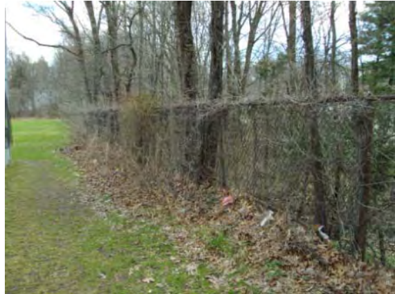
Photo #140: Chain link fencing adjacent to ball field (southeast elevation)
