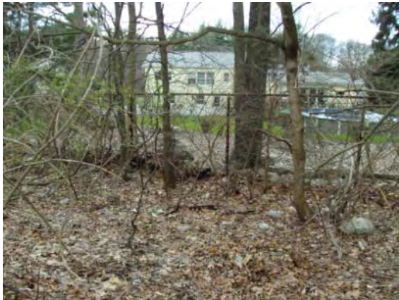
Photo #141: Chain link fencing along perimeter at southeast elevation
