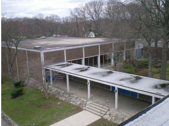
Photo #43: Roof overview of covered walkway and auditorium
