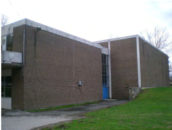
Photo #3: West elevation of auditorium and classrooms
