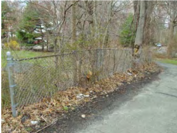
Photo #139: Chain link fencing along sidewalk leading to adjacent neighborhood (south elevation)
