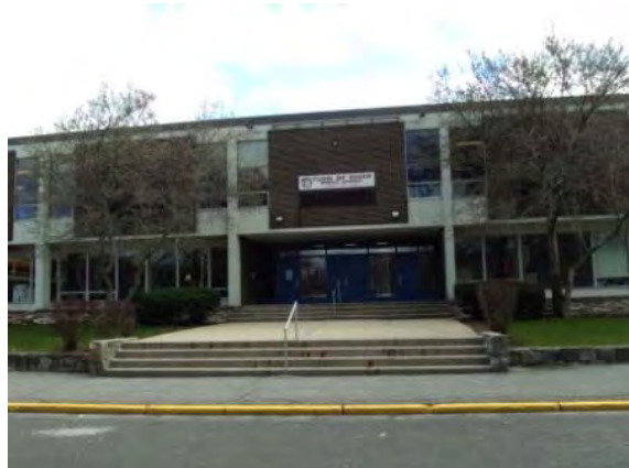
Photo #92: Front elevation of building and building identification signage (west elevation)
