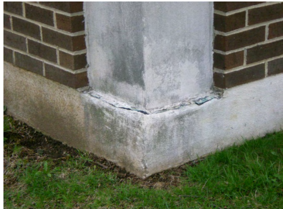
Photo #18: Patched base of column enclosure
