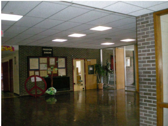
Photo #45: Main lobby
