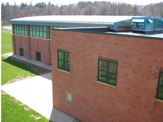
Photo #11: South sidewall and gymnasium exterior beyond
