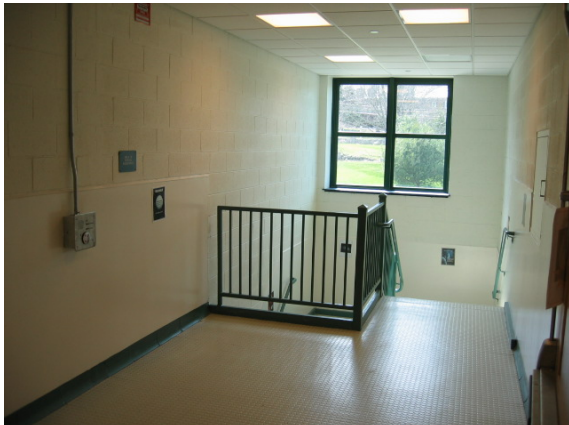
Photo #51: Each stairwell provides an area of refuge at top landing
