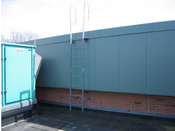
Photo #19: Roof levels are accessed by fixed ladders
