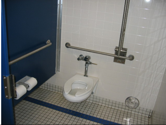
Photo #31: ADA accessible toilets are provided in cafeteria
