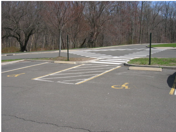
Photo #3: Two handicapped accessible parking stalls are provided in the rear
