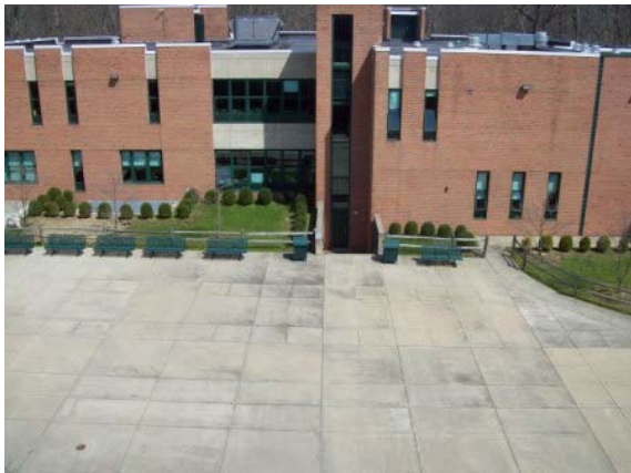
Photo #137: Concrete pedestrian area in courtyard
