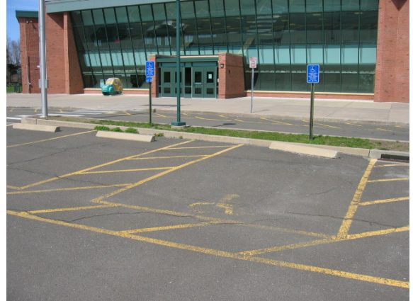
Photo #2: Five handicapped accessible parking stalls are provided in front
