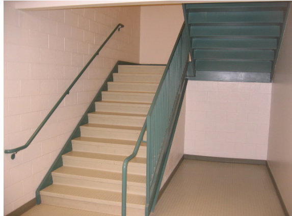
Photo #46: Several stairwells provided access and egress to the 2 nd floor
