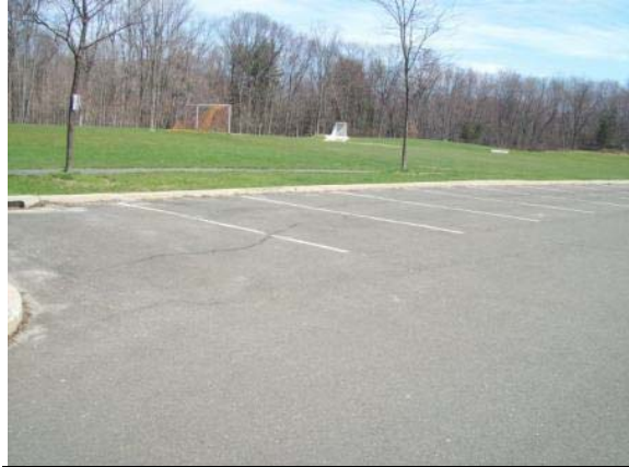
Photo #128: Asphalt detail
