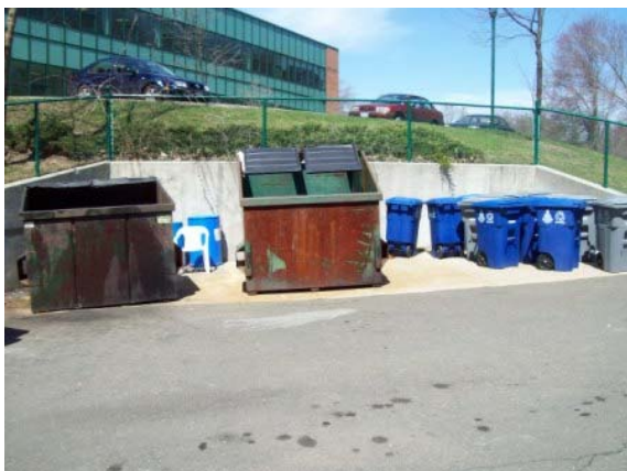
Photo #149: Dumpster pad and retaining wall
