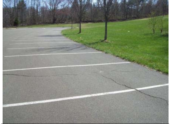
Photo #134: Asphalt with no curbing
