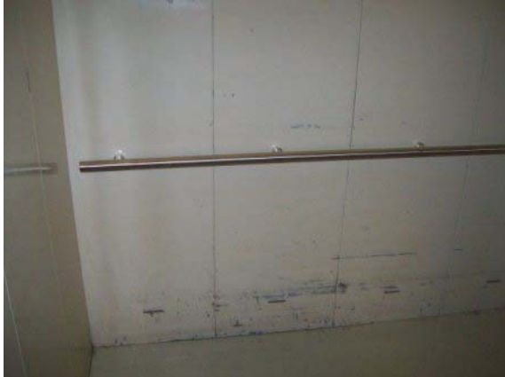
Photo #115: Cafeteria elevator cab interior
