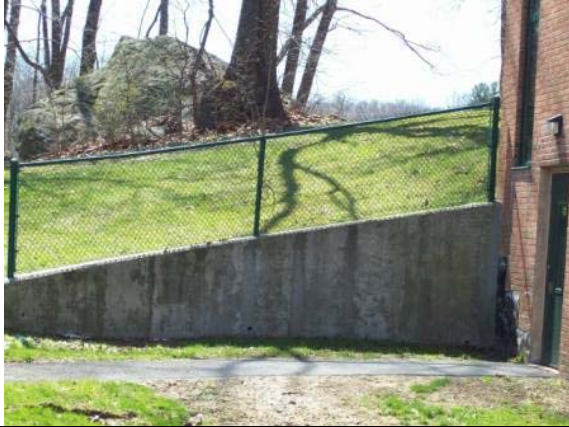
Photo #139: Concrete retaining wall at east side of building
