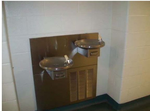
Photo #100: Typical drinking fountains
