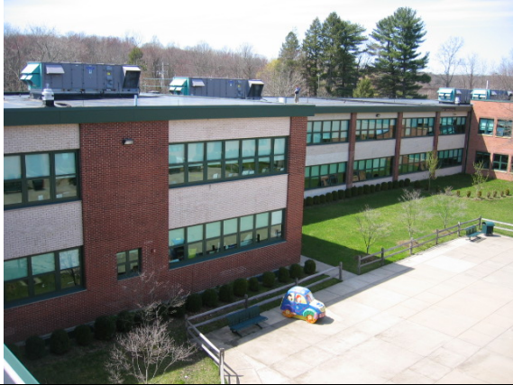
Photo #13: West side of the inner courtyard area
