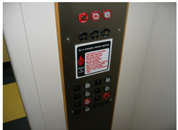
Photo #66: Each elevator provides substantial ADA access
