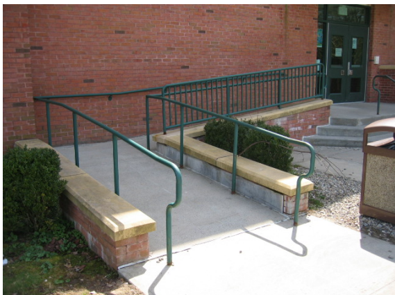
Photo #5: Typical secondary common entrance with steps and an ADA ramp
