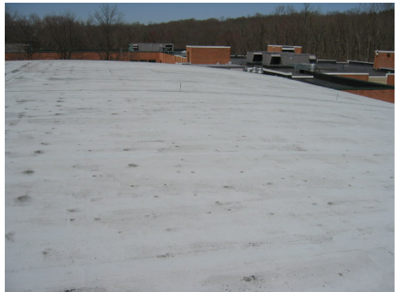
Photo #18: The gymnasium is covered with a shallow barrel vaulted EPDM
