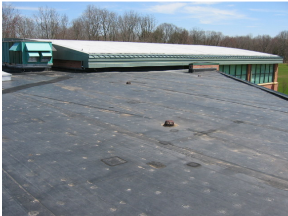
Photo #15: Overview of the flat and shallow barrel vaulted EPDM roofs
