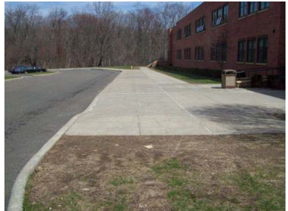
Photo #136: Concrete sidewalk
