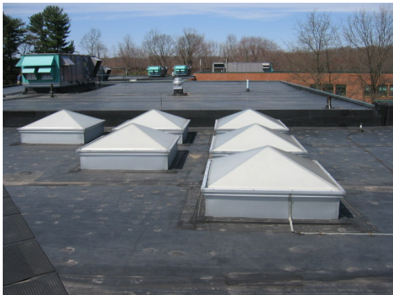
Photo #17: Several skylights are provided above the 2 nd floor atrium lobby
