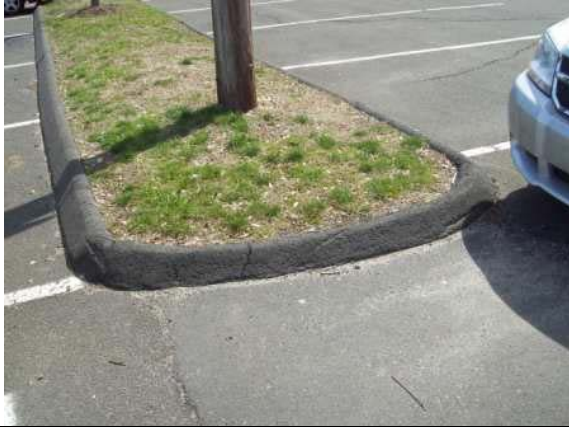
Photo #133: Extruded asphalt curbing
