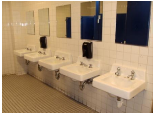
Photo #156: Common area restroom lavatory sinks
