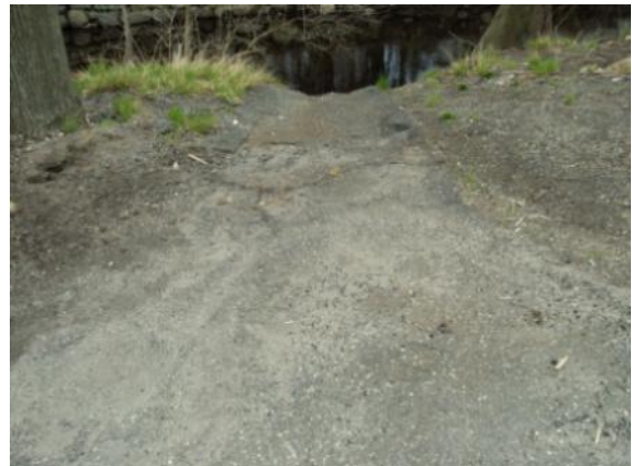
Photo #106: Asphalt swale draining to river at east elevation
