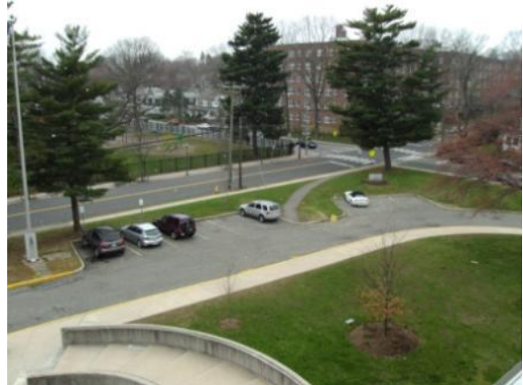
Photo #68: Parking area at front of building, with two accessible parking stalls
