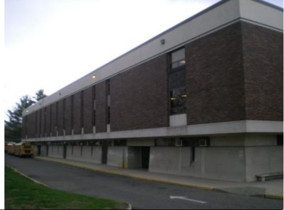
Photo #2: Right side elevation - west
