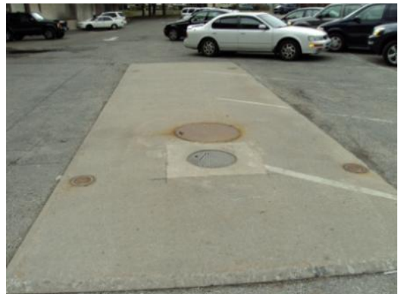
Photo #126: Underground 10,000-gallon fuel oil storage tank at rear of building
