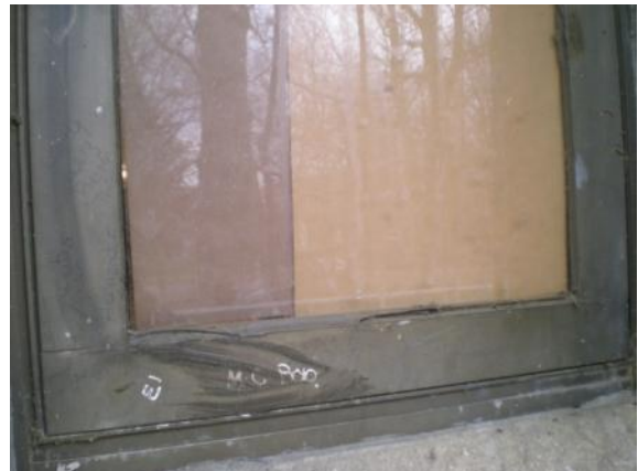
Photo #16: Condition of window sealant and glazing compound
