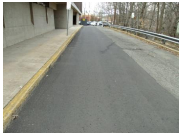
Photo #66: Drive lane at right side of building (east elevation)
