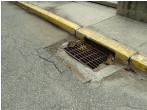
Photo #105: Drainage inlet
