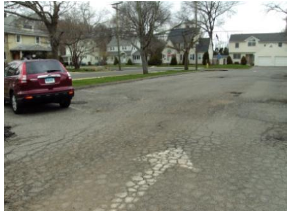
Photo #70: Parking area at the northwest corner of property
