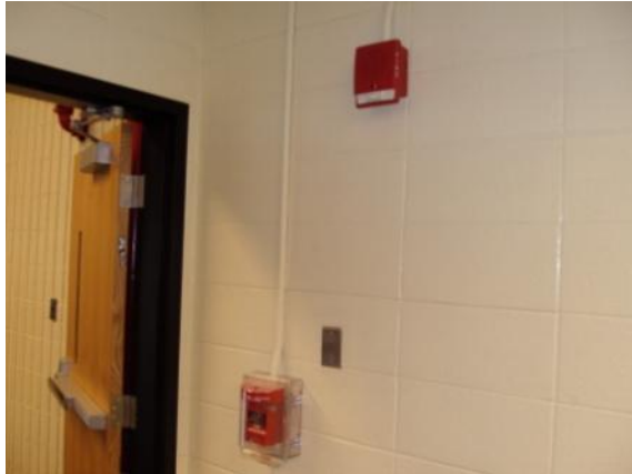
Photo #187: Fire pull station and strobe alarm
