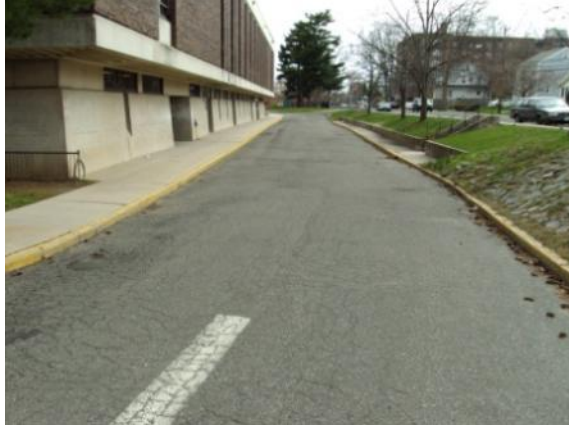
Photo #67: Drive lane at left side of building (west elevation)
