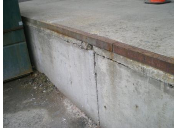
Photo #50: Loading dock conditions
