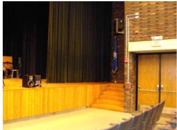
Photo #178: Auditorium stage requiring a wheelchair lift for accessibility
