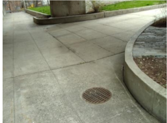
Photo #110: Concrete sidewalks and retaining walls at front elevation
