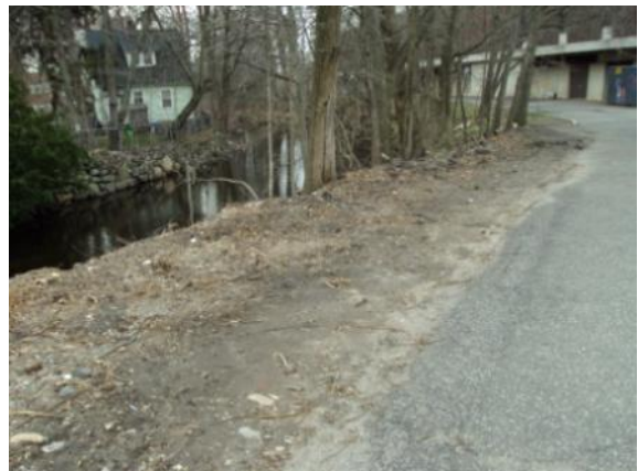
Photo #120: Landscape condition along east elevation (adjacent to river)
