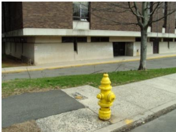
Photo #179: Fire hydrant along Powell Place
