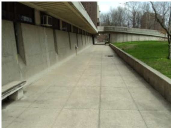
Photo #89: Concrete sidewalk along front of building
