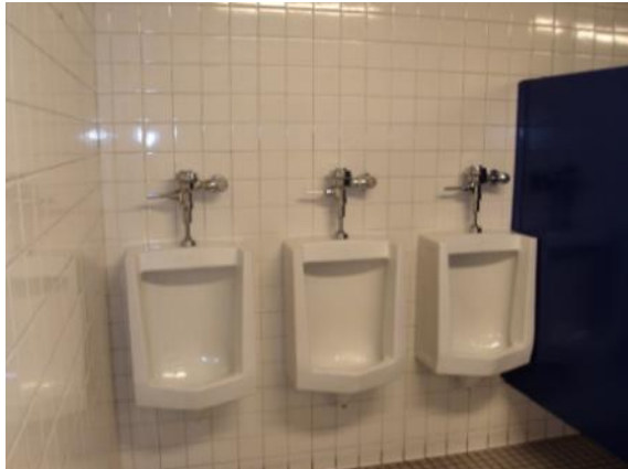
Photo #159: Boys common area restroom urinals
