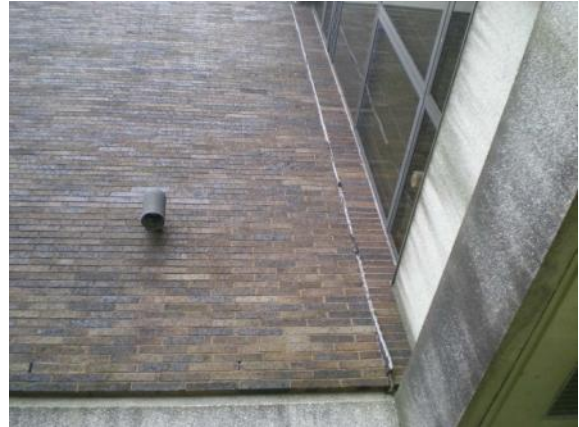
Photo #44: Condition of control joint
