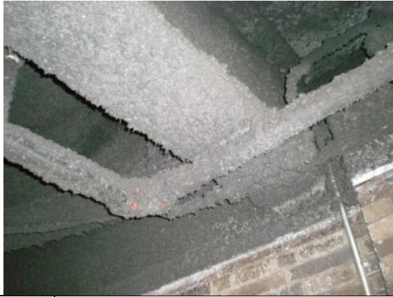
Photo #25: Fire proofing at auditorium ceiling
