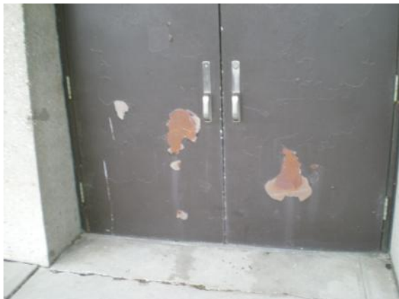
Photo #9: Condition of service doors
