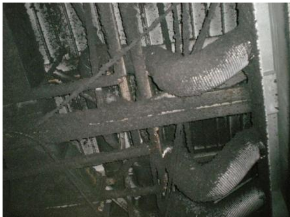
Photo #53: Fire-proofing in auditorium condition
