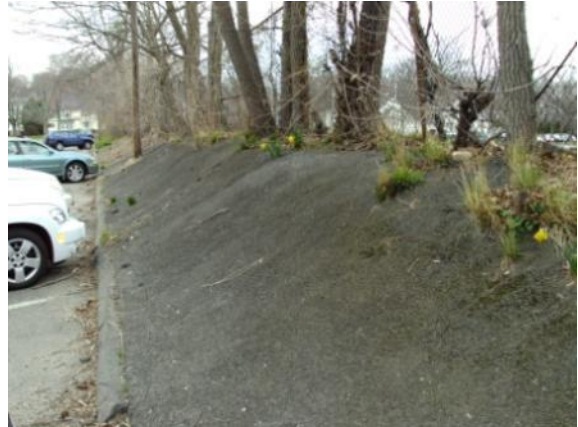
Photo #116: Asphalt overlay on landscape hill at north property line
