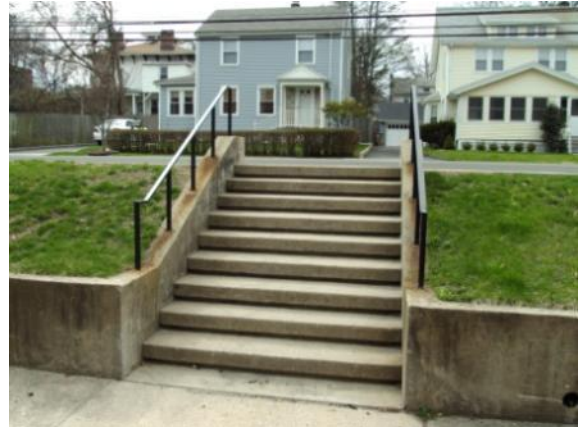
Photo #98: Concrete steps and retaining walls at west elevation
