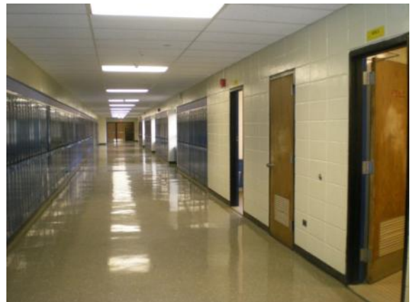
Photo #48: Typical corridor
