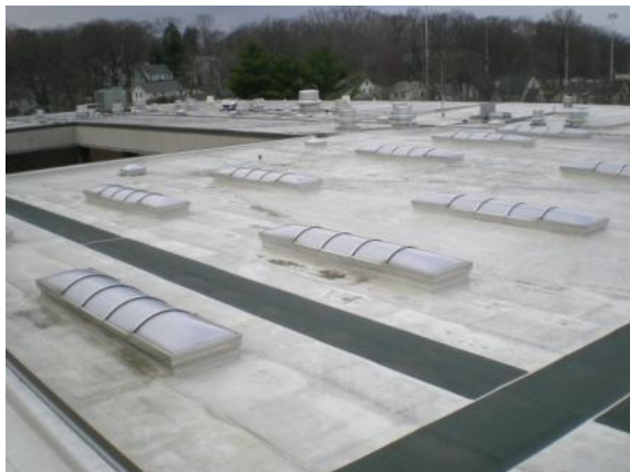
Photo #17: Roof overview
