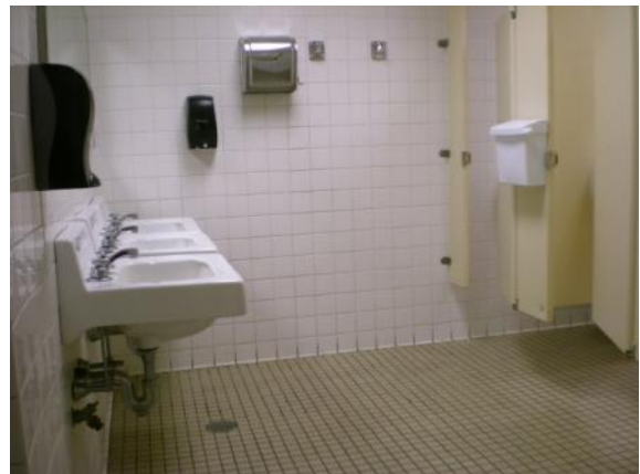
Photo #30: Common area restrooms
