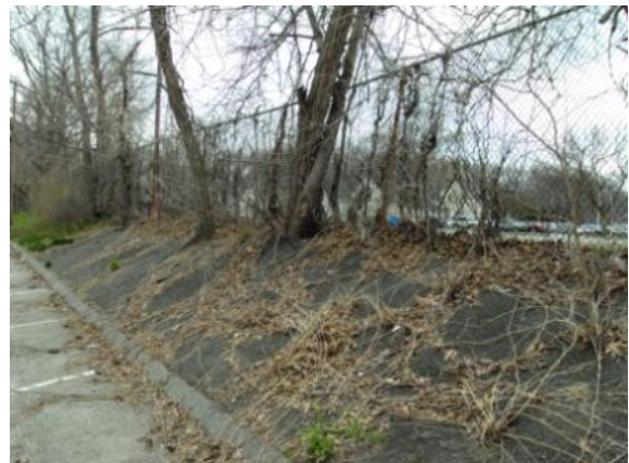
Photo #114: Asphalt overlay on landscape hill and excessive vegetation at north property line
