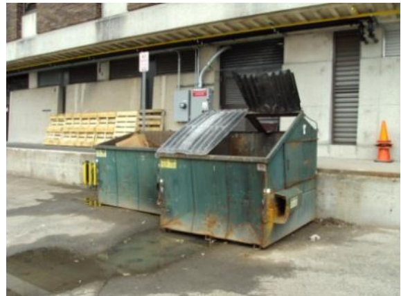
Photo #124: Dumpsters set on asphalt pavement adjacent to rear loading dock
