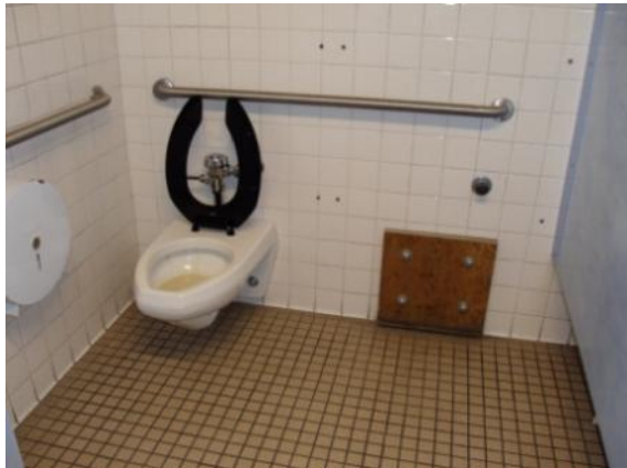
Photo #161: Toilet removed to make ADA stall at common area restroom
