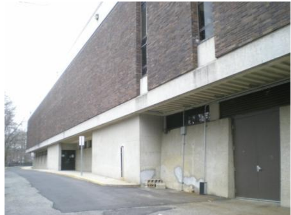
Photo #4: Left elevation - east
