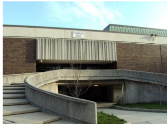
Photo #64: Front elevation of building and building identification signage (south elevation)
