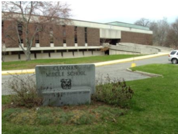
Photo #63: Project site and signage at front elevation
