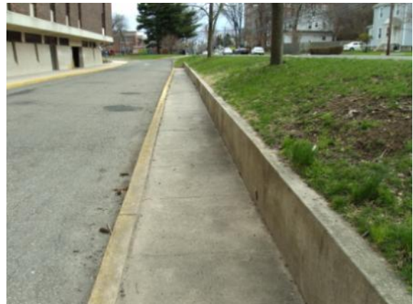
Photo #88: Concrete sidewalk, curbing and retaining wall at west elevation
