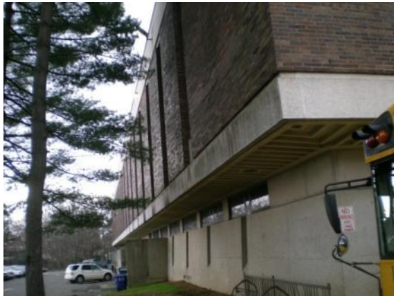
Photo #3: Rear elevation - north
