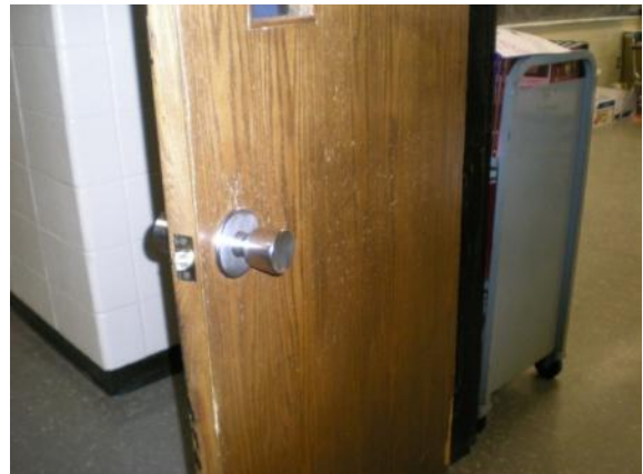
Photo #52: Typical classroom door lockable from outside room only
