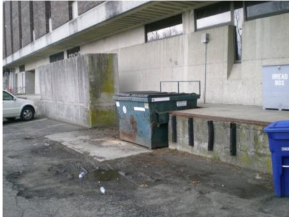
Photo #13: Loading dock conditions
