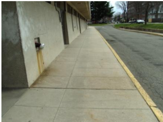
Photo #87: Concrete sidewalk and curbing along left side of building
