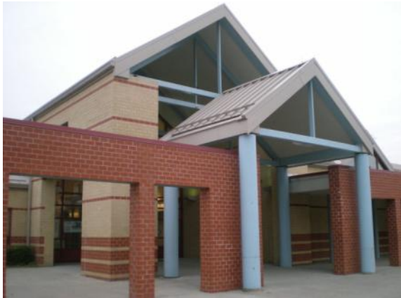
Photo #69: Front entrance canopy
