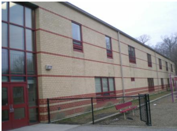
Photo #78: North elevation
