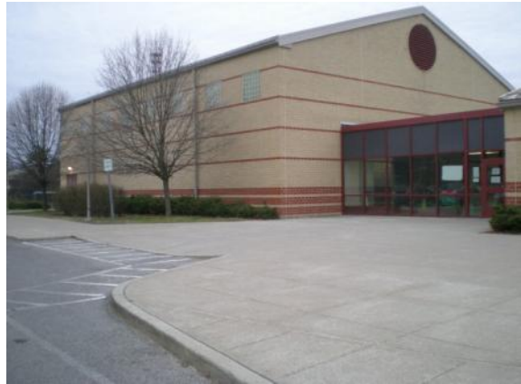
Photo #70: Front elevation of gymnasium
