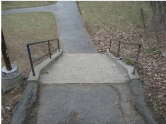
Photo #10: View of cast in place concrete steps.
