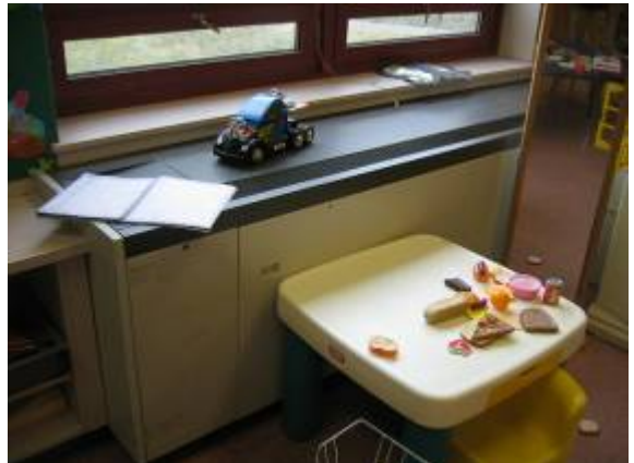
Photo #30: View of fan coil unit.
