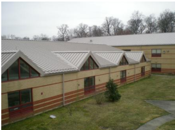
Photo #83: Kindergarten north elevation within courtyard
