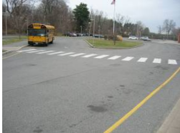
Photo #2: View of asphalt paved entry drive.
