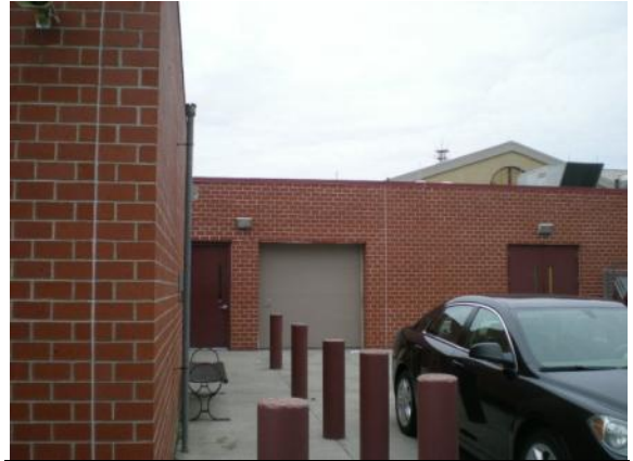
Photo #80: Trash bin garage entrance
