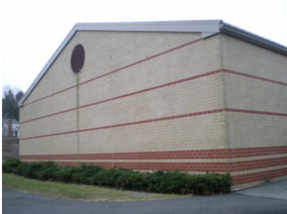
Photo #81: North elevation of auditorium
