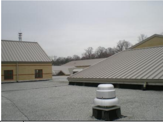
Photo #85: Roof overview
