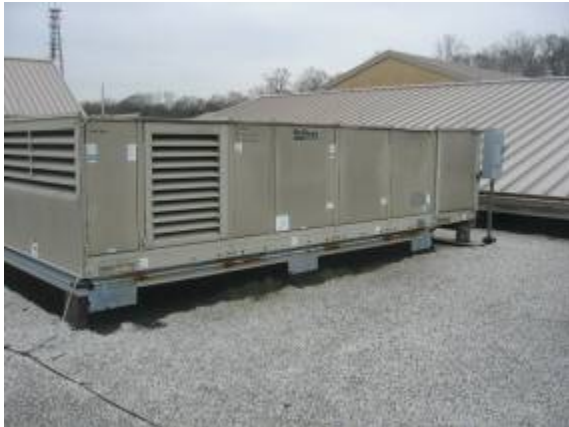
Photo #39: View of RTU-6.
