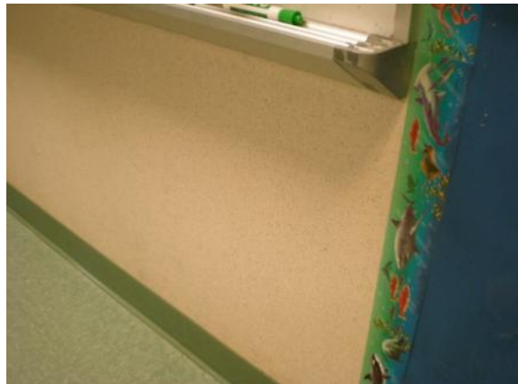
Photo #118: Close up of multi-paint system in classroom
