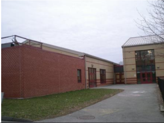
Photo #79: North side entrance
