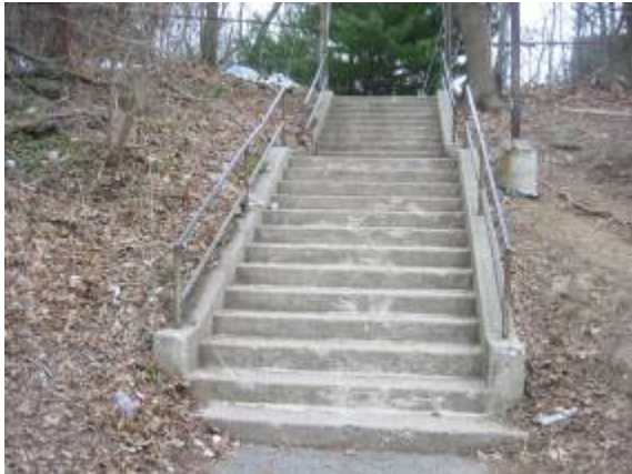
Photo #9: View of cast in place concrete steps.
