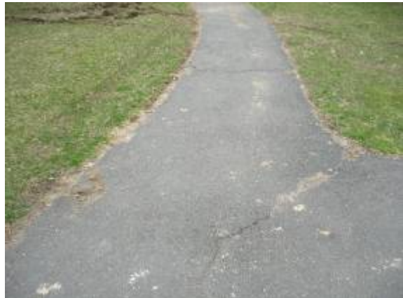
Photo #6: View of asphalt paved sidewalks.
