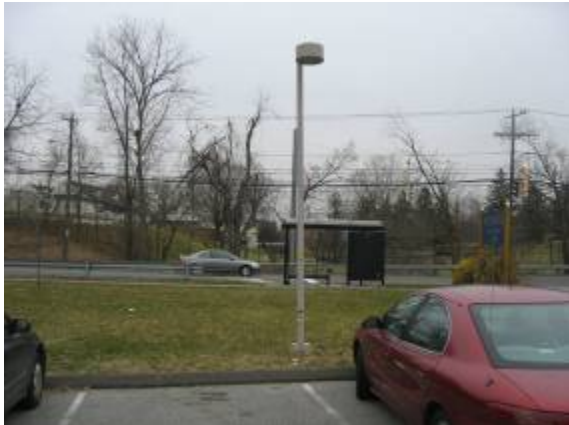
Photo #3: View of pole mounted lighting fixtures.
