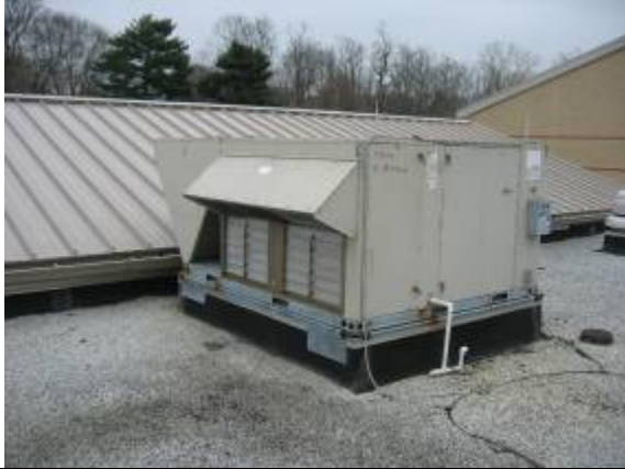
Photo #37: View of RTU-4.
