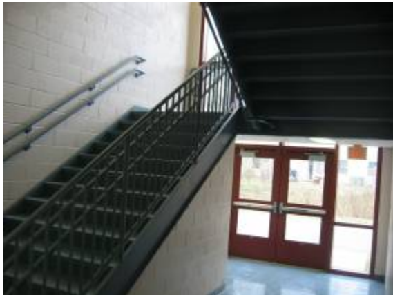
Photo #59: View of fire stairwell.
