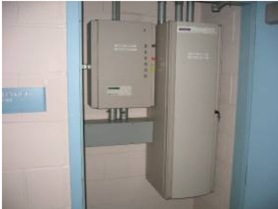
Photo #63: View of auditorium lighting system.
