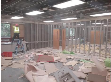
Removal of all interior sheet rock walls, ceiling tiles and insulation
