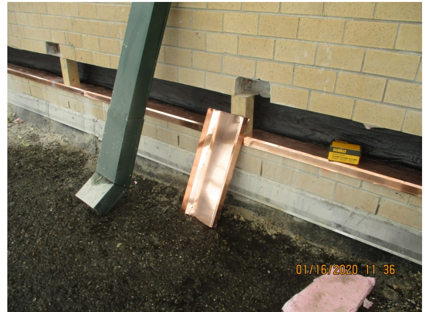
Roof Flashing replacement.
