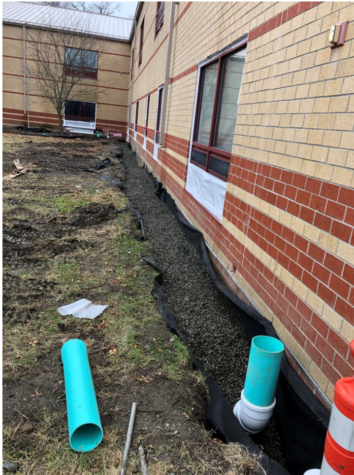
New building under drain in courtyard and around building perimeter
