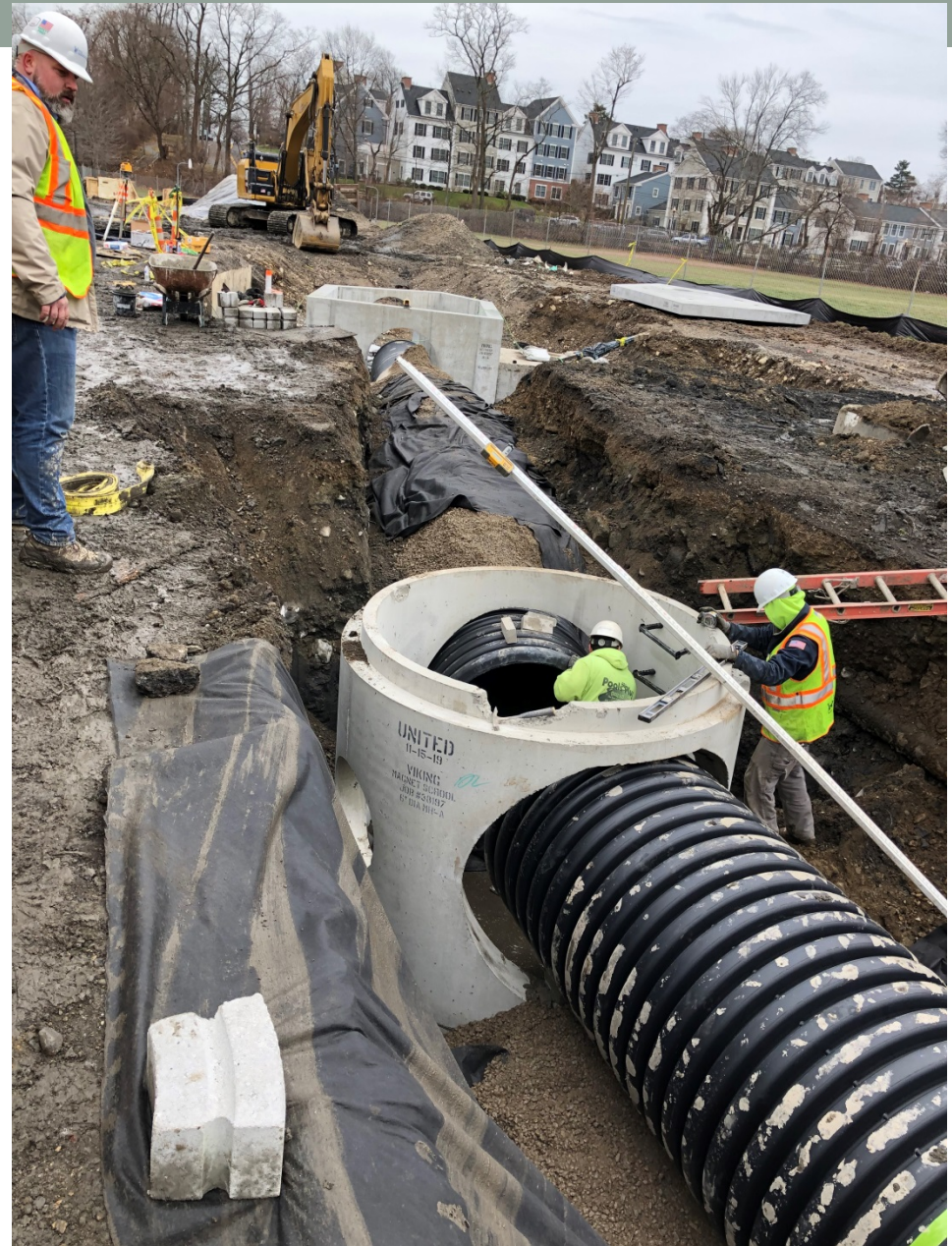
New 60" culvert bypass piping
