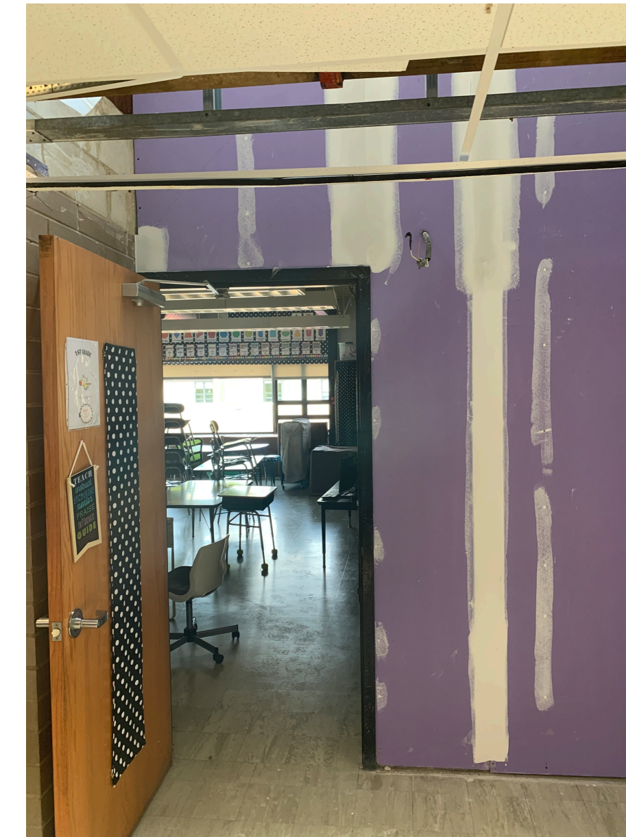
Entry of Room 2 GWB Repair
