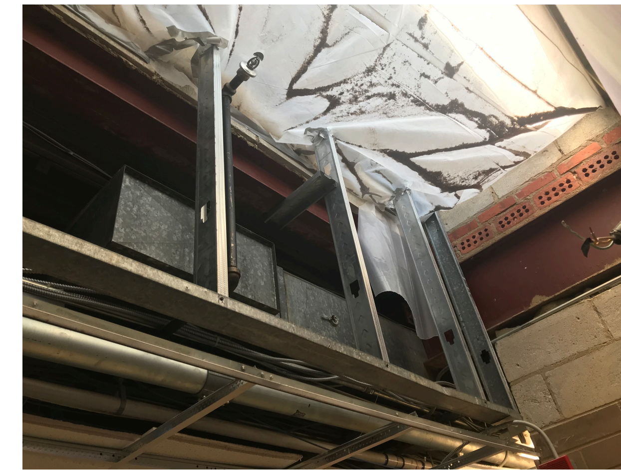
Hallway GWB Repair under skylight framing
