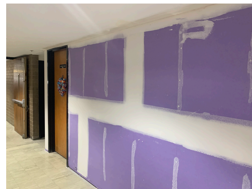
Hallway GWB Repair between Rooms 1 and 7
