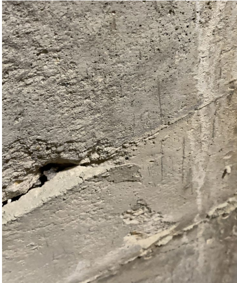
Photo # 9: Pitting and cracking of interior foundation wall.
