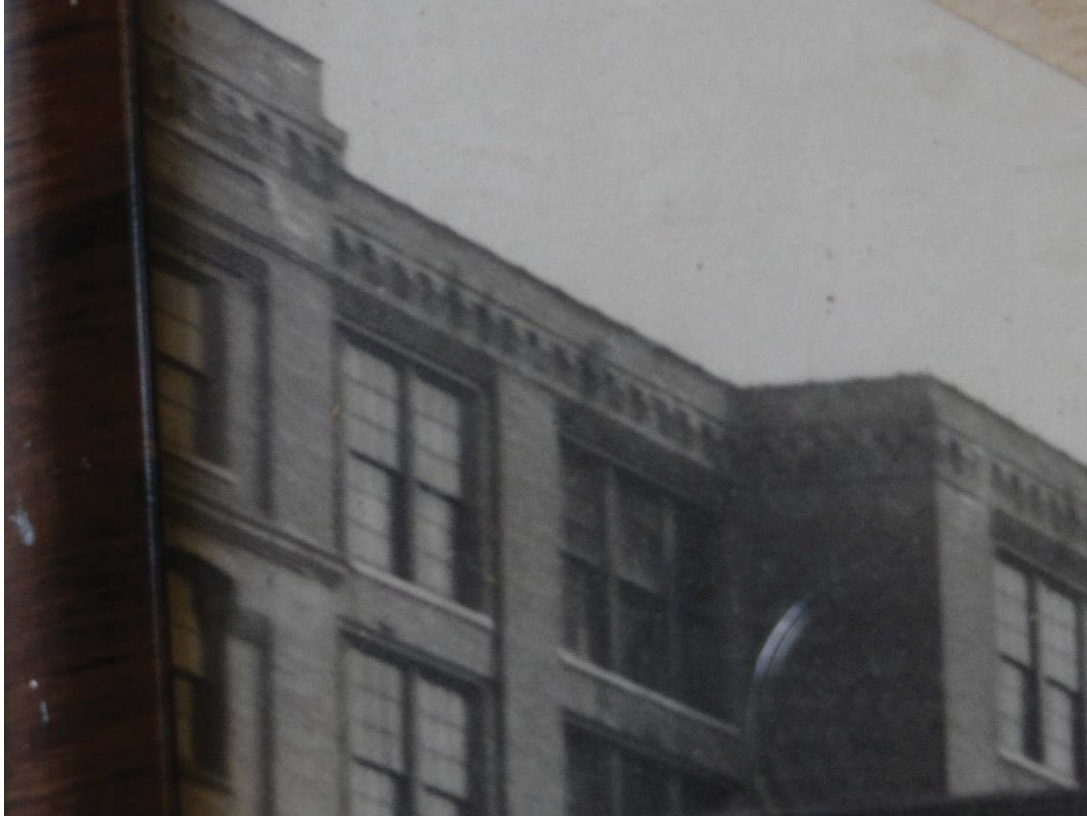
Architectural Reference- Yale & Towne Lock Company, Windows and Cornice
