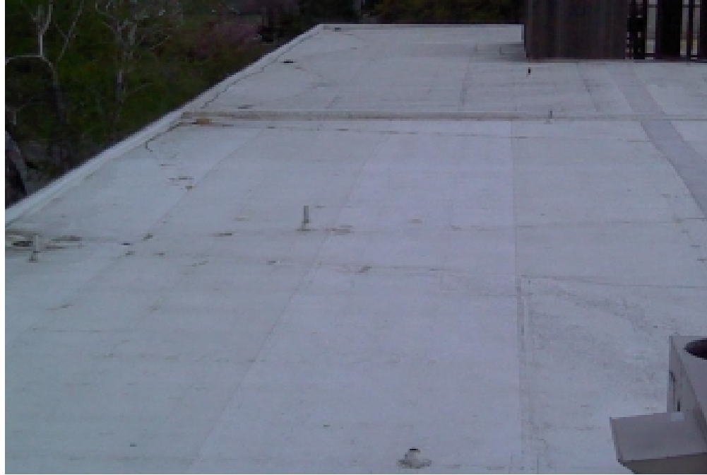
Dry area of roofing
