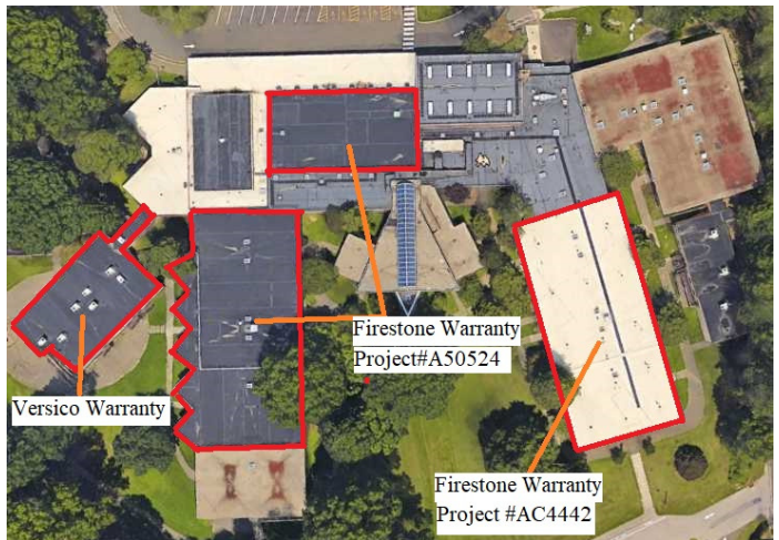
Roof areas with active warranties
