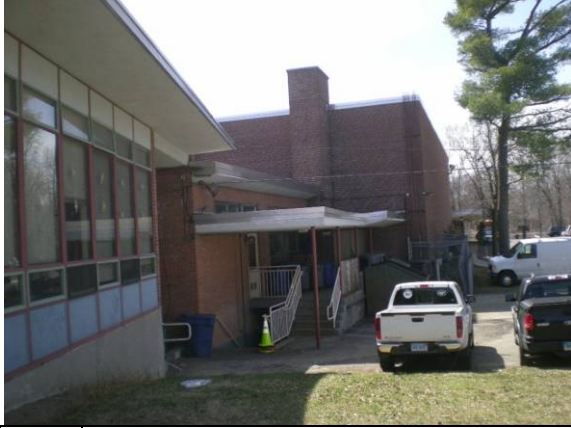
Photo #79: Loading dock and gym
