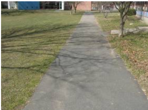
Photo #5: View of asphalt paved sidewalks.
