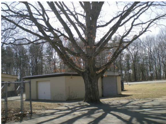
Photo #95: Storage building at south end of property
