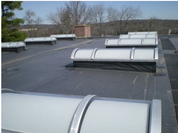
Photo #89: Roof over cafeteria
