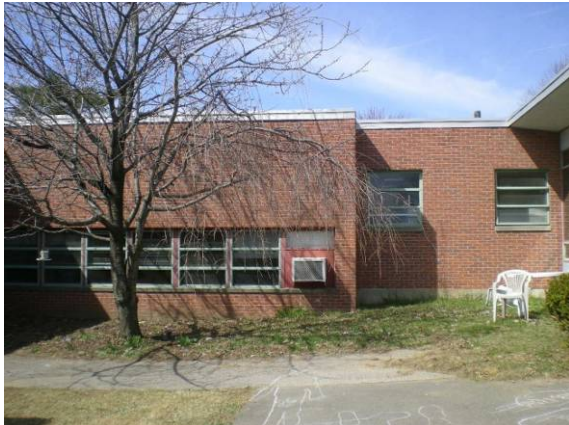
Photo #75: Elevation between 400 wing and 500 wing addition
