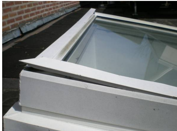
Photo #90: Close up detail of skylight
