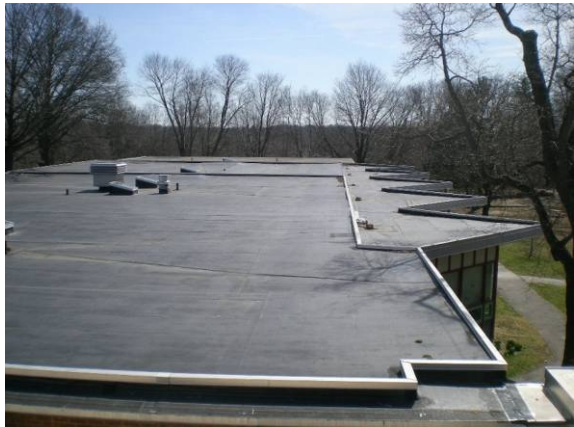
Photo #84: Roof overview over 200 wing
