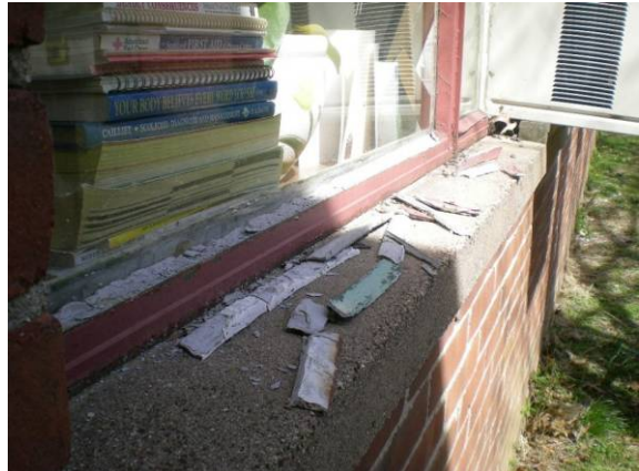
Photo #100: Condition of original windows
