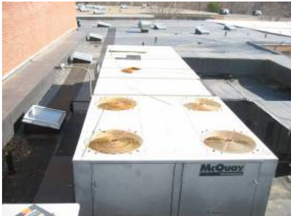
Photo #31: View of ACC-1, which serves the media center.
