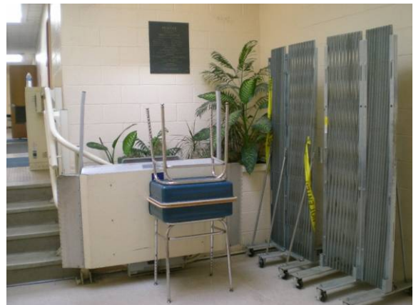
Photo #138: Stair lift to access 500 wing
