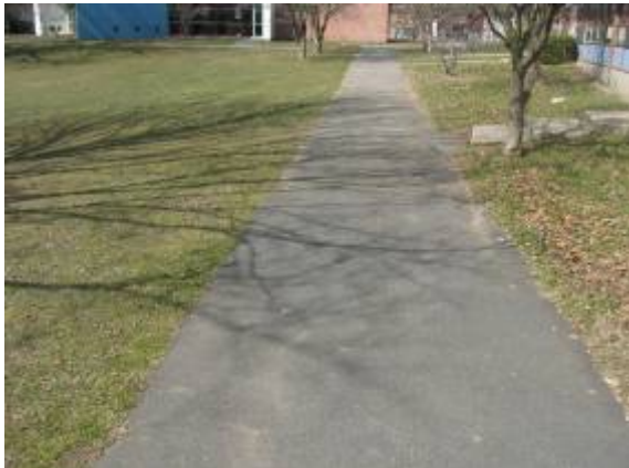
Photo #13: View of asphalt paved sidewalks.
