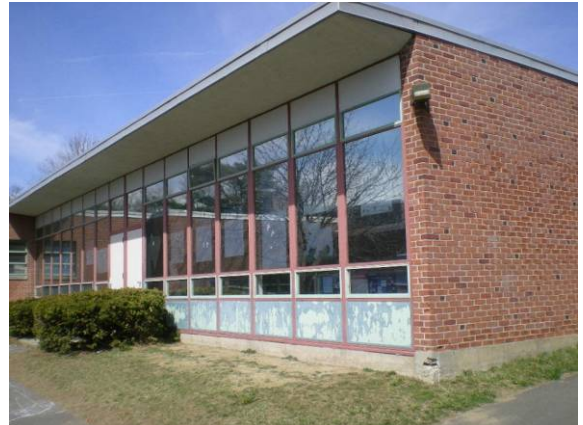
Photo #76: South elevation of 500 wing addition
