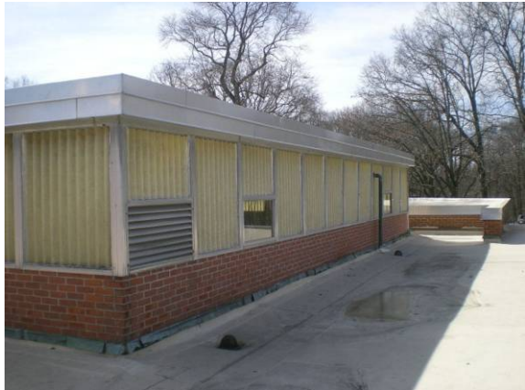
Photo #82: Clerestory section of gym
