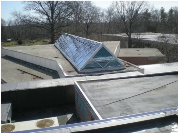
Photo #87: Roof over Media Center
