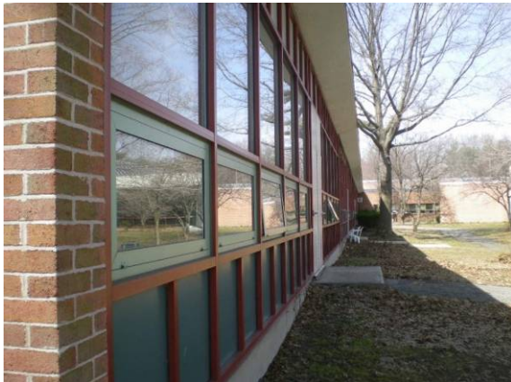
Photo #71: North side of 200 wing
