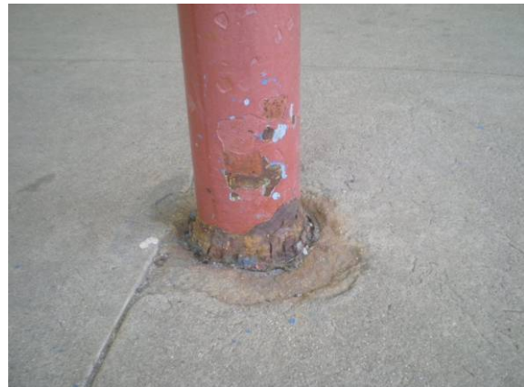
Photo #94: Typical condition of column base at main entrance
