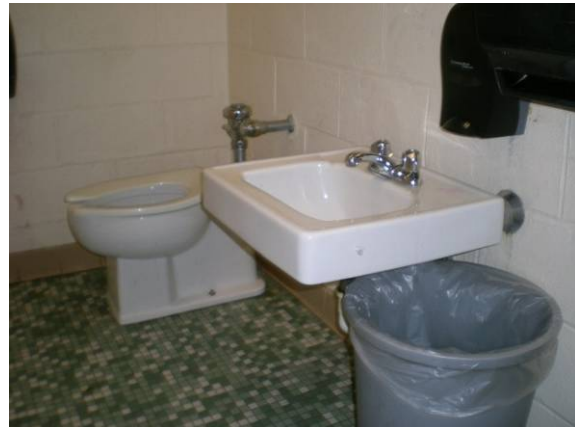
Photo #120: Restroom across from gym
