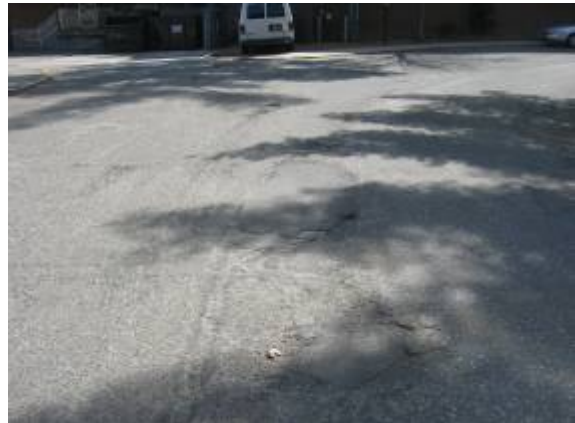
Photo #2: View of asphalt paved entry driveway.
