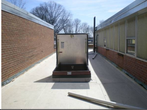
Photo #80: Roof hatch
