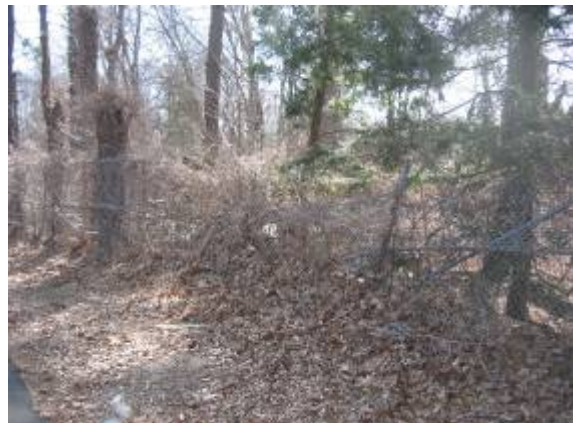
Photo #18: View of deteriorated chain link fencing.
