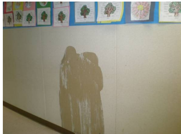
Photo #126: Vinyl wall covering in south modular wing
