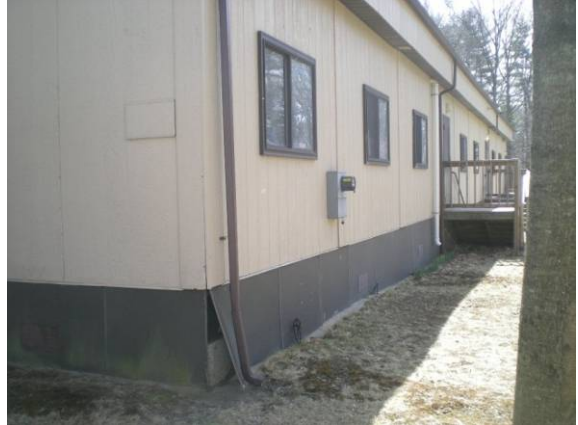
Photo #68: Modular addition
