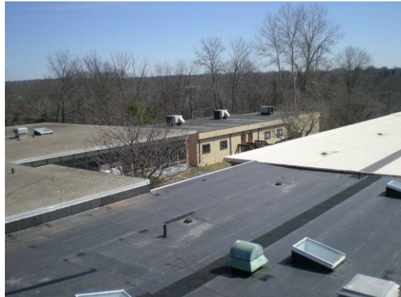
Photo #88: Roof overview looking towards 500 wing and north end modular wing
