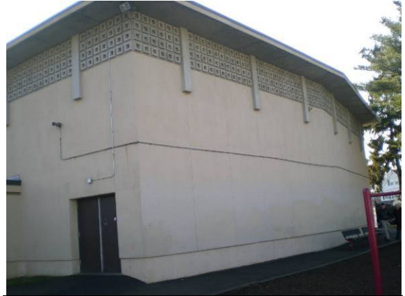
Photo #8: West elevation of gymnasium
