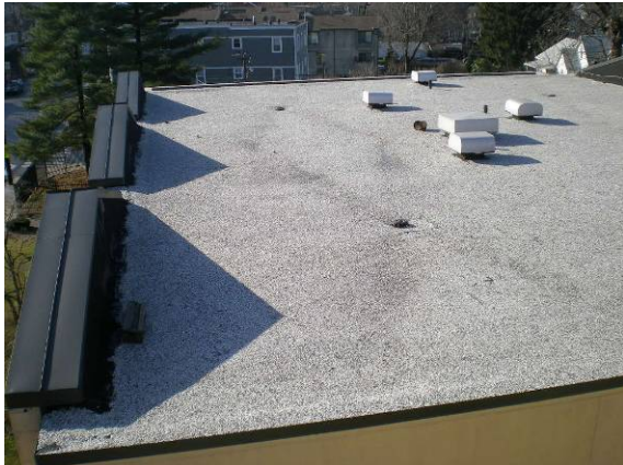
Photo #33: Roof over south wing
