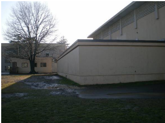
Photo #9: North elevation of gymnasium
