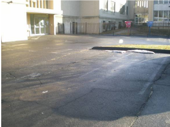
Photo #19: Potential for ADA entrance from south lot
