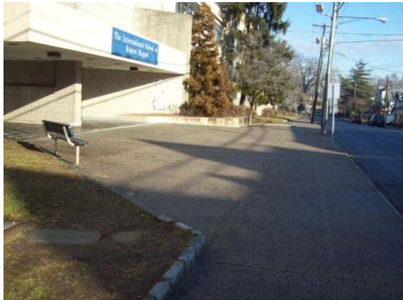
Photo #40: Pedestrian pavement near Lockwood Avenue entrance
