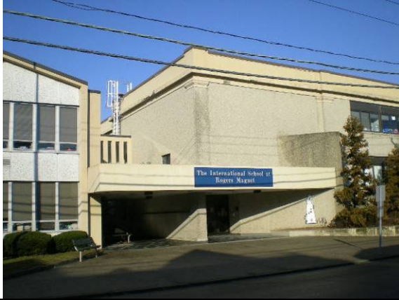
Photo #1: Main entrance off Lockwood Avenue
