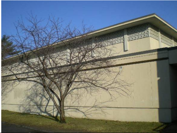
Photo #7: South elevation of gymnasium
