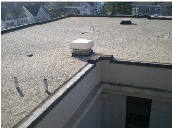
Photo #29: Middle section of school roofing
