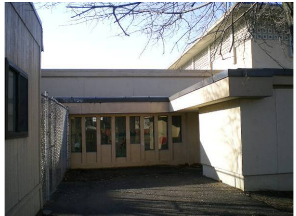
Photo #10: Elevation of corridor on north side
