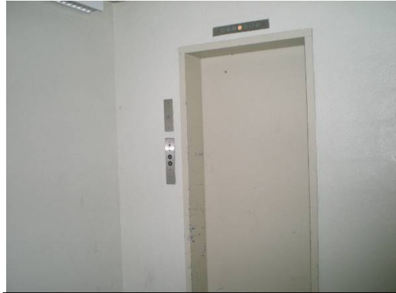
Photo #62: Elevator without Braille on jams
