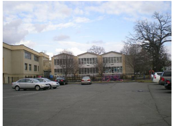
Photo #4: West elevation of south wing
