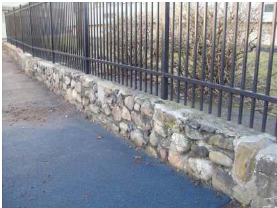
Photo #47: Retaining wall and fencing
