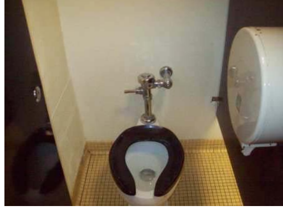
Photo #114: Typical toilet plumbing fixture
