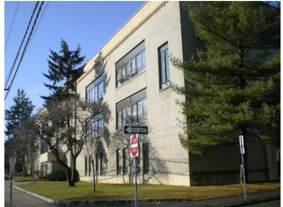
Photo #16: Partial front elevation along Lockwood – right section
