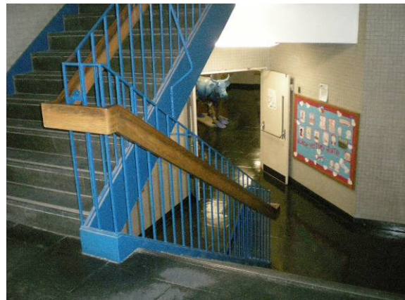
Photo #54: Split level main entrance – looking down to main office level
