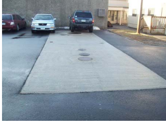
Photo #88: Underground storage tank location
