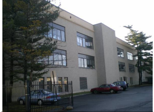
Photo #14: West elevation of north wing
