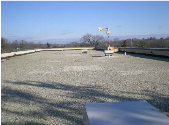
Photo #27: Roof over north wing
