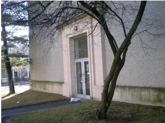
Photo #15: North elevation of north wing
