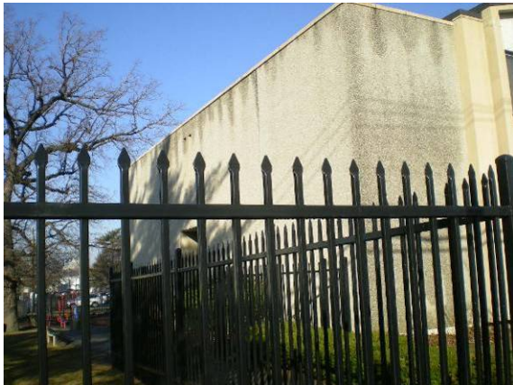
Photo #3: Left side elevation of south wing
