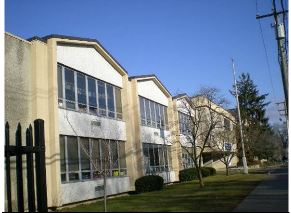
Photo #2: Partial front elevation off Lockwood – left end
