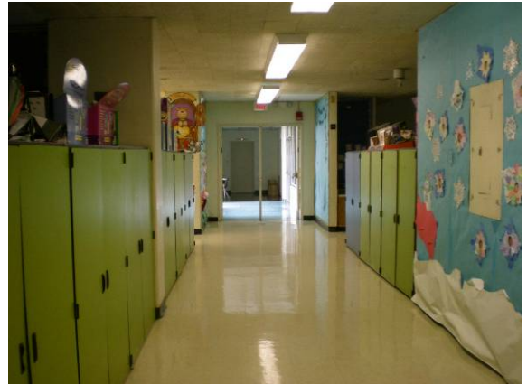
Photo #70: Open corridor in south wing
