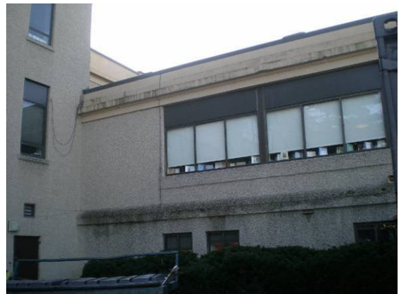
Photo #12: Upper partial north facing elevation
