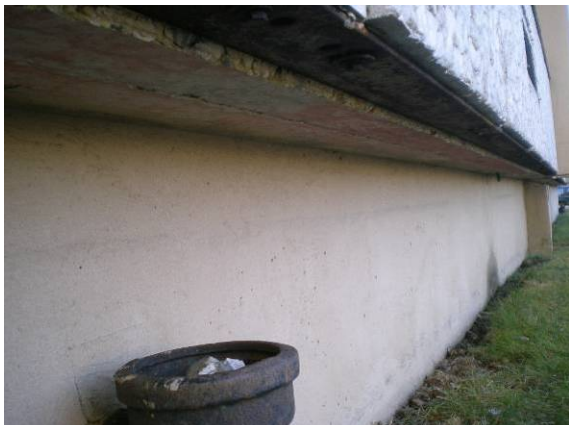
Photo #17: Underside detail south wing – steel angle supporting exposed aggregate panels
