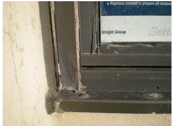
Photo #6: Condition of window sealant and gasket
