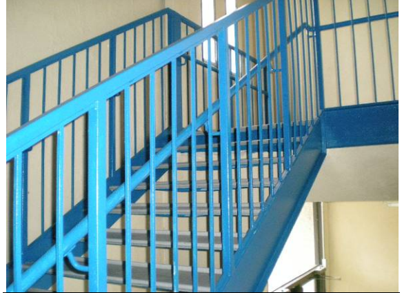
Photo #68: Open riser stair
