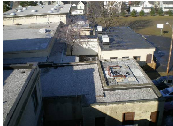
Photo #28: Various roofs looking towards gymnasium, including modular roofing
