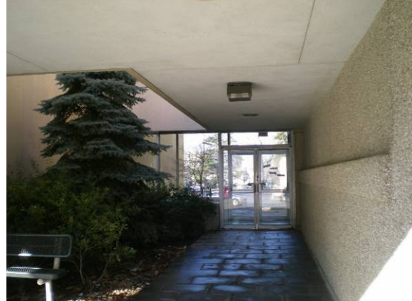
Photo #26: Side entrance into connector between main entrance and south wing
