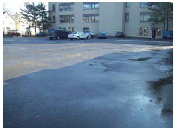
Photo #36: North parking lot
