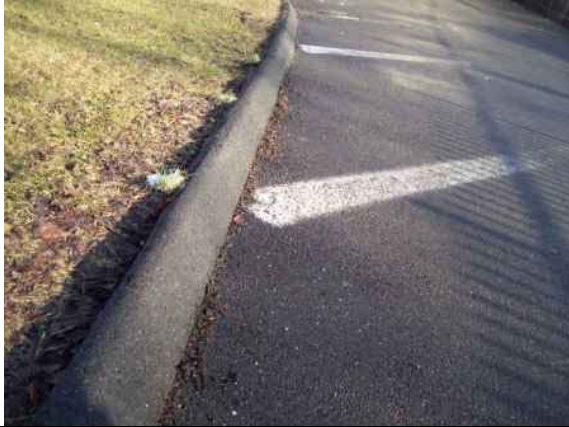
Photo #37: Extruded asphalt curbs
