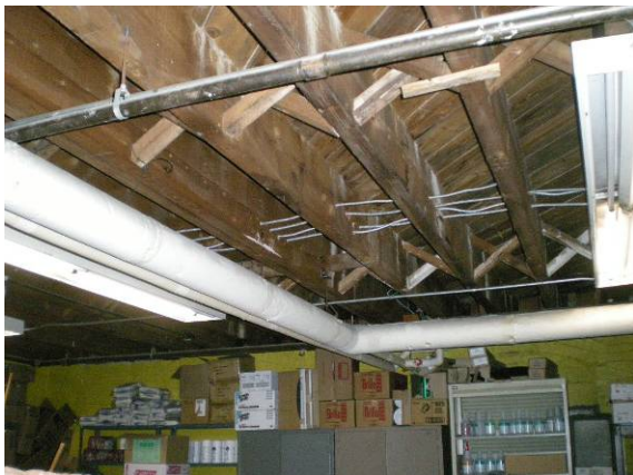
Photo #77: Floor structure in north wing
