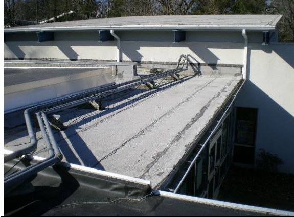
Photo #14: Built up roofing over Media Center
