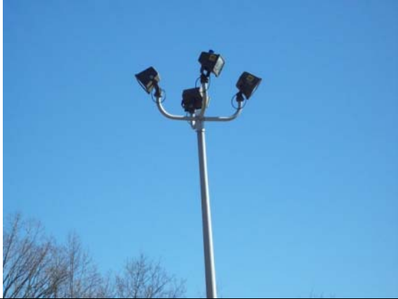
Photo #43: Site lighting
