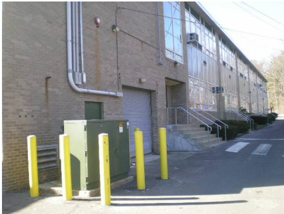
Photo #3: East elevation
