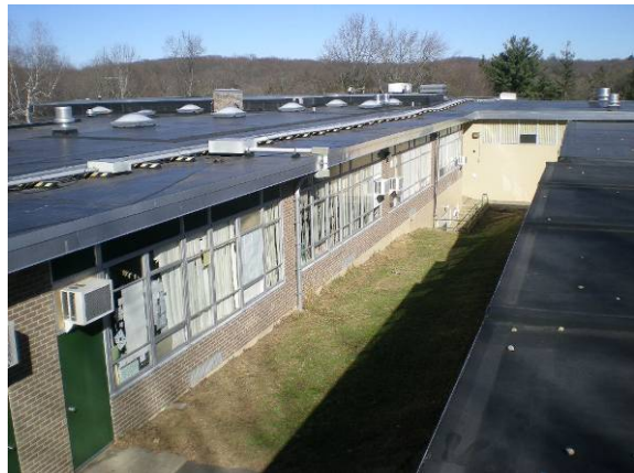
Photo #6: South elevation of classrooms at original school building
