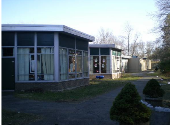
Photo #8: West elevation
