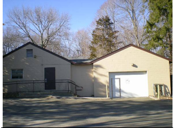
Photo #122: Garage attached to Annex building
