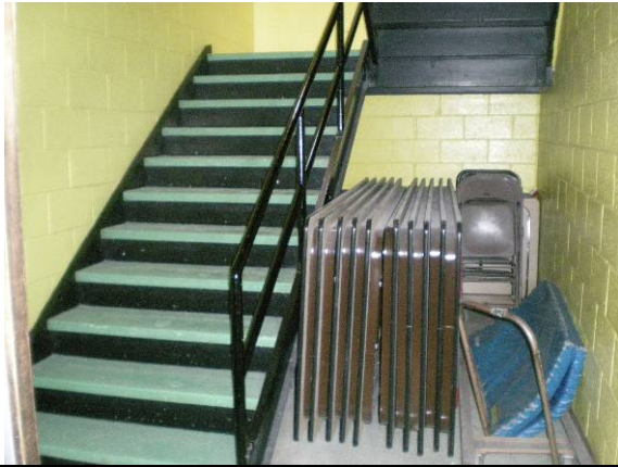
Photo #73: Storage under stairwell
