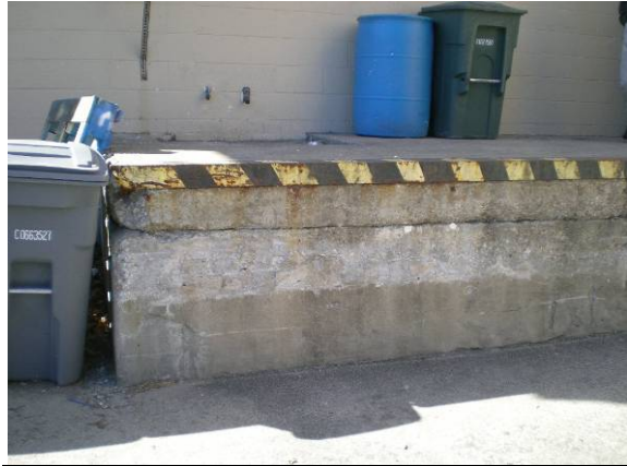
Photo #26: Loading dock conditions
