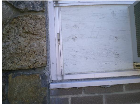
Photo #22: Sealant condition
