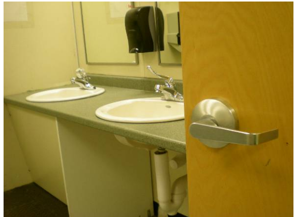
Photo #70: Restroom in modular wing
