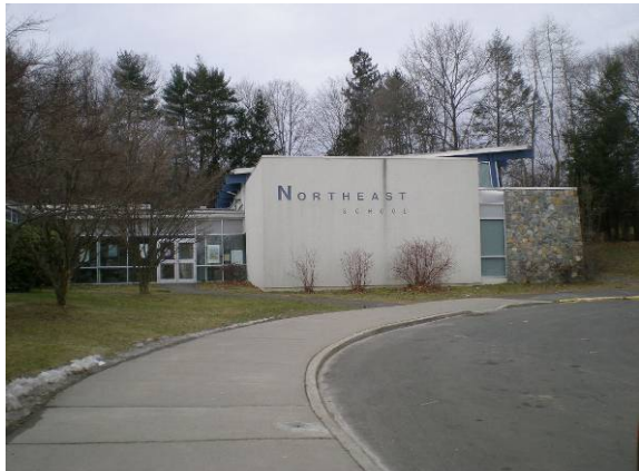
Photo #12: Front/east elevation of Media Center and only handicapped route
