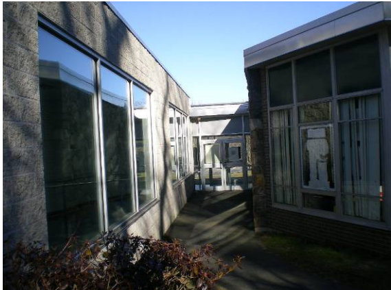
Photo #9: Junction between original school and Media Center
