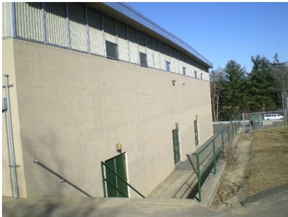
Photo #5: Rear/south elevation of gymnasium
