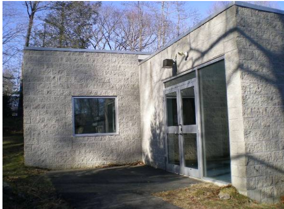
Photo #10: Rear/west elevation of Media Center
