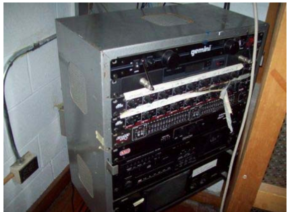
Photo #108: Sound system controls for auditorium
