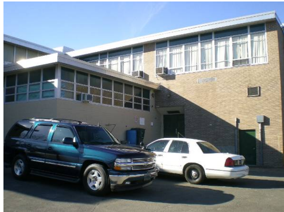
Photo #4: Southeast corner – loading dock area
