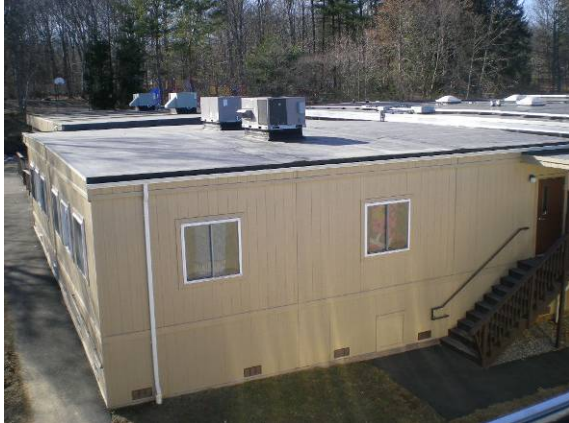
Photo #7: Modular classroom addition on south end of building
