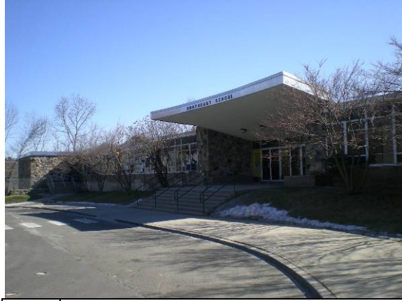
Photo #2: Front elevation and main entrance
