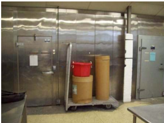
Photo #119: Walk in refrigerator and freezer
