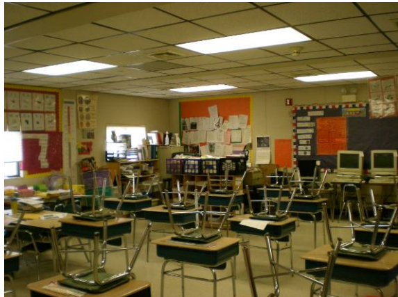
Photo #69: Classroom in modular wing
