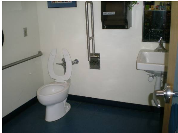
Photo #64: Media Center ADA unisex restroom
