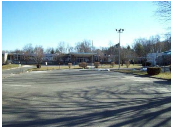
Photo #28: Main parking lot
