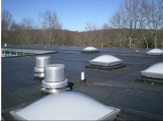
Photo #13: Roof overview of original school building
