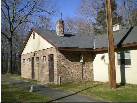
Photo #121: Annex building – west elevation
