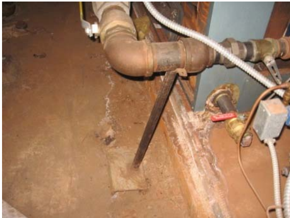
Photo #131: Leaning metal support post at gas piping to boiler
