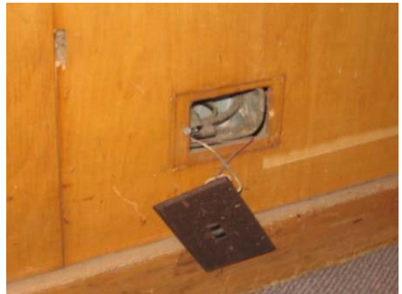
Photo #156: Loose and exposed wiring at receptacle outlet at Auditorium
