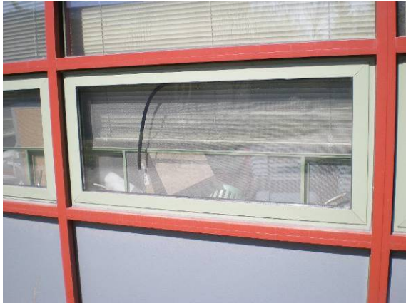
Photo #21: Loose window gasket
