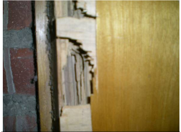
Photo #56: Evidence of termite damage in auditorium near access panel
