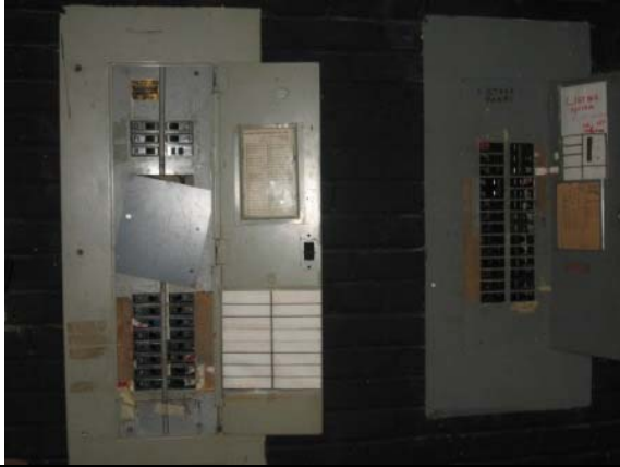
Photo #151: Original and worn circuit break panels at stage
