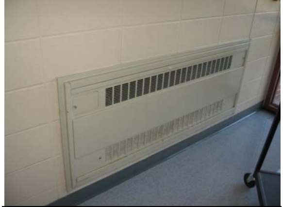
Photo #134: Replacement in-wall mounted radiant heat unit at end of corridor
