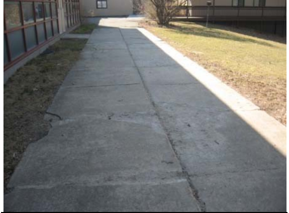
Photo #98: Deterioration and spalling of concrete sidewalk at left side of building
