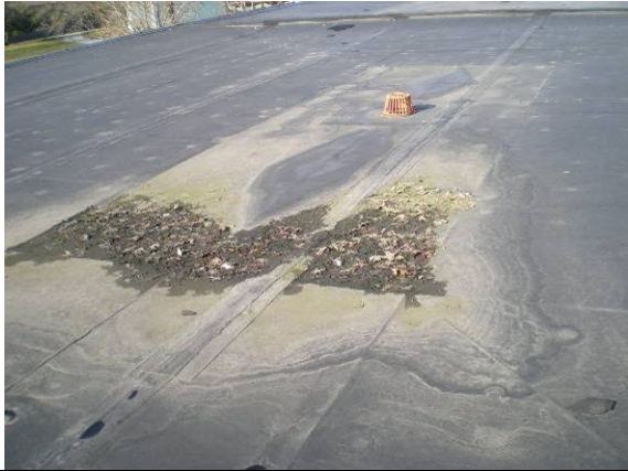
Photo #31: Evidence of ponding and area requiring resloping to existing drainage device
