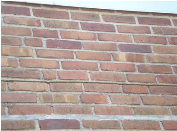
Photo #23: Damaged mortar and shifting of brick veneer at rear off of main office area
