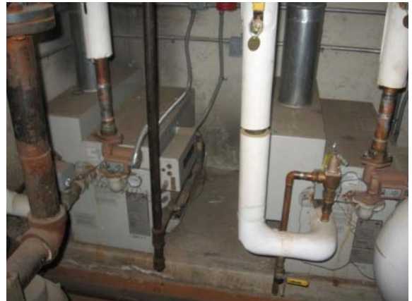
Photo #138: Domestic water boilers
