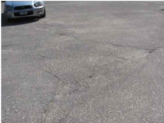
Photo #89: Cracking and worn asphalt paving at main parking lot
