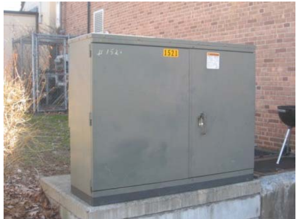
Photo #148: Pad-mounted transformer
