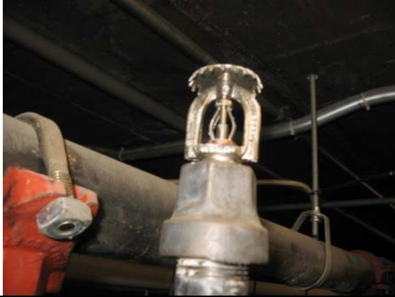
Photo #163: Central sprinkler head installed in fire suppression system at basement
