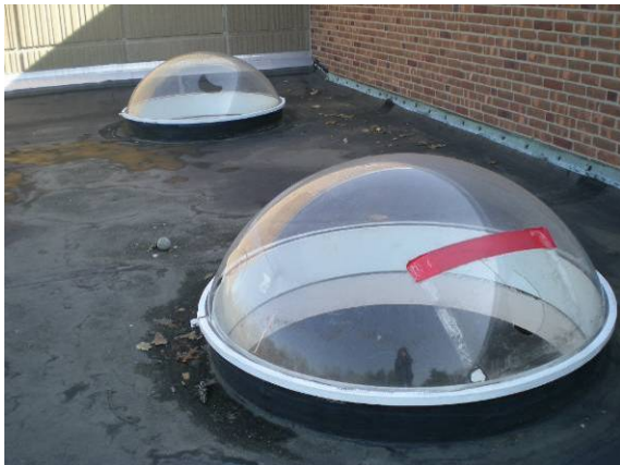
Photo #39: Broken/damaged skylights at main covered walkway
