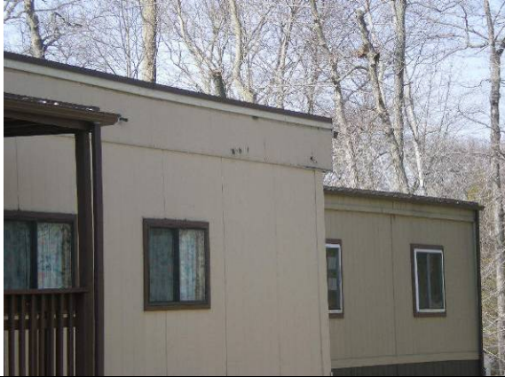
Photo #19: East side of modular – evidence of active nesting and wood damaging birds
