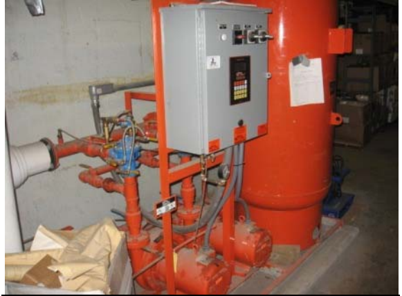
Photo #146: Unused domestic water booster system
