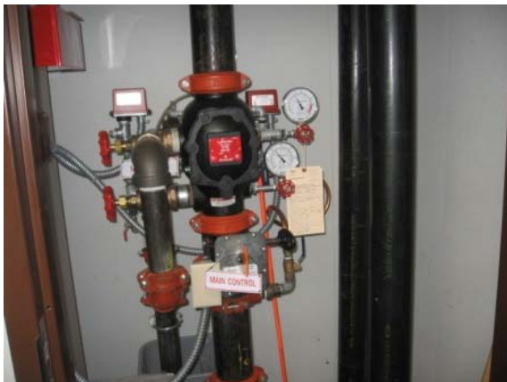
Photo #161: Dry-pipe riser at modular building
