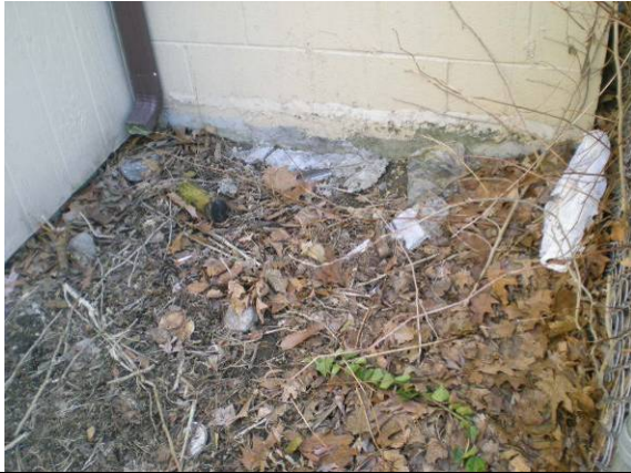
Photo #79: Area above efflorescence in basement – evidence of ponding – near transformer
