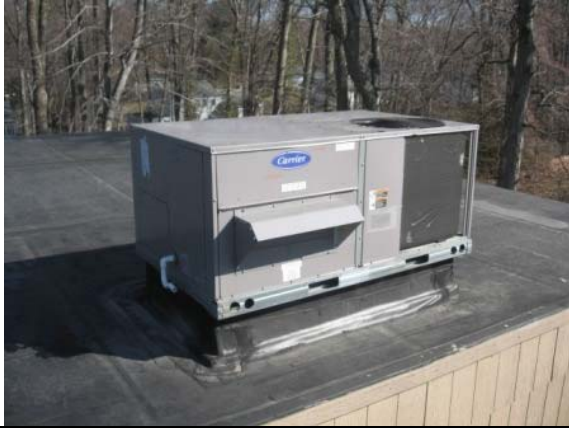
Photo #127: Rooftop package unit (RTU) for modular classrooms
