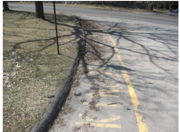
Photo #90: Caved in section at exit asphalt drive lane
