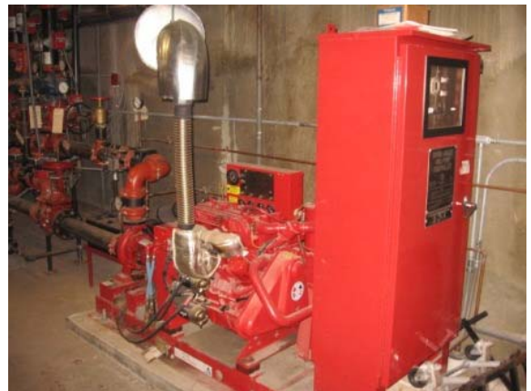
Photo #162: Fire suppression fire pump and controller at basement
