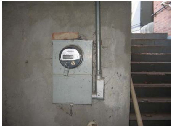
Photo #150: Main electric meter at exterior stairs adjacent to basement
