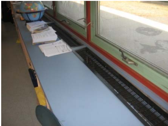
Photo #135: Perimeter radiant heat unit at classroom
