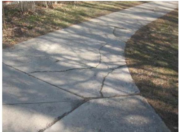
Photo #100: Settlement and cracking at concrete sidewalk at right side of building
