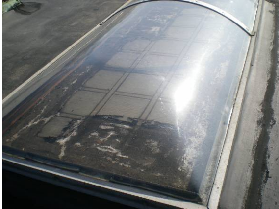
Photo #37: Mastic covered skylight glass blocks
