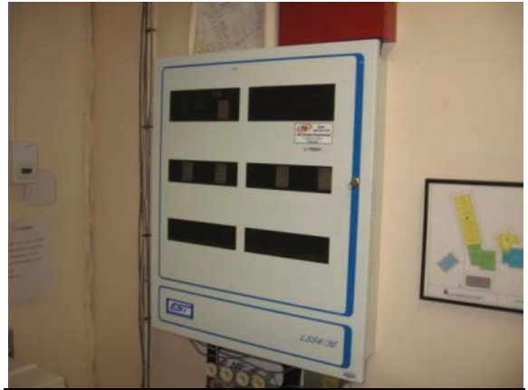
Photo #158: Central fire alarm panel at office
