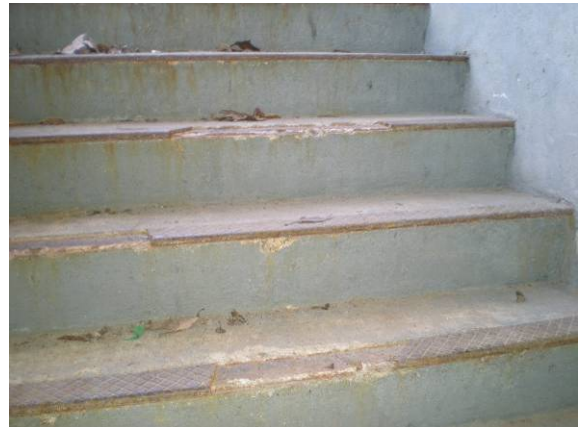
Photo #60: Stair to basement missing steel tread nosings
