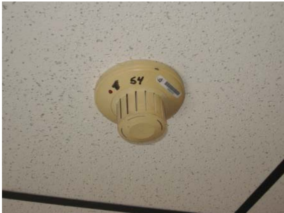
Photo #167: Smoke detector at common area
