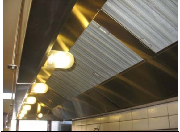
Photo #164: Kitchen exhaust hood without fire suppression system
