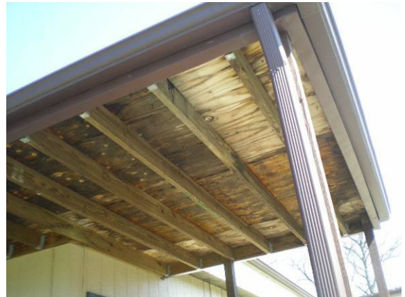
Photo #18: Water stained covered walkway of modular wing
