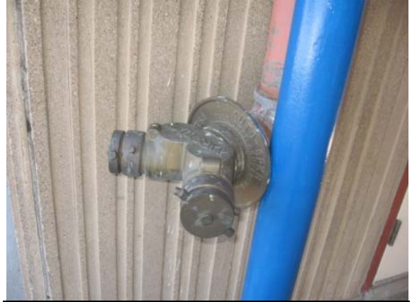
Photo #170: Siamese hose connector at front of building
