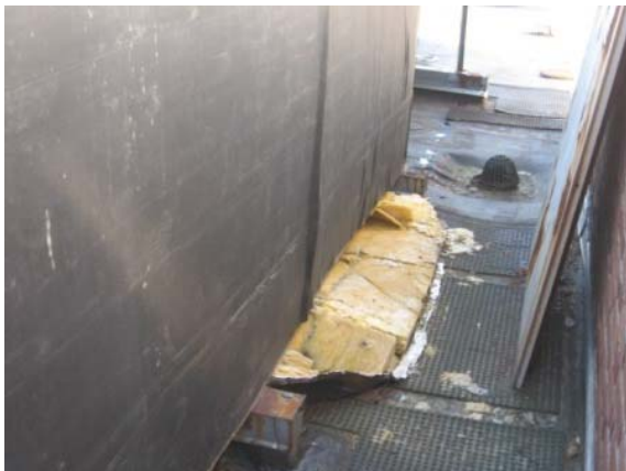
Photo #125: Deterioration at HVAC rooftop ducting
