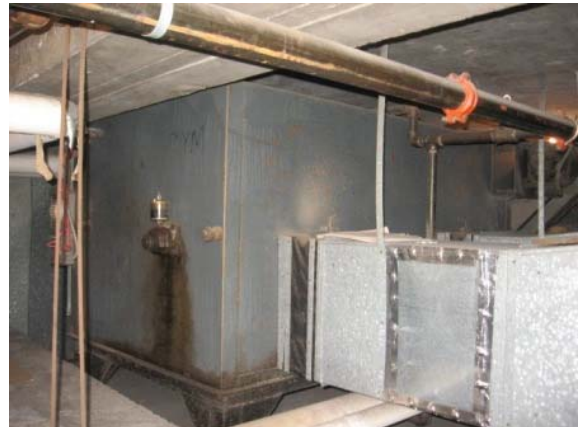
Photo #132: HV-2 High-capacity AHU for Gymnasium/Cafeteria
