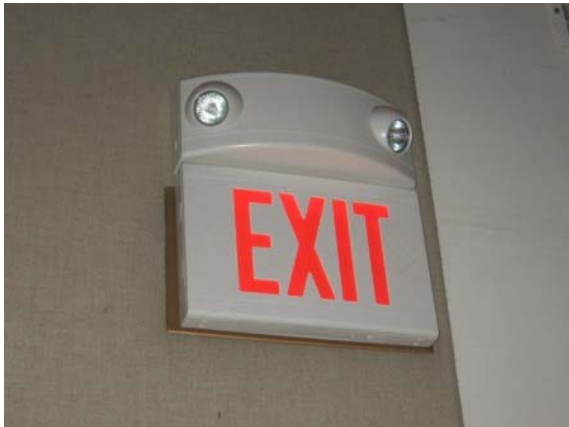
Photo #171: Combination emergency lights/illuminated exit sign
