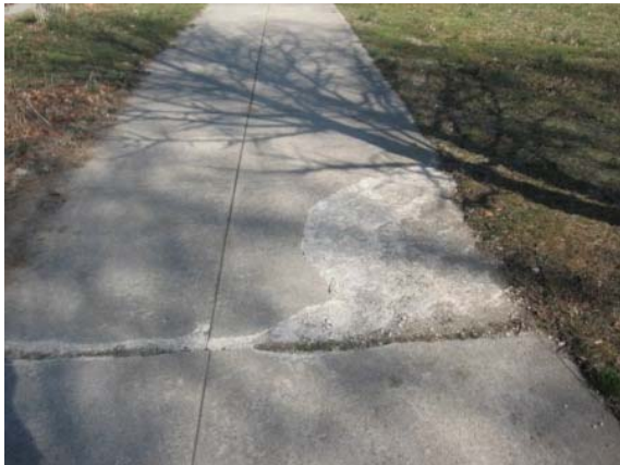
Photo #99: Deterioration and spalling of concrete sidewalk at rear of building
