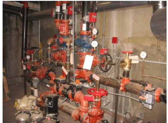
Photo #160: Main fire suppression system at basement
