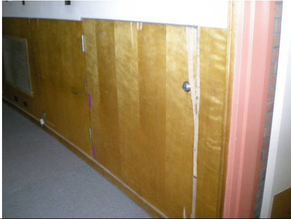
Photo #55: Evidence of termite damage at access panel at rear of auditorium
