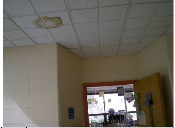
Photo #74: Evidence of roof leaks in corridor
