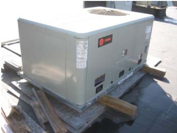
Photo #129: Replacement RTU for older rooftop package unit
