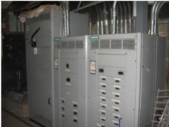
Photo #149: Main electrical switchgear in basement of building
