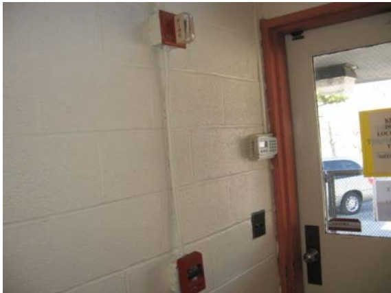
Photo #165: Fire pull station, strobe alarm and building security code pad
