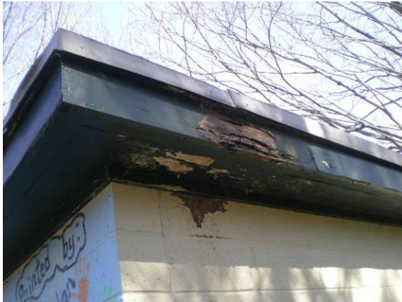
Photo #63: Damaged fascia and soffit of storage building
