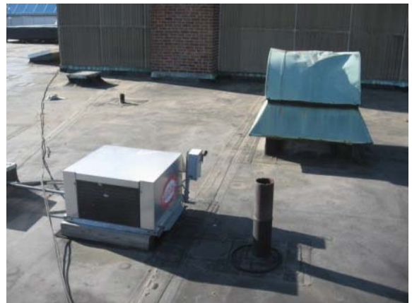
Photo #180: Rooftop refrigeration unit and exhaust hood
