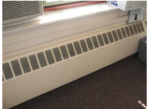
Photo #136: Perimeter baseboard radiant heat unit at office
