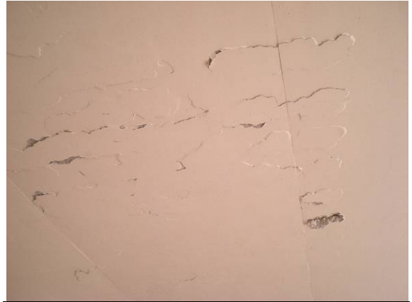
Photo #80: Spalling under main walkway canopy
