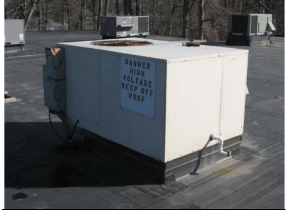
Photo #128: Older rooftop package unit (RTU) for modular classrooms
