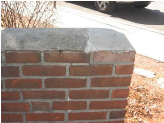
Photo #105: Deterioration at brick retaining wall adjacent to loading dock
