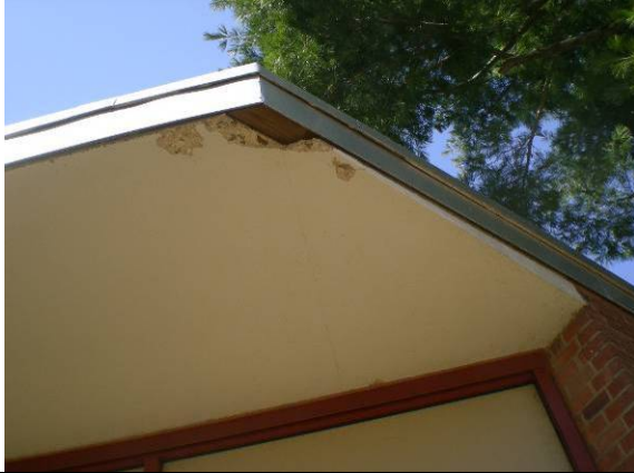
Photo #25: Spalling soffit near kindergarten classrooms
