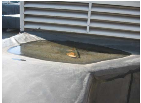
Photo #124: Ponding at HVAC rooftop ducting
