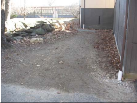
Photo #97: Worn landscaping path rear of modular building (install asphalt sidewalk)
