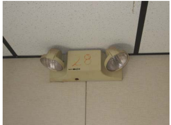
Photo #168: Emergency backup lights at common area
