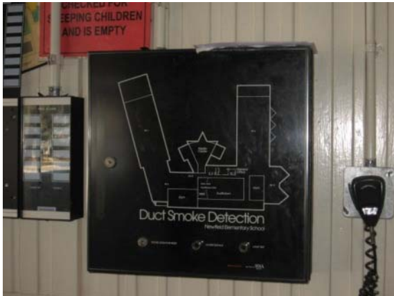
Photo #159: Annunciator panel at entrance vestibule
