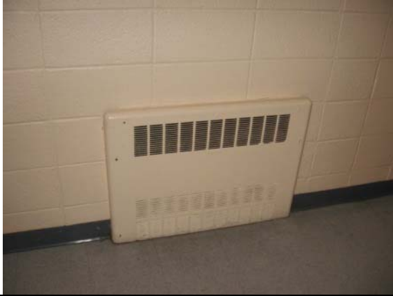
Photo #133: In-wall mounted radiant heat unit at corridor
