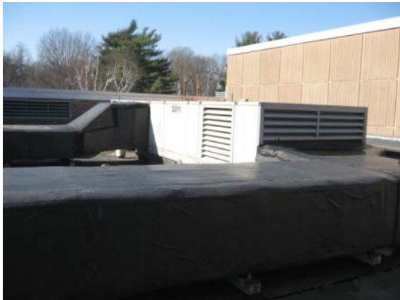
Photo #123: Rooftop package unit (RTU), for media center, with rubber covering HVAC ducting
