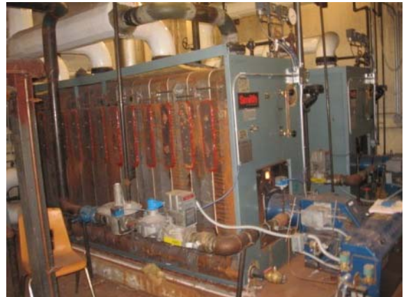
Photo #130: Heating boilers (one with side jackets off the boiler)
