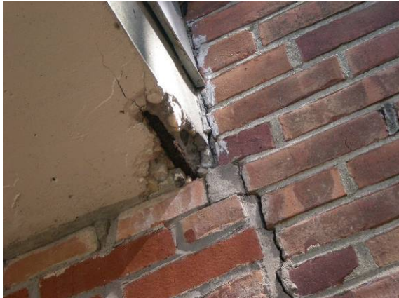
Photo #27: Cracking brick and exposed rebar at front canopy at kindergarten area
