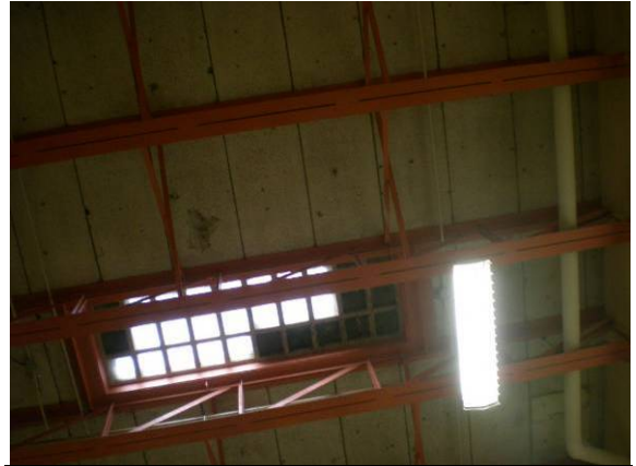
Photo #68: Covered glass block and damaged tectum panels at ceiling of gymnasium/cafeteria
