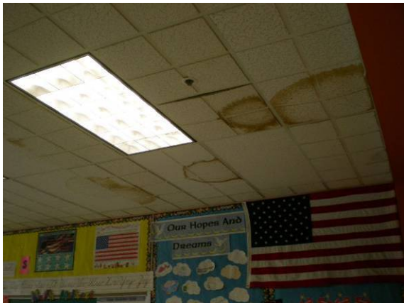
Photo #75: Ceiling staining in Classroom 316
