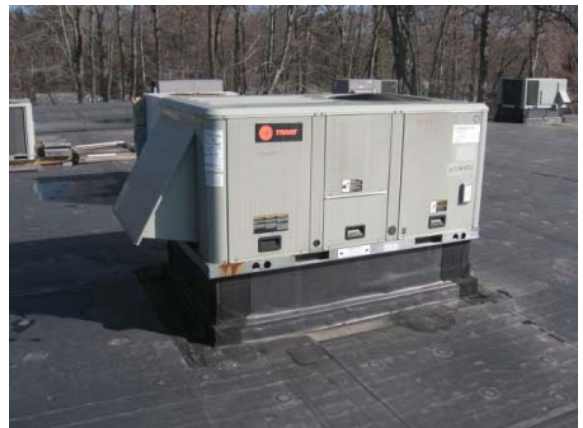
Photo #126: Rooftop package unit (RTU) for modular classrooms
