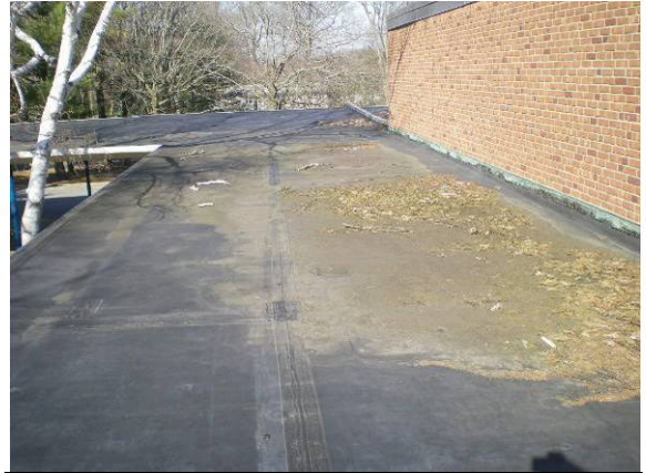
Photo #38: No drainage devices on north side of courtyard roof
