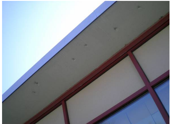
Photo #24: Damaged soffit
