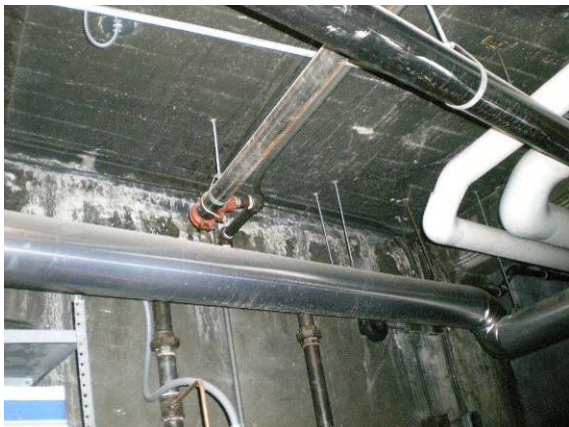
Photo #71: Efflorescence in basement under downspout in corner near transformer
