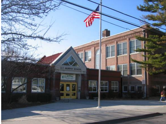
Photo #1: View of the front façade and main office lobby entrance
