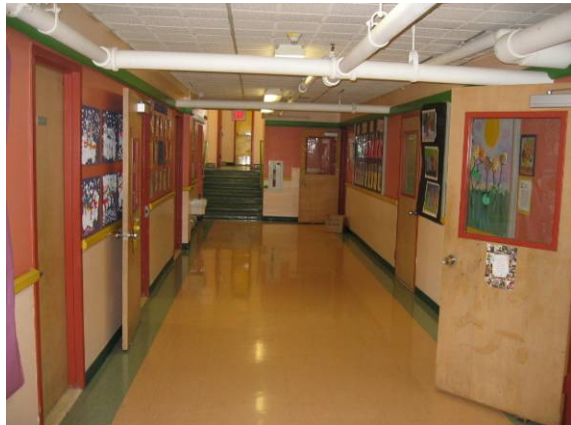
Photo #51: View of a typical common interior corridor
