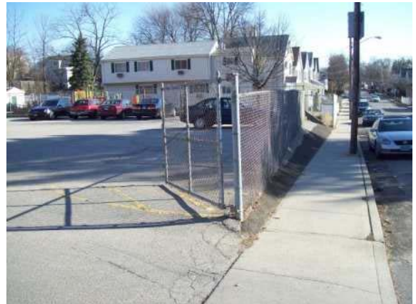
Photo #142: Perimeter fence at parking lot
