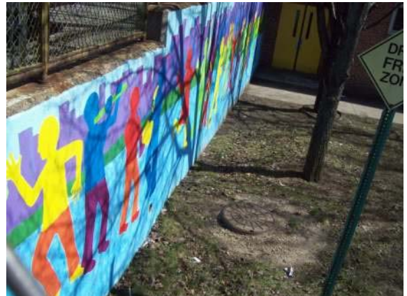
Photo #136: Concrete retaining wall at west side of building
