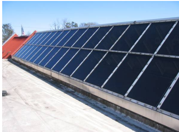
Photo #28: View of the pitched skylight system over the media center
