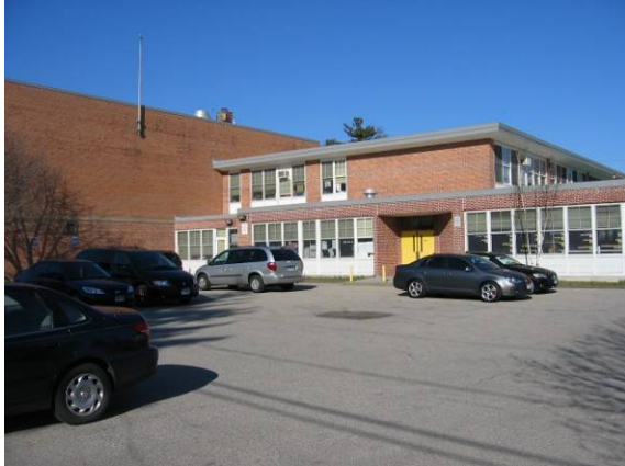
Photo #19: View of the rear façade of the kindergarten, first grade and gym
