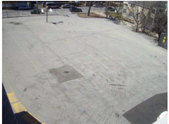
Photo #124: Northwest paved area
