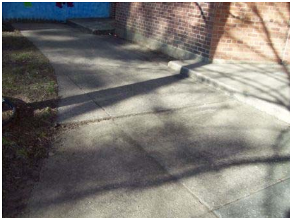
Photo #131: Concrete sidewalk
