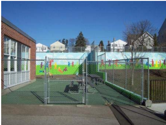
Photo #141: Typical site fencing
