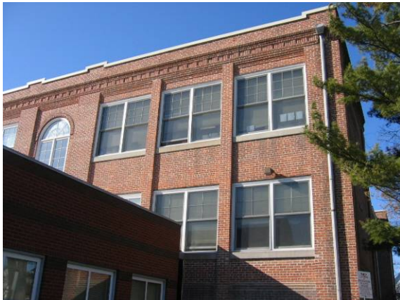
Photo #15: View of the south façade of the 3-story portion
