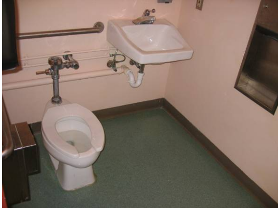
Photo #61: The single user toilet room within the nurse's office has one grab bar
