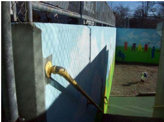
Photo #137: Concrete retaining wall near playground at south side of building
