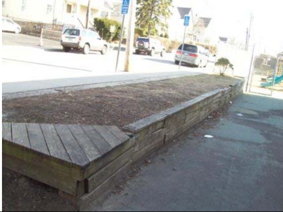
Photo #139: Wood timber retaining wall at east side of building
