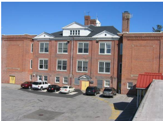
Photo #11: View of the rear façade facing the bus parking lot
