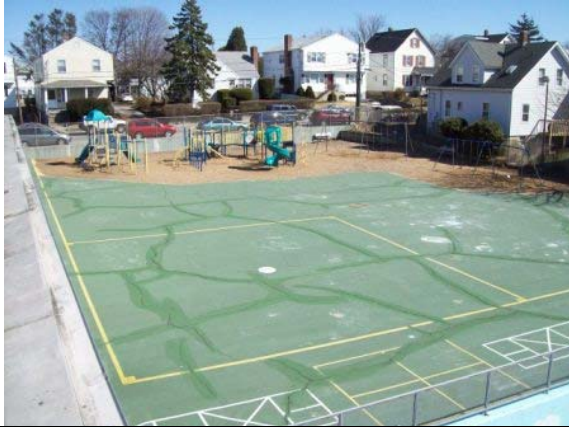
Photo #127: Paved area at playground
