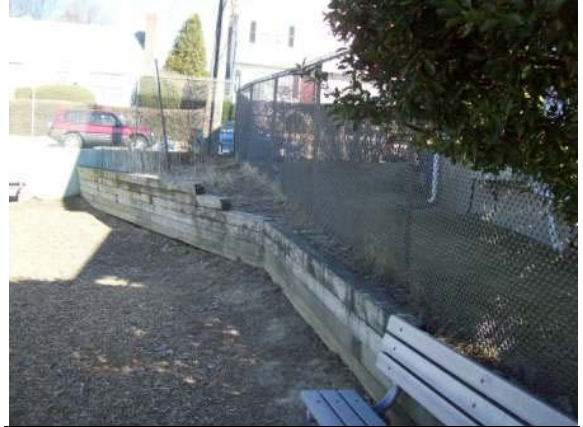
Photo #140: Wood timber retaining wall at southeast corner of property
