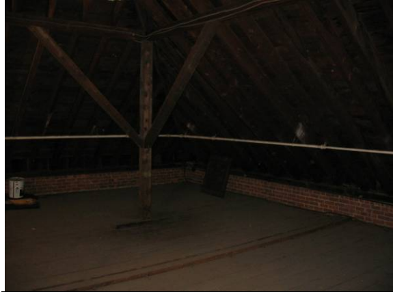
Photo #38: View of the pitched roof attic - no insulation exists
