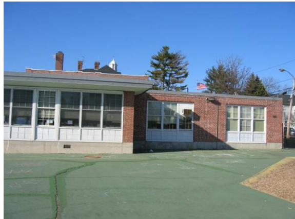
Photo #16: View of the south façade of the 1-story first grade wing
