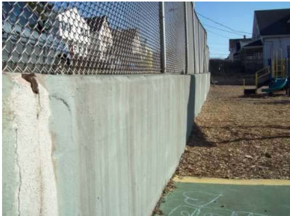
Photo #135: Concrete retaining wall along east property line
