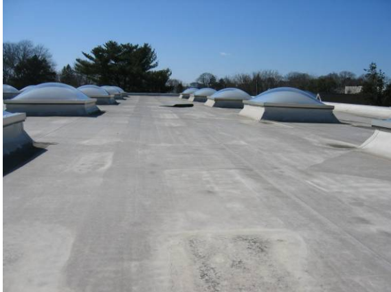
Photo #31: Overview of the flat white EPDM gymnasium roof
