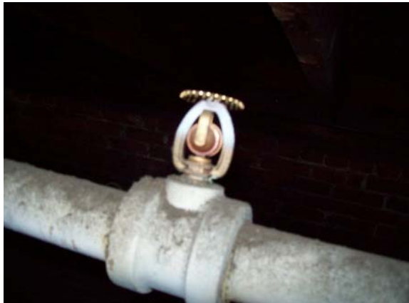
Photo #112: Dry-pipe sprinkler head in attic
