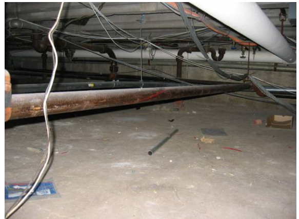
Photo #72: Limited portions of the school have crawl space type cellars
