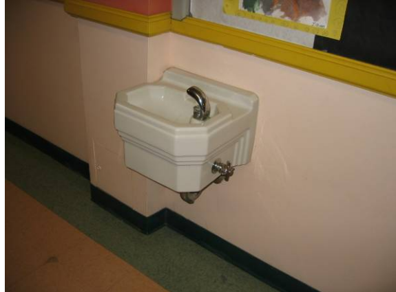
Photo #62: None of the corridor or gymnasium child water fountains are accessible
