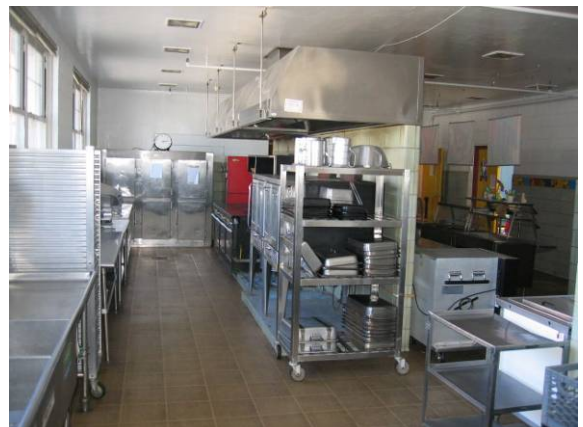
Photo #48: View of the cafeteria kitchen
