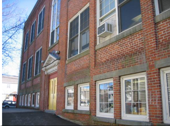
Photo #14: View of the north façade of the 3-story portion
