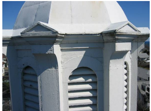
Photo #36: Detail view of the wood and painted metal bell tower - note the deteriorated wood work
