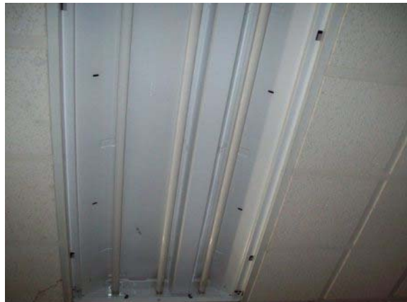
Photo #102: Typical fluorescent lighting ballast
