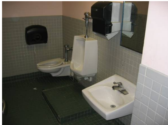
Photo #60: Second view of a typical toilet room with limited handicapped access
