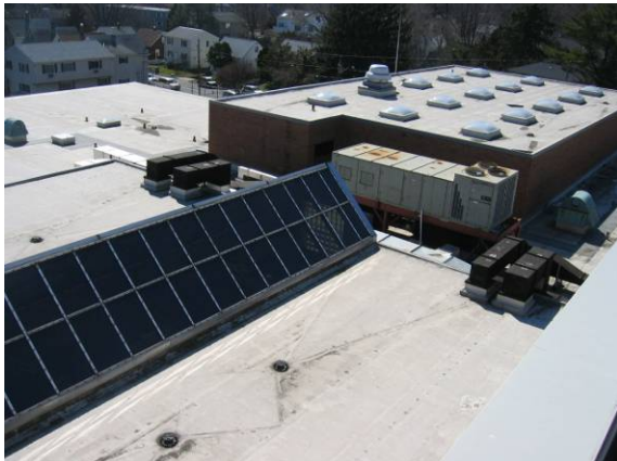
Photo #21: Overview of the flat white EPDM roofs towards the rear
