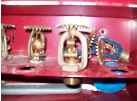
Photo #110: Wet pipe sprinkler head
