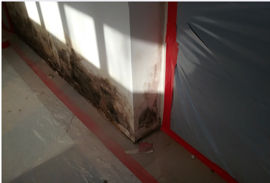
Wall covering was removed on the first floor to identify the location of the mold.
