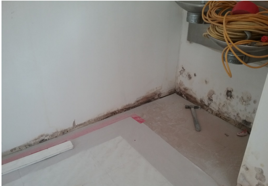
Wall covering was removed on the first floor to identify the location of the mold.
