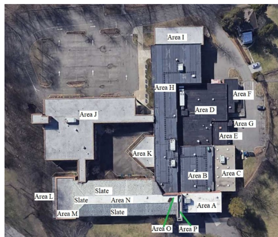
Roof with labeled roof areas
